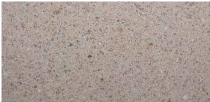
Image 18. Indicative example of Exposed Aggregate Concrete
