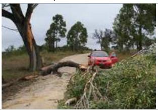
Debris, including fallen limbs, on carriageway causing an obstruction to more than 50% of the traffic lane.
