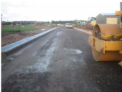
Rankin Street Construction
