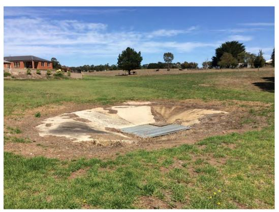
Photo 8 - Drainage inlet structure near intersection of Harris Rd and Scanlan Drive
