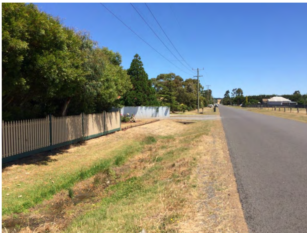
Photo 27 – Typical roadside channel in Sinclair Street South
