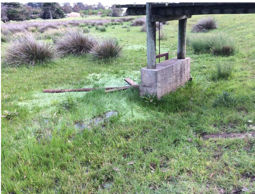
Photo 12 – Outlet structure within Irrewillipe Road retarding basin
