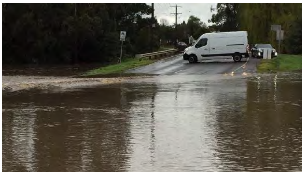
Figure 6.13 Flooding across Wallace Street
