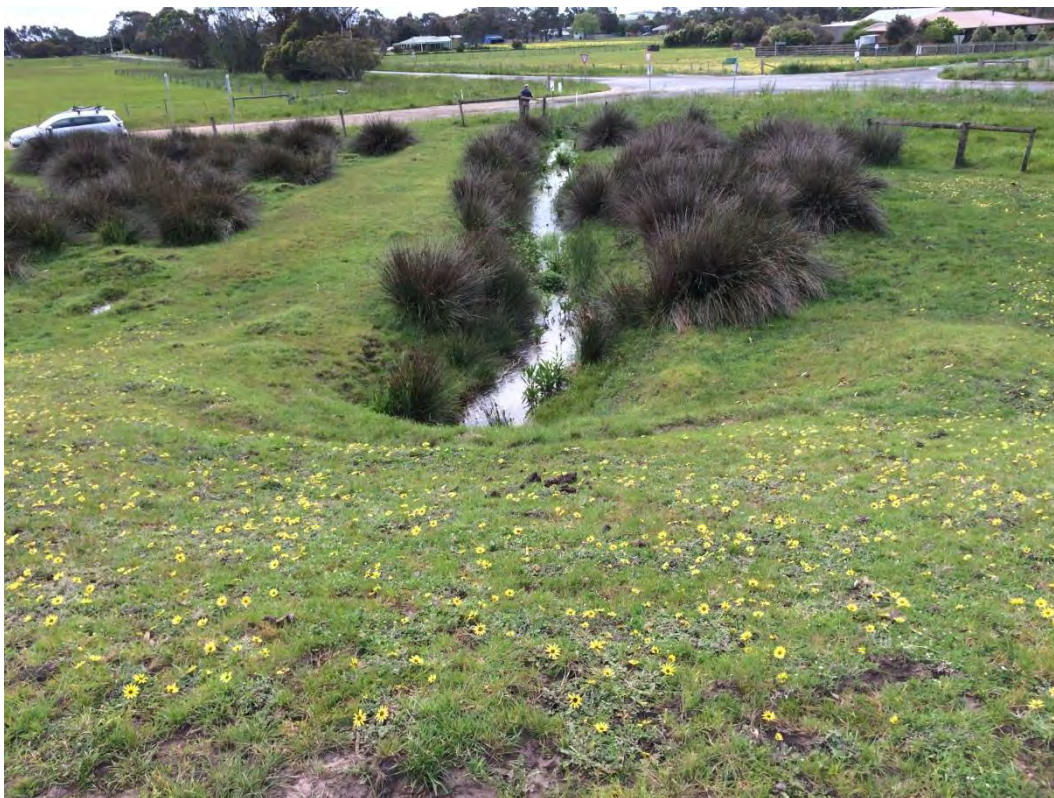
Photo 11 – Outlet from Irrewillipe Road retarding basin
