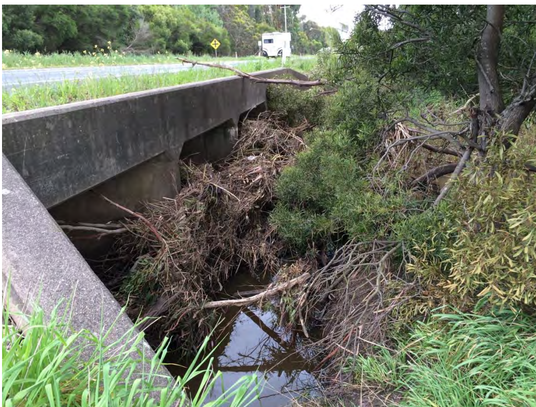
Photo 25 – Deans Creek at Princes Highway
