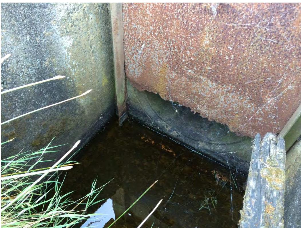
Photo 13 – Drainage outlet from Irrewillipe Road retaining basin
