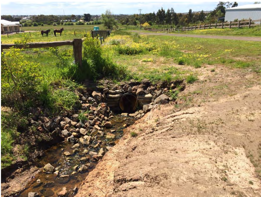
Photo 19 – Drainage along western side of Dowling Street
