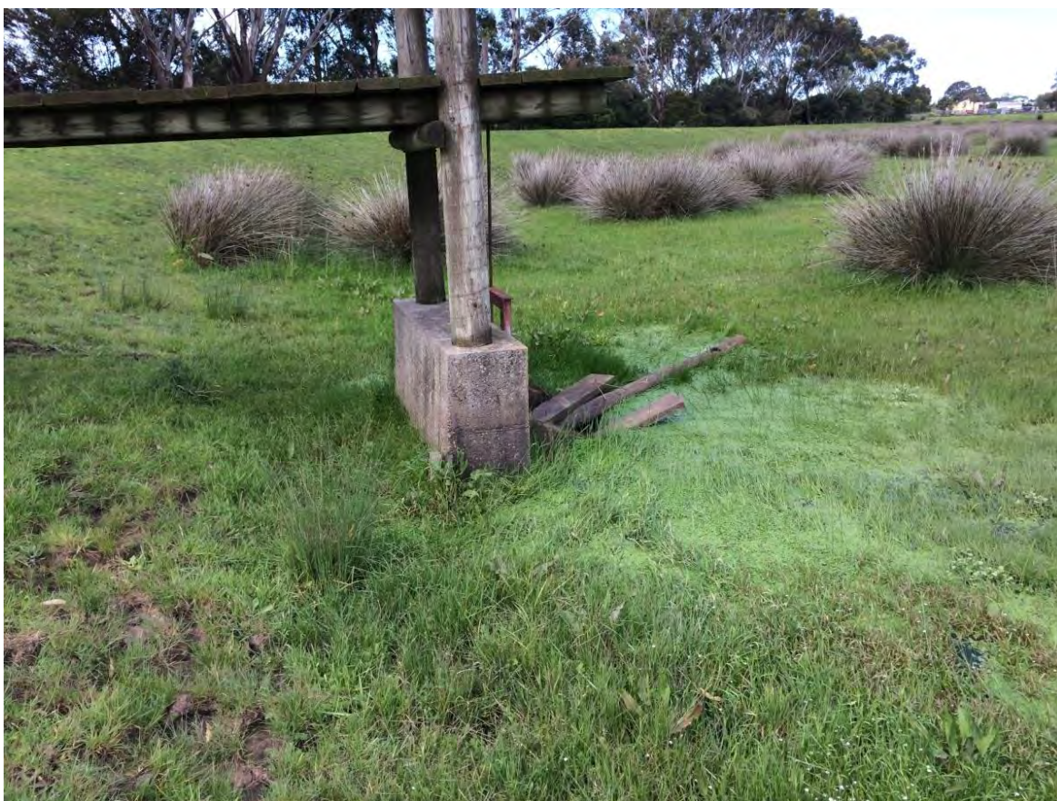
Figure 6.2 Irrewillipe Road Retarding basin outlet structure
