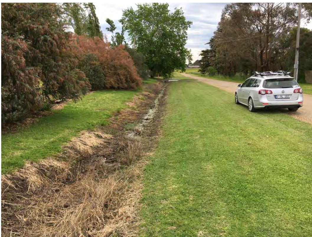
Photo 9 – Drainage swale alongside Ballagh Street
