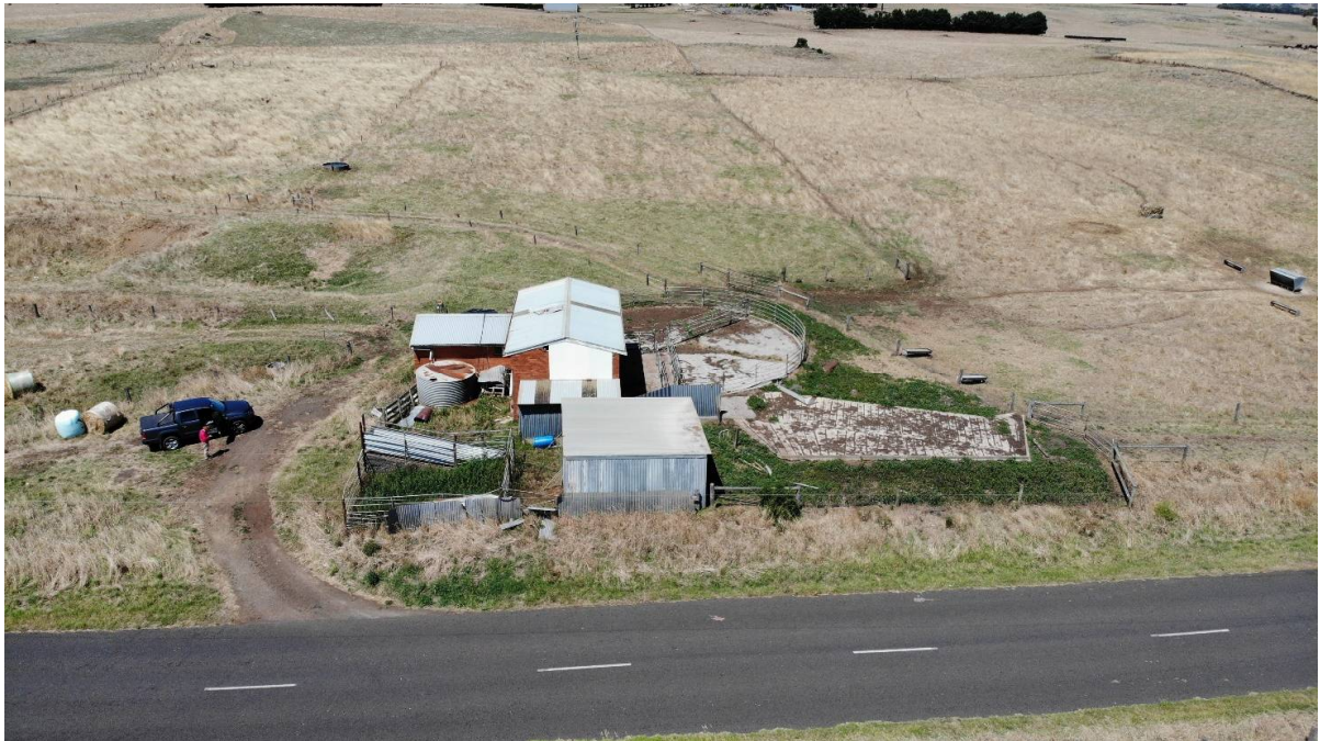
Images 7 & 8: Old dairy, yards, shed and loading yards on Nalingil Road.
