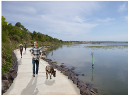
Visualisation of the proposed concrete path on a rock boulder revetment wall, Option B
