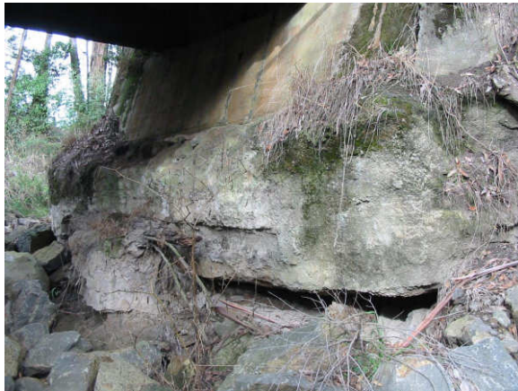
Undermining of Concrete Abutment
