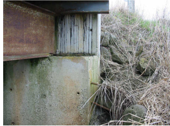
Missing Concrete Wingwall
