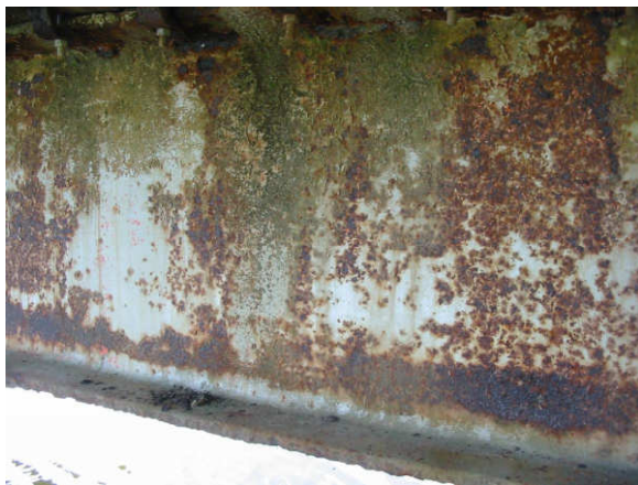
Corrosion of Steel Beams
