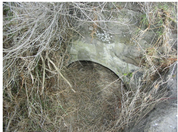
Blocked Culvert/Waterway
