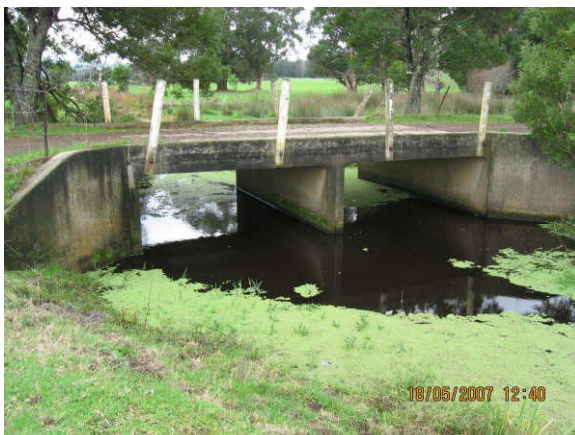
Major Drainage Structure (Box Culvert)
