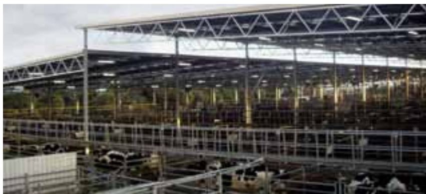
A new roof was constructed over the Colac Regional Saleyards facilities.
