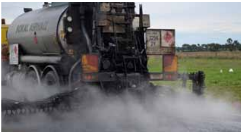
Resealing works at the Colac municipal aerodrome.
