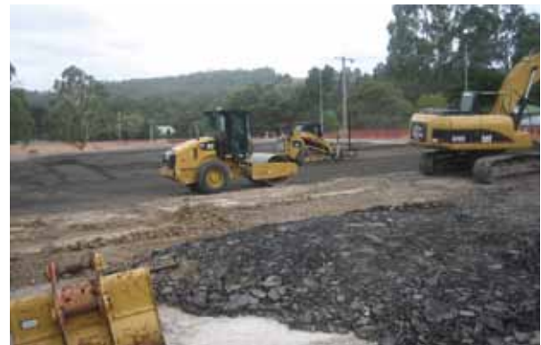
Above: Gellibrand netball courts under construction.
