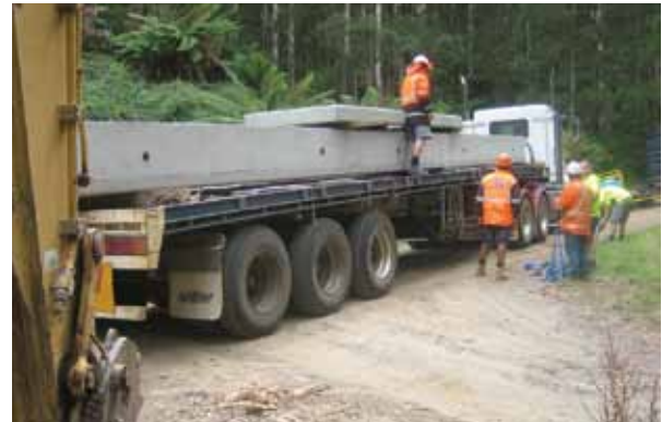
Above: Transporting Carlisle Valley Road bridge beam.
