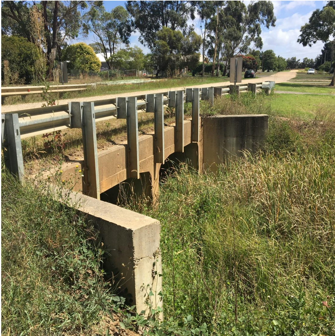
Appendix Figure A. 3: Box culverts crossing Sladen Street at Unnamed Tributary
