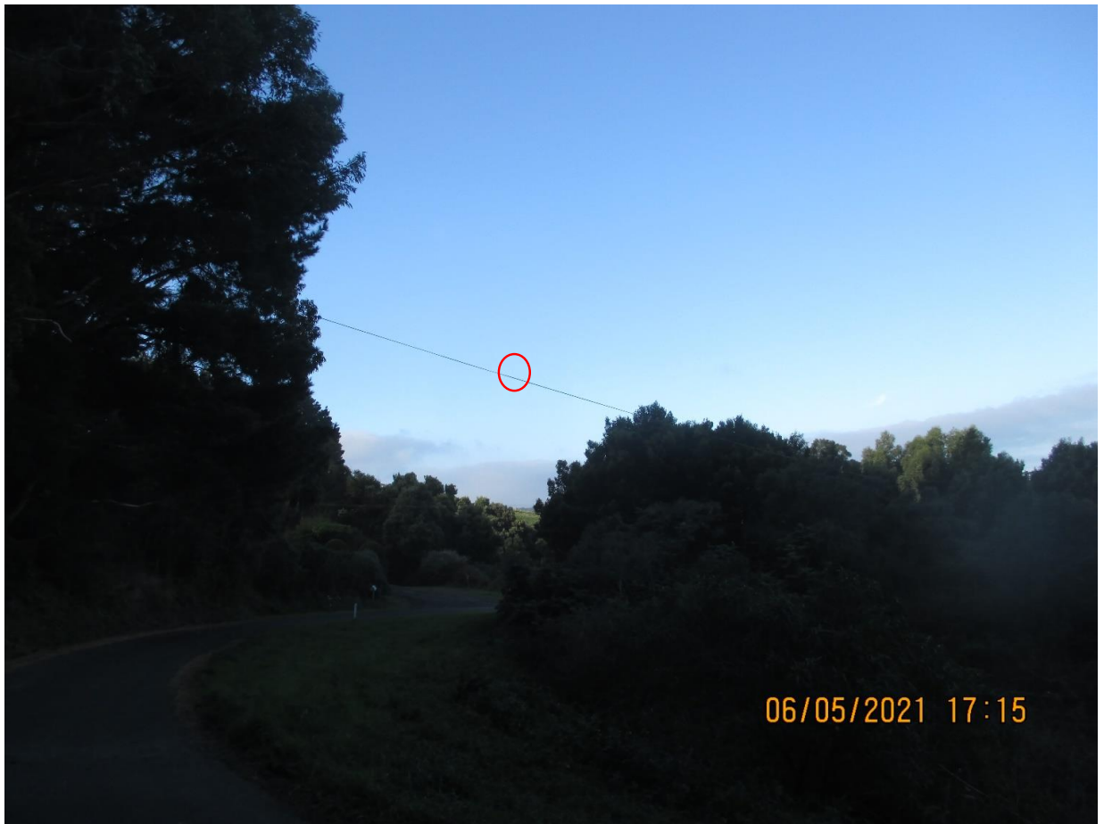
Coming down Sunnyside road adjacent to 290 Sunnyside
