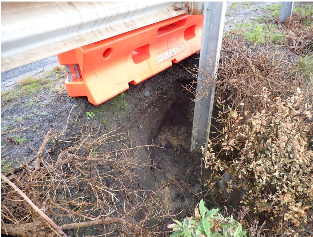
Photo 7 View of the western extent of the slide< the failed area has retrogressed under the barrier as far as the rear side of the barrier at the surface. The extent of the lower cavity extends a further approximately 200 mm beyond the rear of the barrier when viewed in plan.
