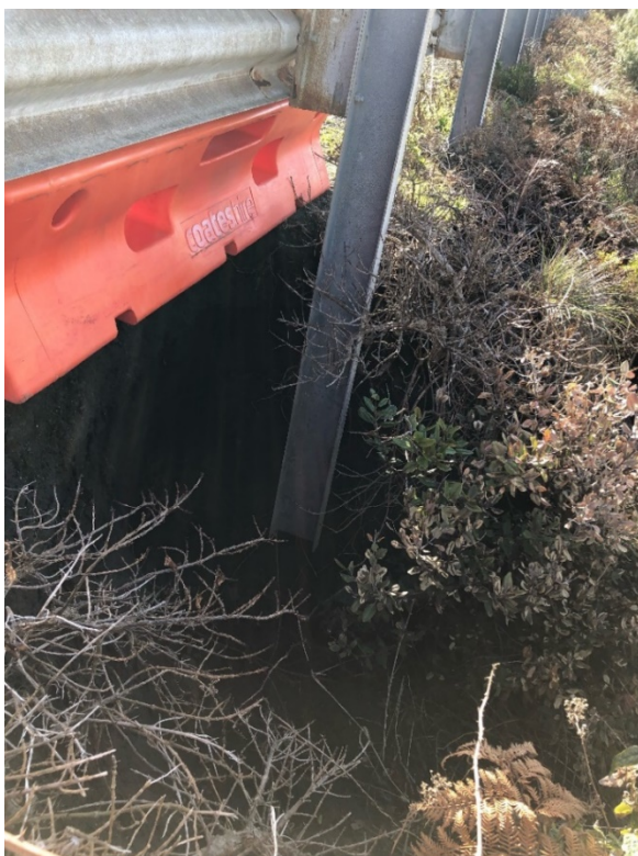
Photo – May 2021 erosion under roadway at the stormwater outlet. Erosion has deteriorated to the point that the guard rail posts are no longer supported, making them an ineffective road safety treatment.
