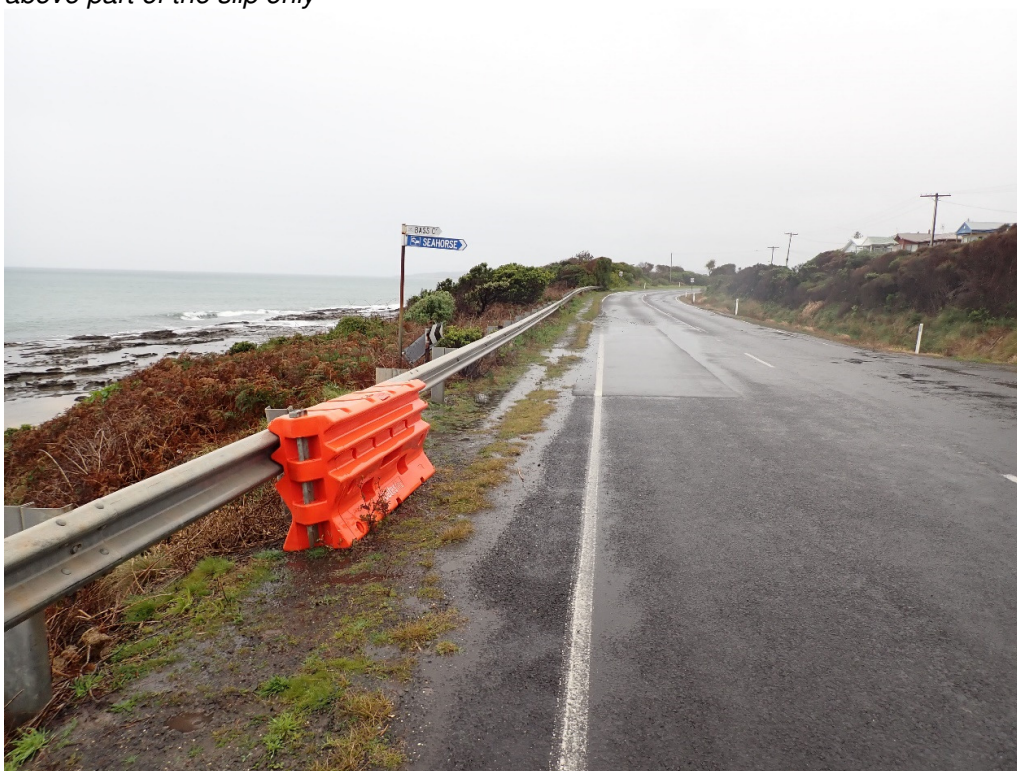
Photo 2 View looking west along Great Ocean Road. Note flow of surface water on the outer side of the road flowing downhill towards the failed area and exiting over the edge. Note the barrier is now leaning further seaward as further distortion of the guardrail and supporting ground is occurring.
