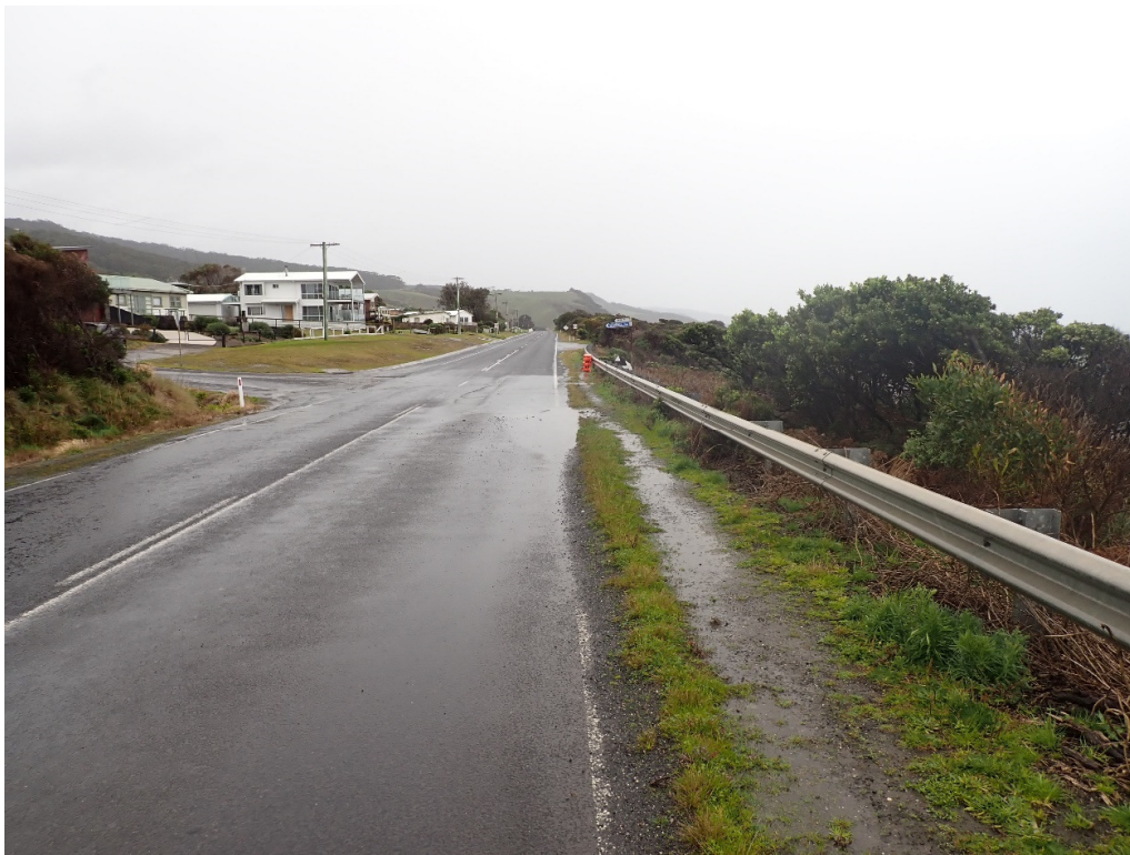
Photo 3 Alternate view of surface water travelling downslope to the failed area. Generally no signs of distress in road pavement above the slip area
