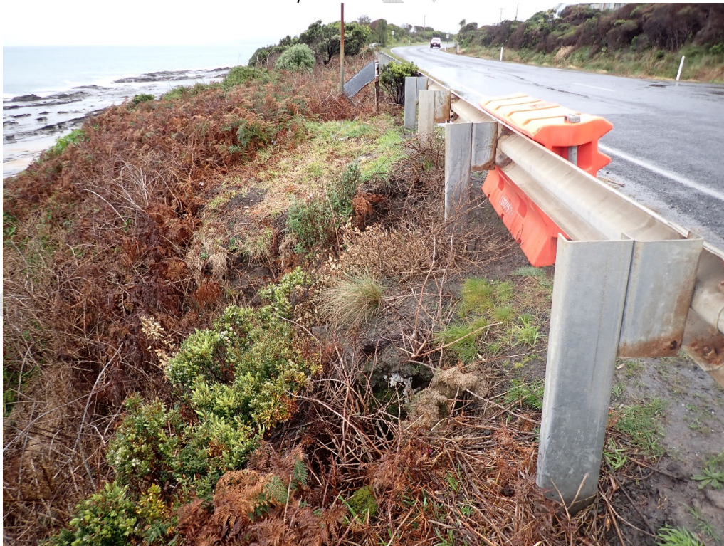
Photo 8 View of the eastern extent of the slide which extends beyond the safety barrier. The stormwater pipe is located within the center of the slide and can be seen protruding into the slide area opposite the end of the barrier (see site plan).
