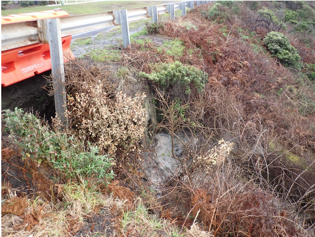
Photo 9 View of the stormwater pipe and end headwall (center of the photo) extending into the slip area. The pipe and headwall are located within the center of the overall slide area (see site plan).
