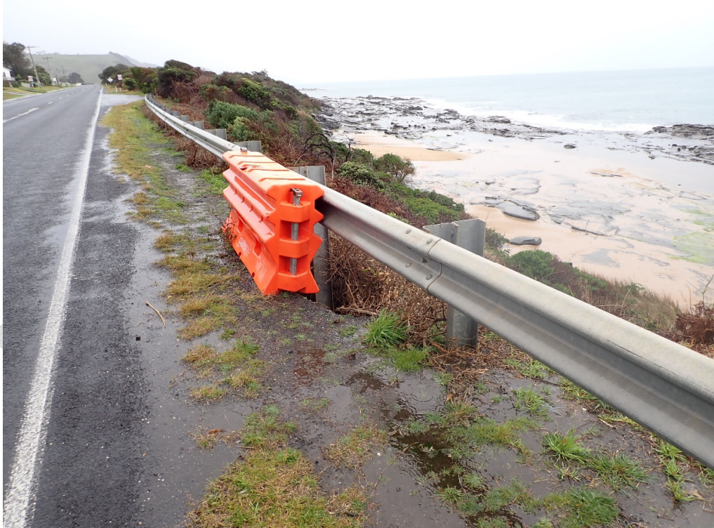
Photo 4 Western extent of the slip with surface water flowing over the backscarp of the slip
