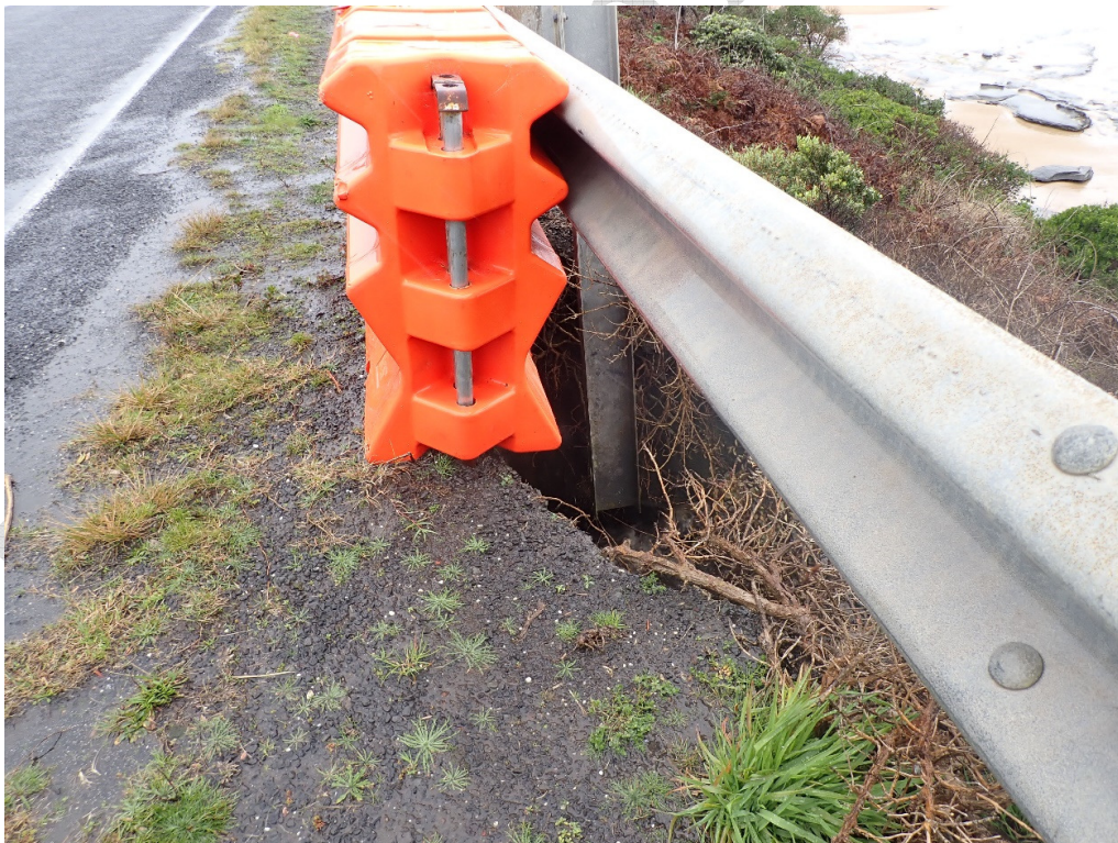
Photo 6 Edge or backscarp of the slide at the western extent has retrogressed under the orange safety barrier
