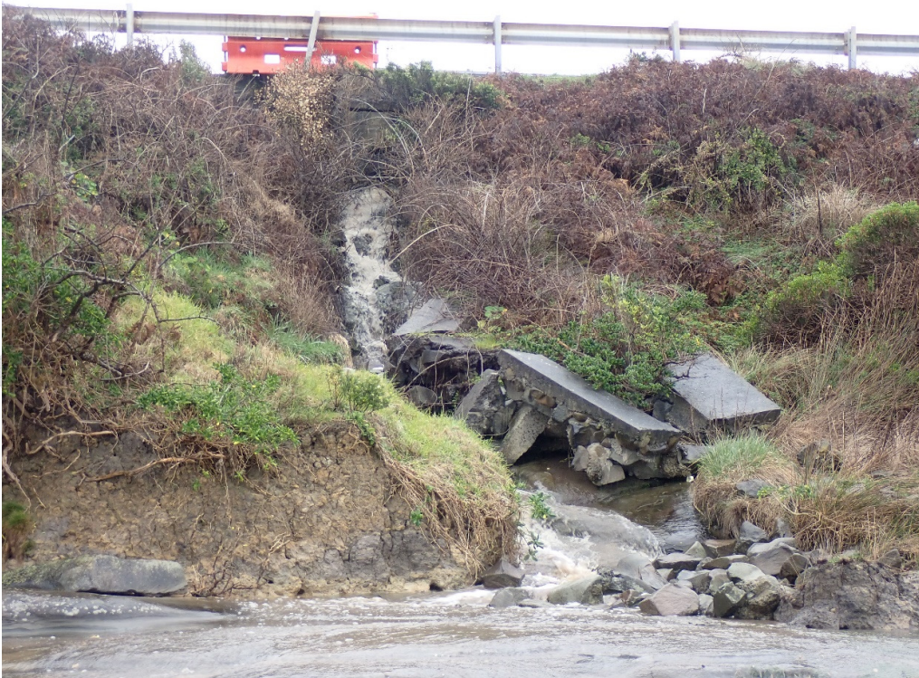
Photo 12 Overall view of slide area. Note failed landslide debris on left hand side of the photo. The channel appears to have a sandstone base although other rock revetment and concrete slabs are evident within the channel possibly indicating previous attempts to stabilize the area.
