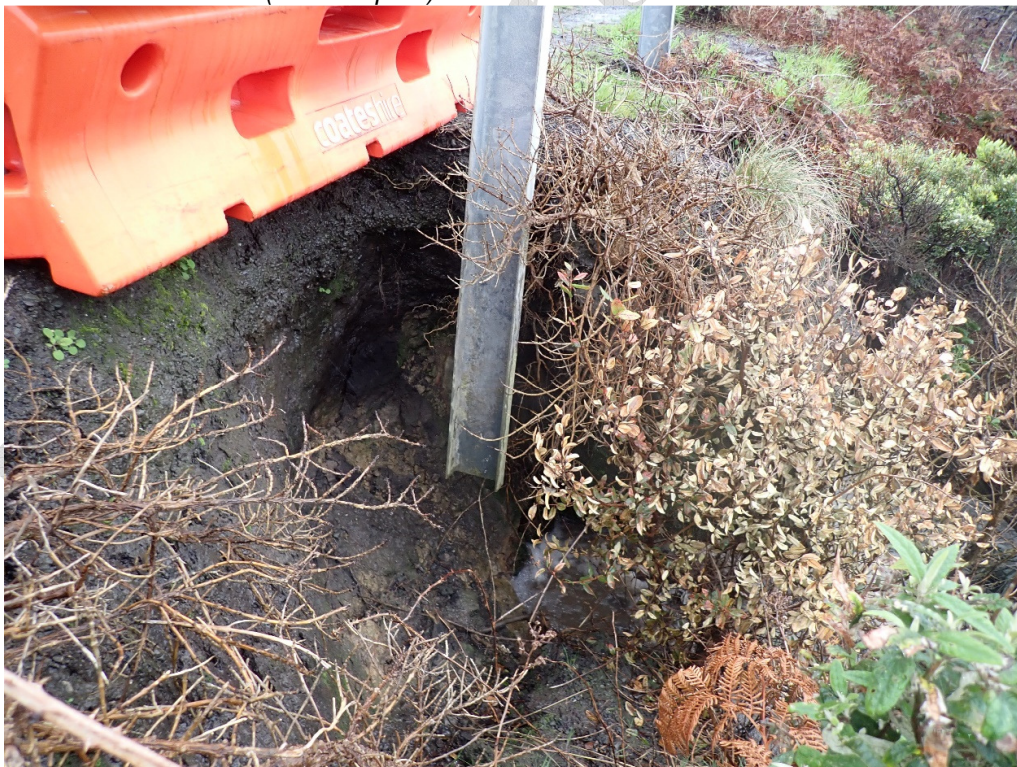
Photo 10 The stormwater pipe is approximately 800 to 1000 mm in diameter and appears to be still intact at the rear of the cavity. Although the outlet for the pipe was not able to be observed, it clearly does not now correspond with the headwall outlet as significant flows were noted discharging before and below the headwall .
