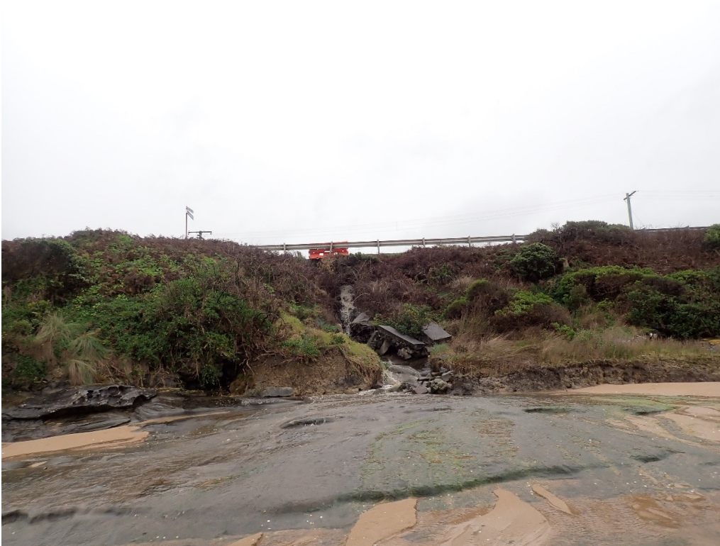
Photo 11 View of the slide area from the beach below looking north towards Bass Crescent The slide area is defined by browned off/dead vegetation. Colluvium and previously failed landslide debris is evident at beach level on both sides of the outlet channel.
