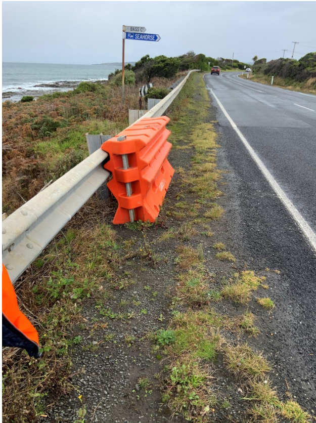
Photo – May 2021 showing the proximity of the erosion to the traffic lane.
