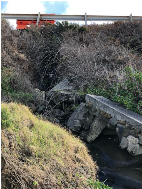
Photo – May 2021 showing the disturbed outlet point which is contributing to the erosion.
