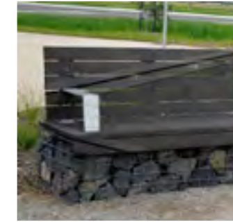
Gabion and metal seating
