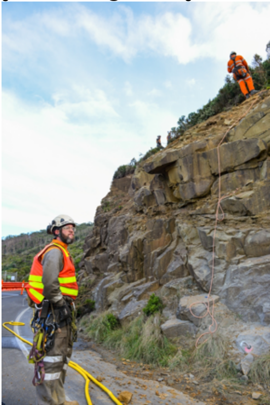
Stabilising the cliff face just west of Lorne in preparation for installing rock fall netting.
