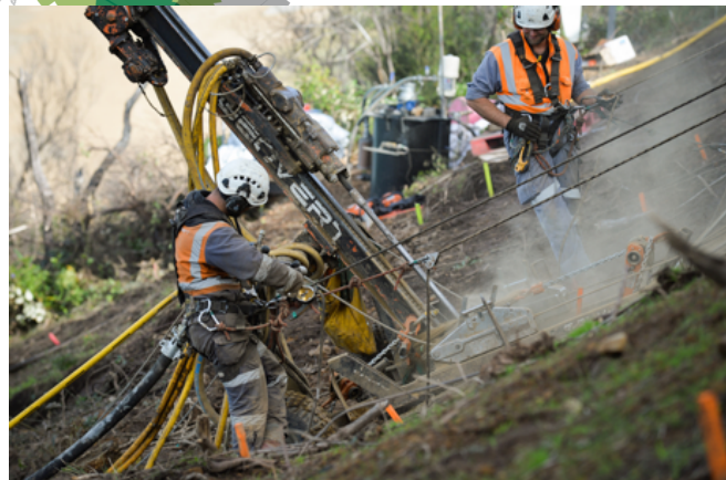
Soil nailing the Paddy’s Path hillside at Wye River
