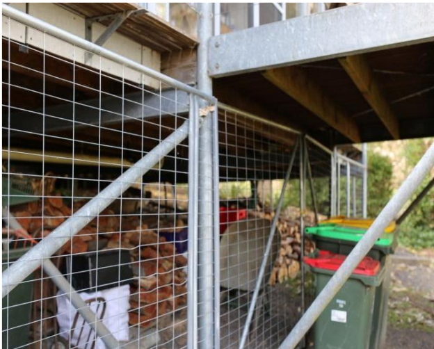
Figure 23: Heavy fuel stored under a house
