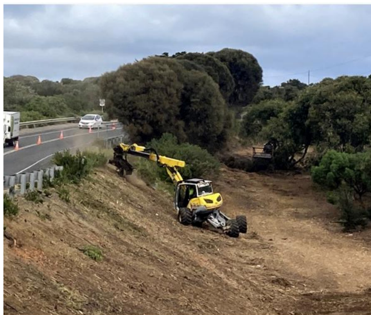
Figure 30: Image of construction of Strategic Fuel Break along the Great Ocean Road Aireys Inlet.
