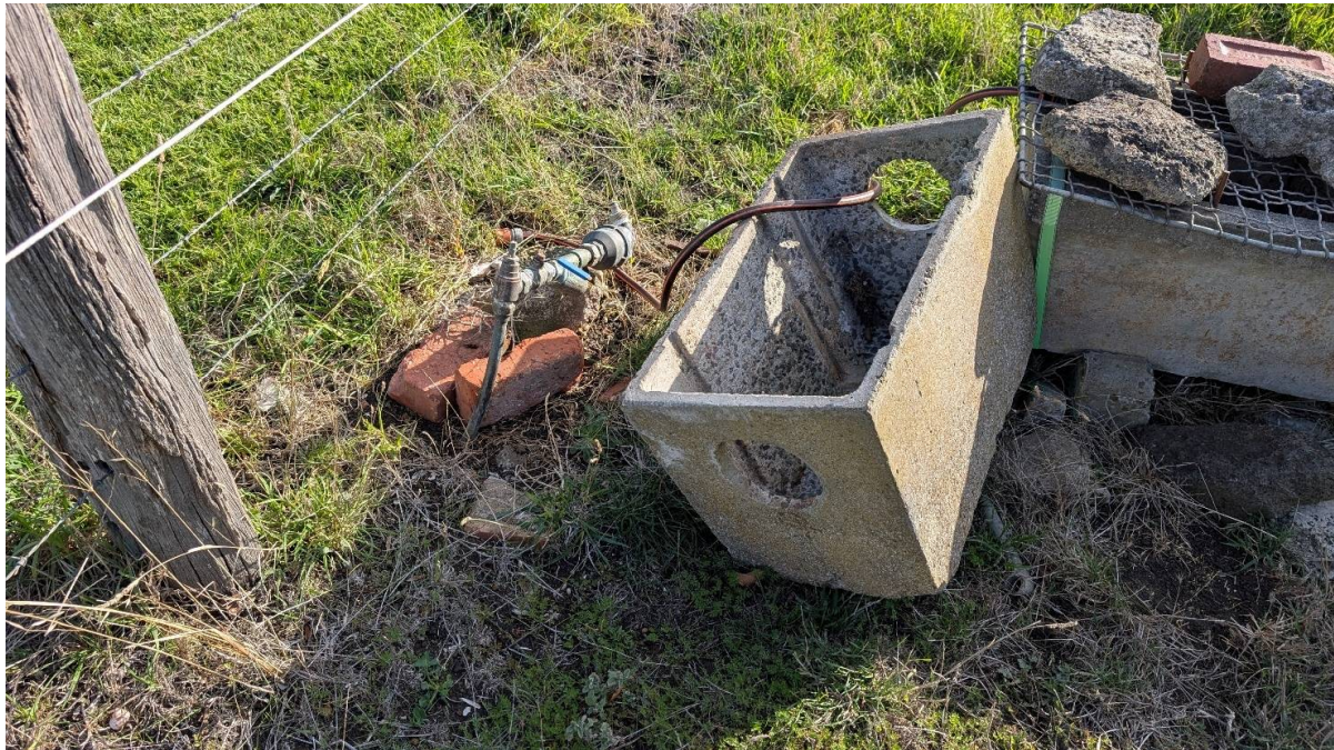
Image 7: The existing town water connection will remain the main supply.
