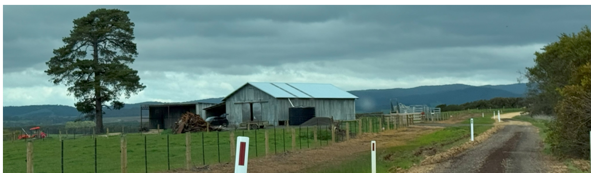
Figure 8 - Existing shed at the subject site
