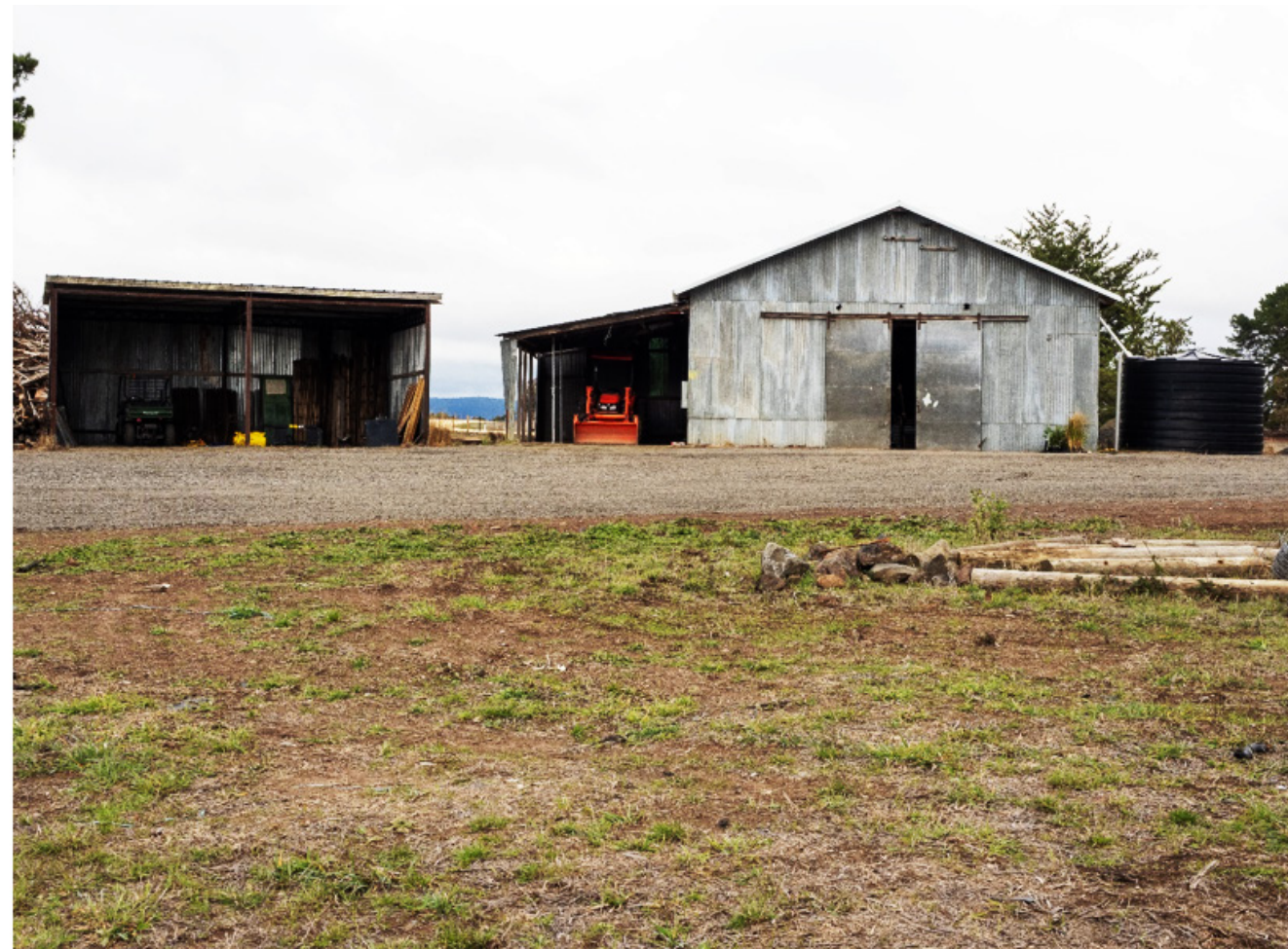
12 EXISTING FARM SHEDS
