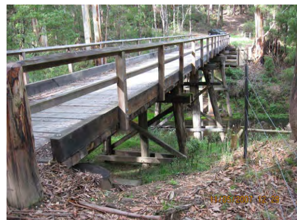
Bridge Structure (Composite)
