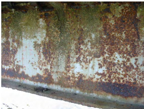
Corrosion of Steel Beams
