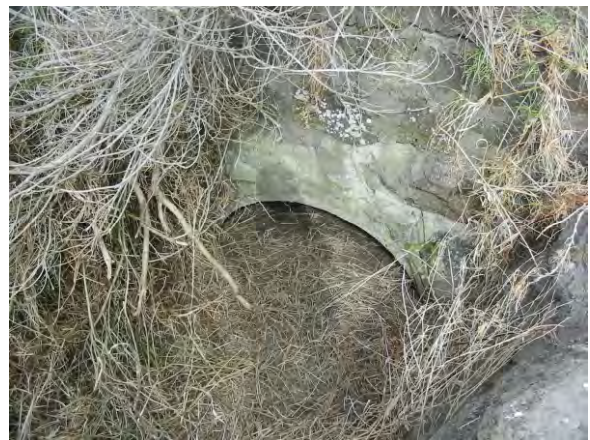
Blocked Culvert/Waterway
