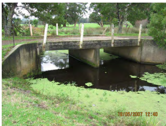
Major Drainage Structure (Box Culvert)
