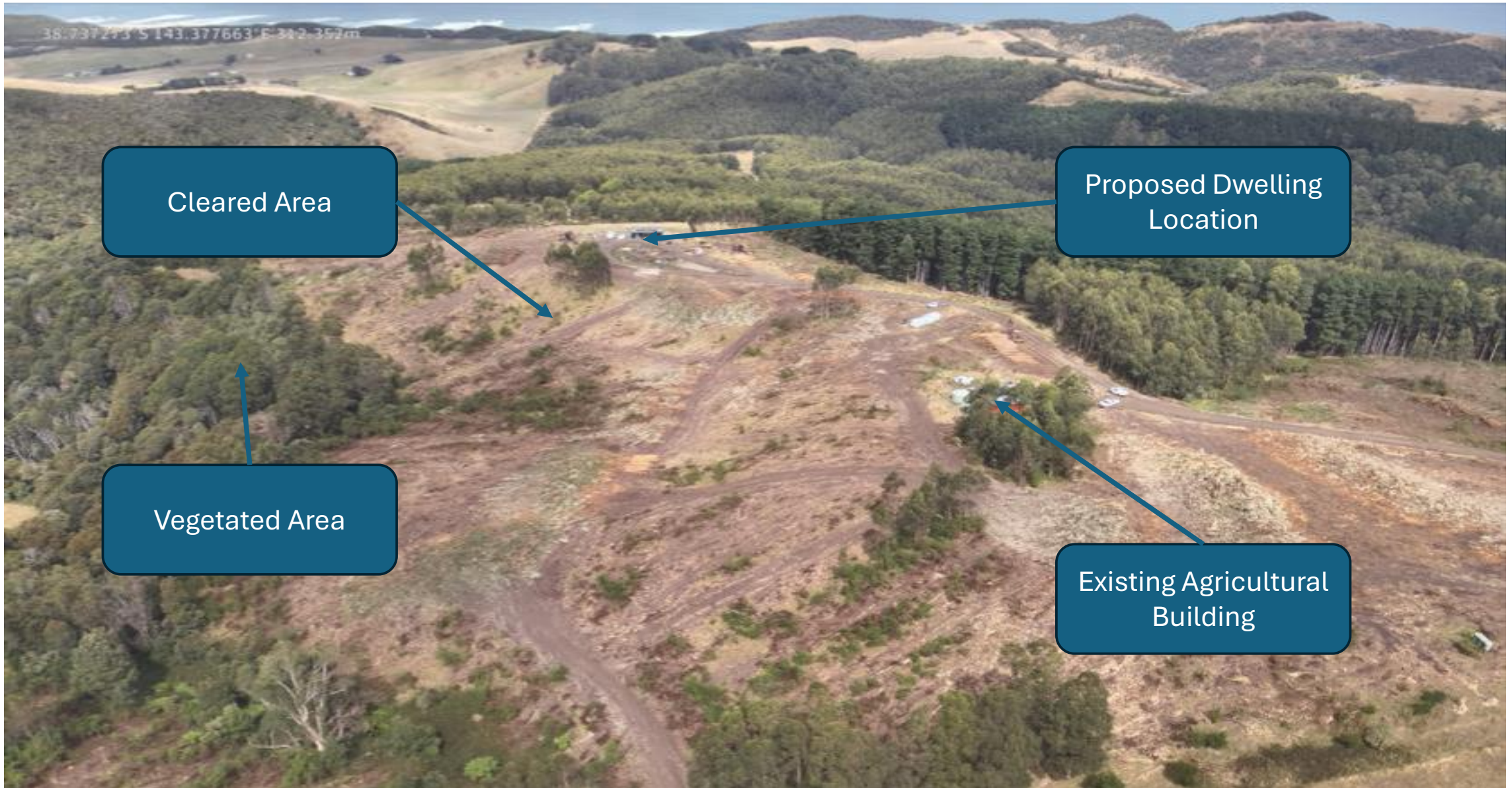
Image 2 - Drone photo (provided by applicant) looking north-east post timber harvest
