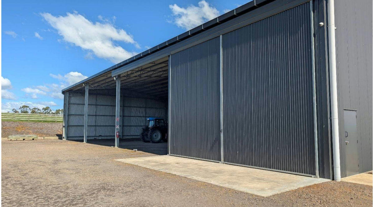
Image 6: Recently constructed farm shed,
