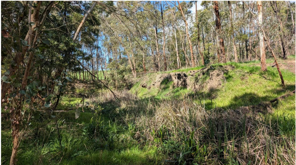
Image 11: Deans Creek showing old erosion scars.
