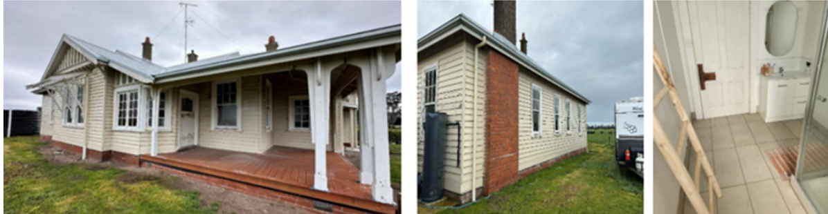
Figure 4 – Images of existing dwelling (Source: Permit Applicant)
