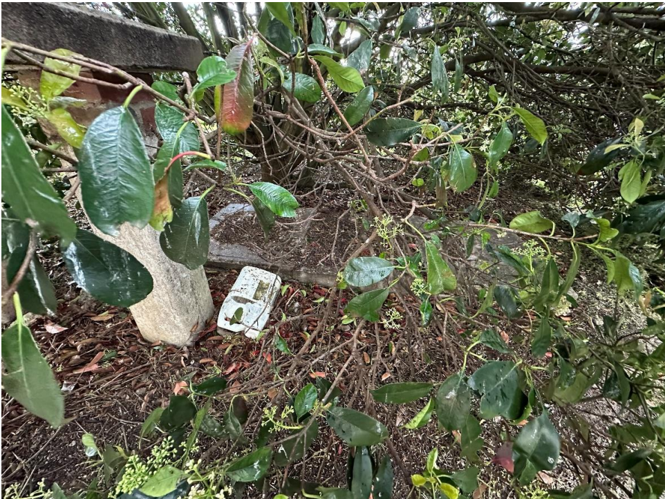
Location of the long-term septic system, see concrete pit.
