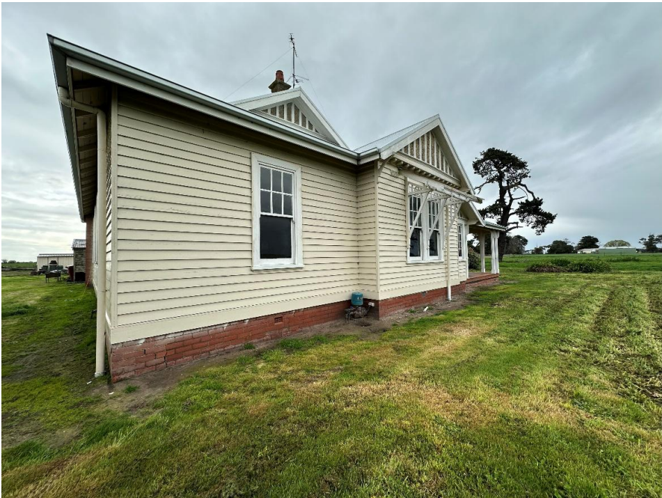
More renovation improvements.
