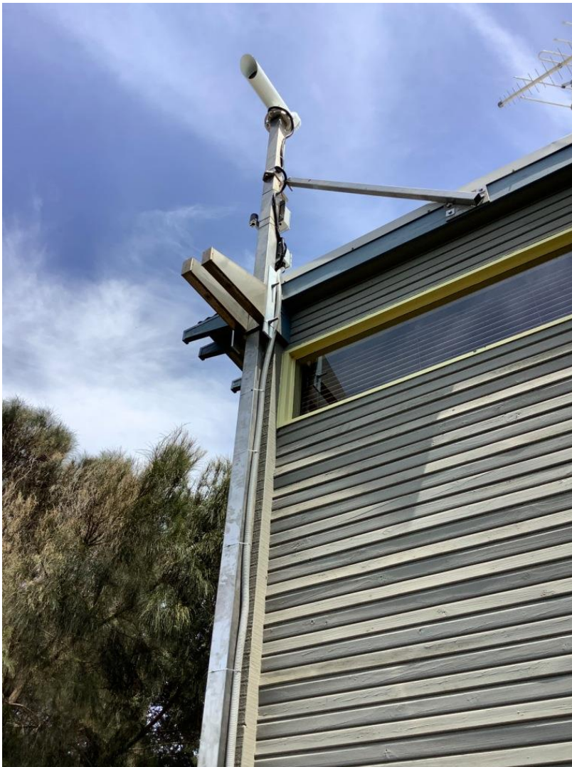
Picture 1- New directional light
