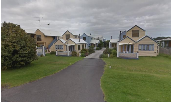
VIEW OF 9-13 NOEL STREET LOOKING SOUTH FROM NOEL STREET
