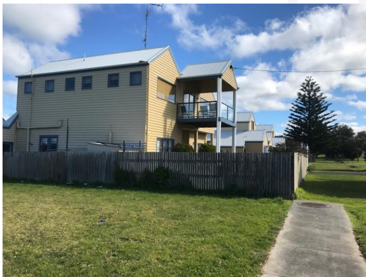
VIEW OF 9-13 NOEL STREET LOOKING WEST
