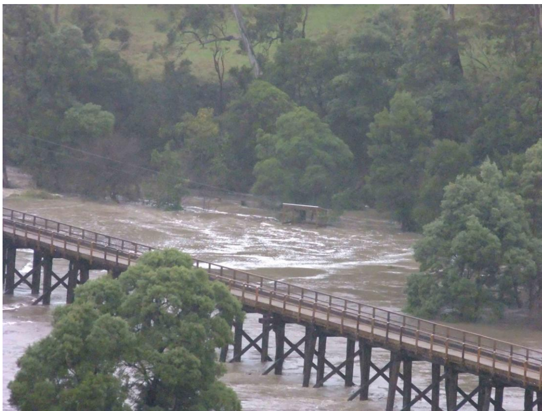
Curdies River at the Trestle Bridge, Curdie. Highest level reached on record at this site.
