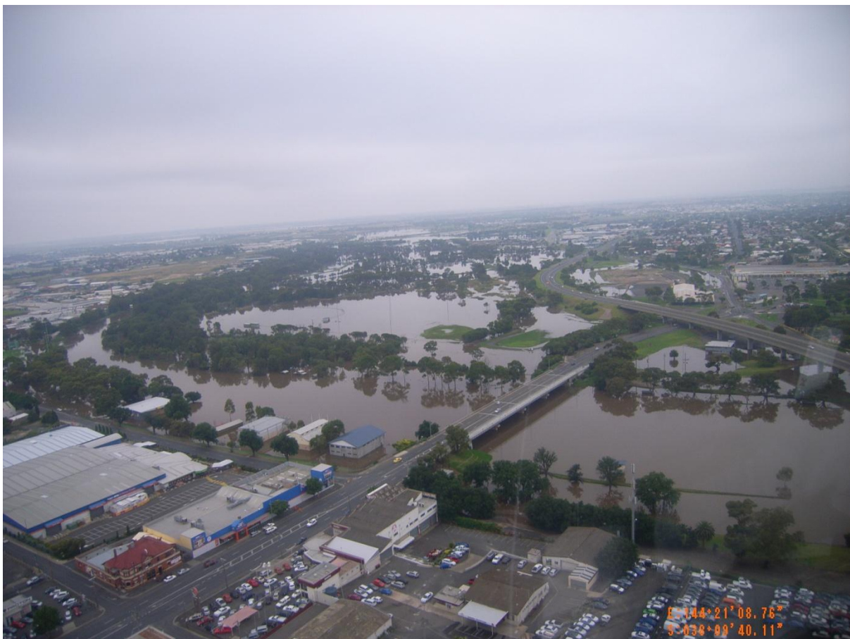
Jan 2011 Barwon River flood at Moorabool Street Bridge Geelong
