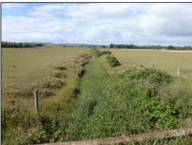
Plate 8. Deans Creek intersecting Back Larpent Road (east of Deans Creek Road – looking south)
