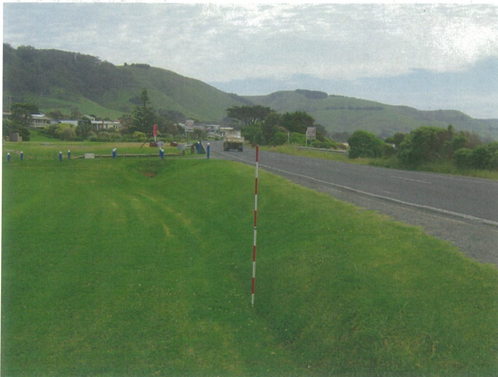
Plate 4: The Great Ocean Road road reserve near the outlet of Milford Creek. Note how the road has been raised above natural ground level.
