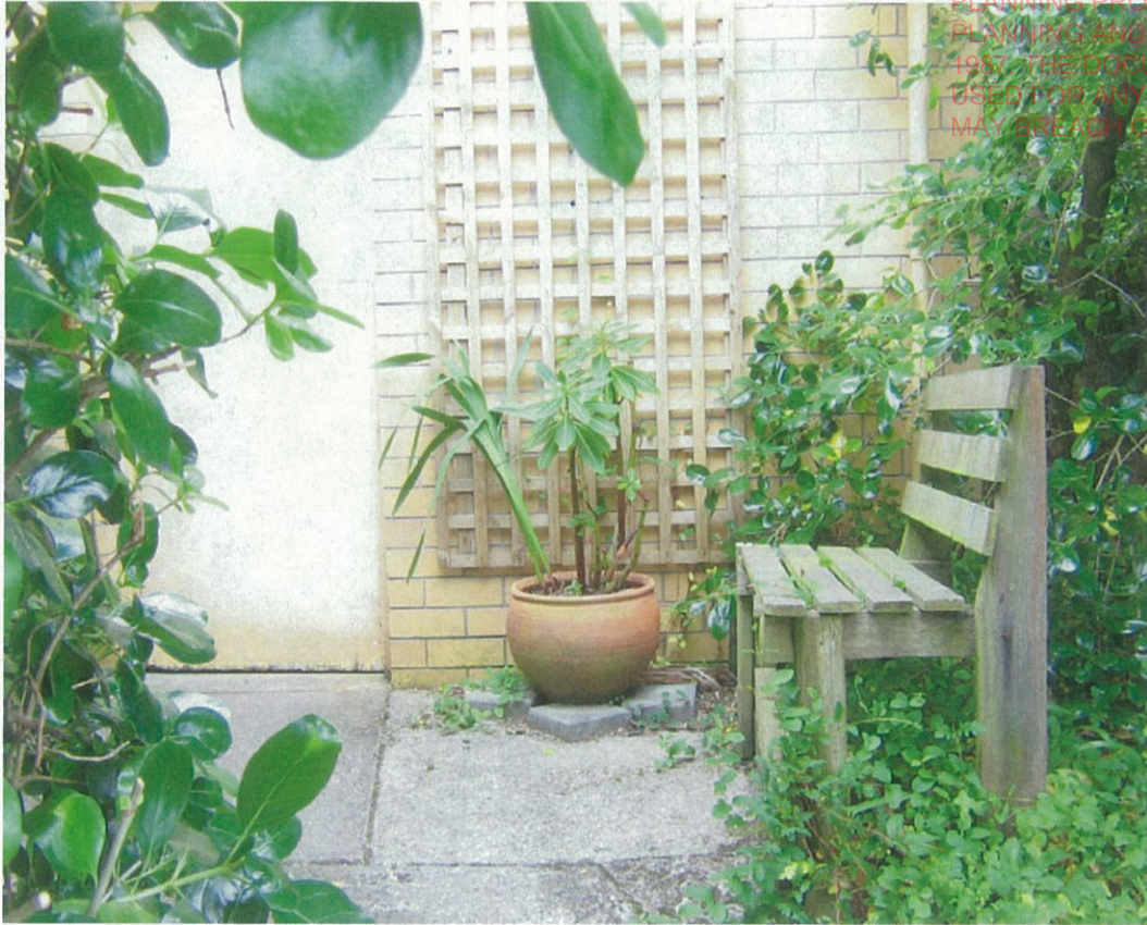
Plate 9: Entrance to the rooms on the southern side of the brick residence which have been dug into the hillside. ie these rooms are below the natural ground levels.
