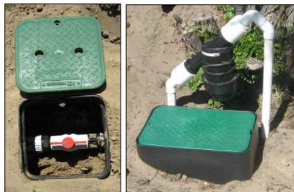
Figures 26-27 – Flush valve, subsurface irrigation trenches; filter (Source: Mornington Shire Council 2014).
