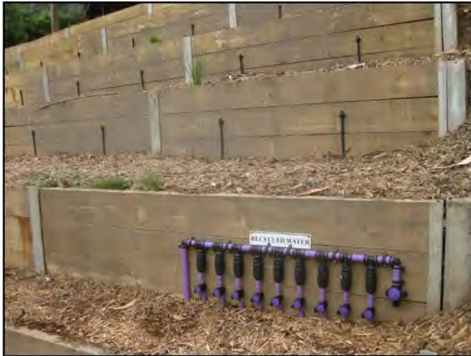
Figure 3: Typical multi-tiered irrigation disposal
