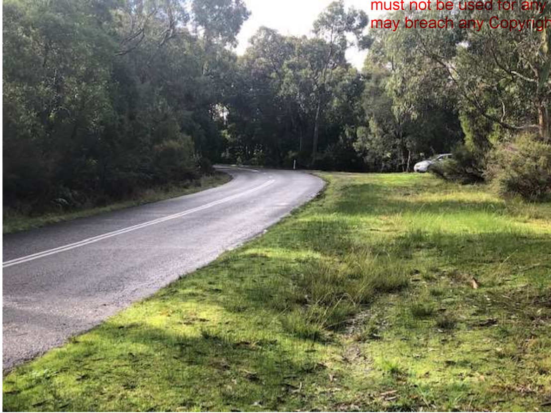
Photo 8: Proposed road access point to east.
