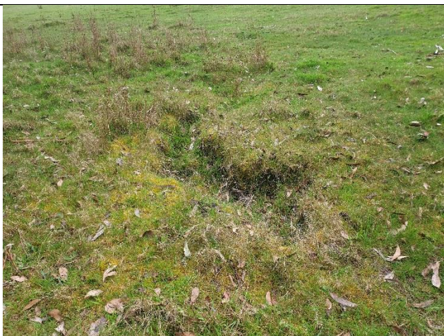
Photo5: Tunnel erosion in the north-western corner of the property.
