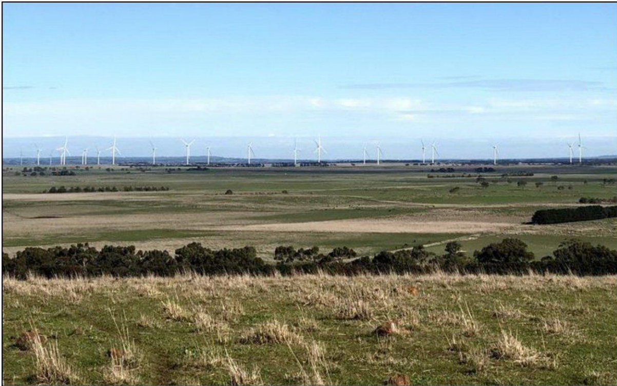
Figure 16: View southwest across neighbouring properties from the proposed site location to Mt Gellibrand Wind Farm
