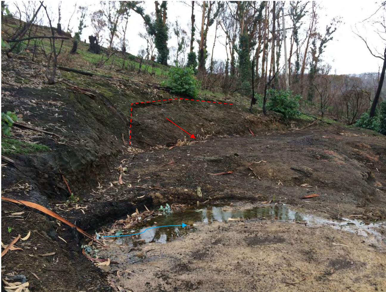
Photo 89 Slumping of cut slope in residual material (Unit 2) on 4 Iluka Avenue with strong seepage from broken stormwater in the foreground.
