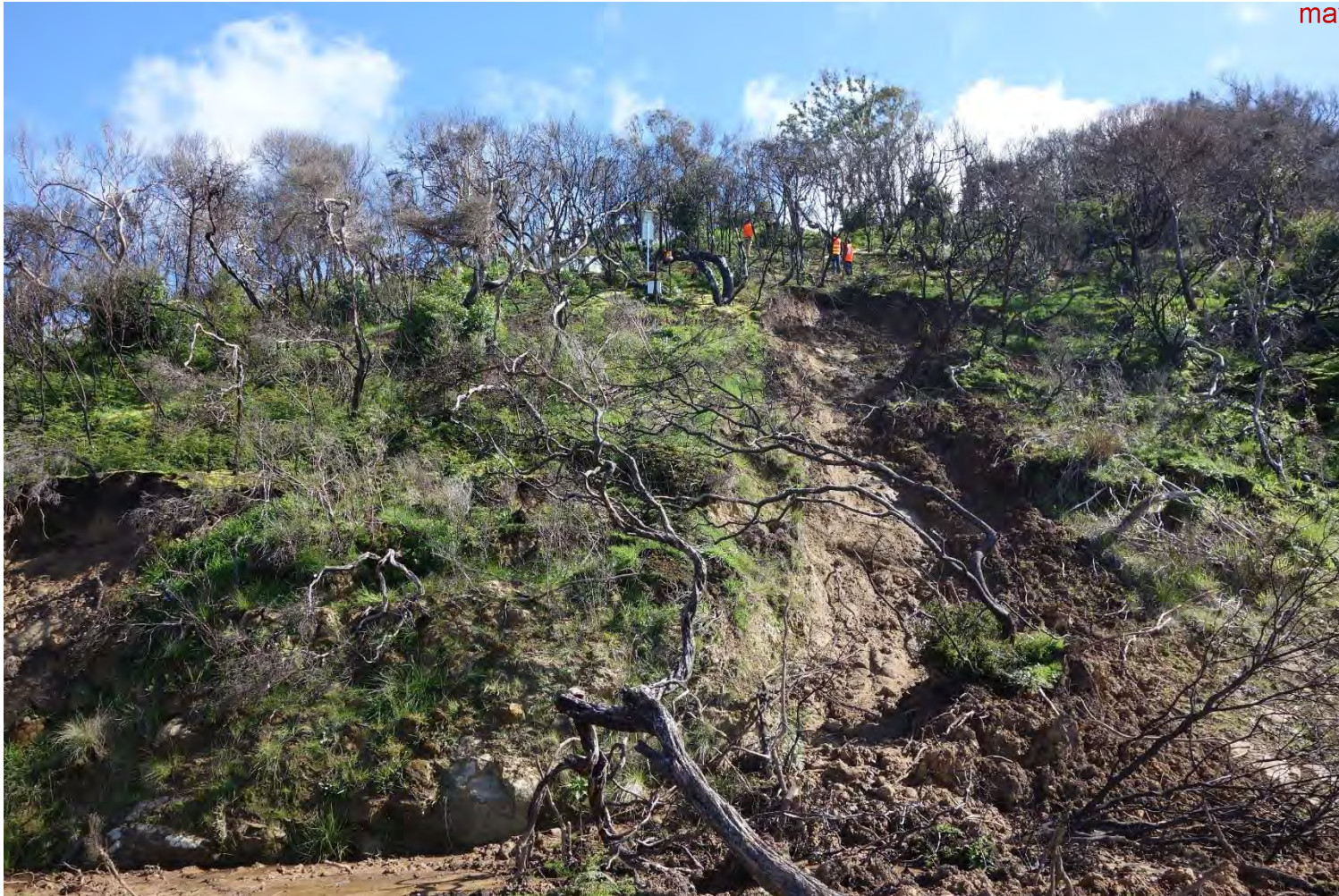
Photo 4 Regression of Paddy's Path failure following heavy rainfall in September 2016.
