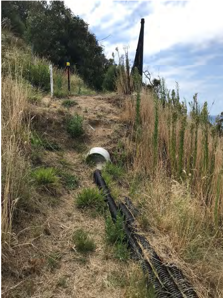
Photo 16 VicRoads retaining wall works at 25 Iluka Avenue – February 2019.
