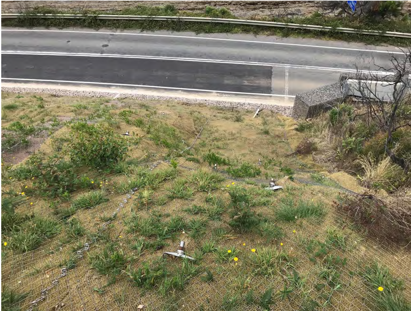
Photo 13 VicRoads remedial works of Great Ocean Road.
