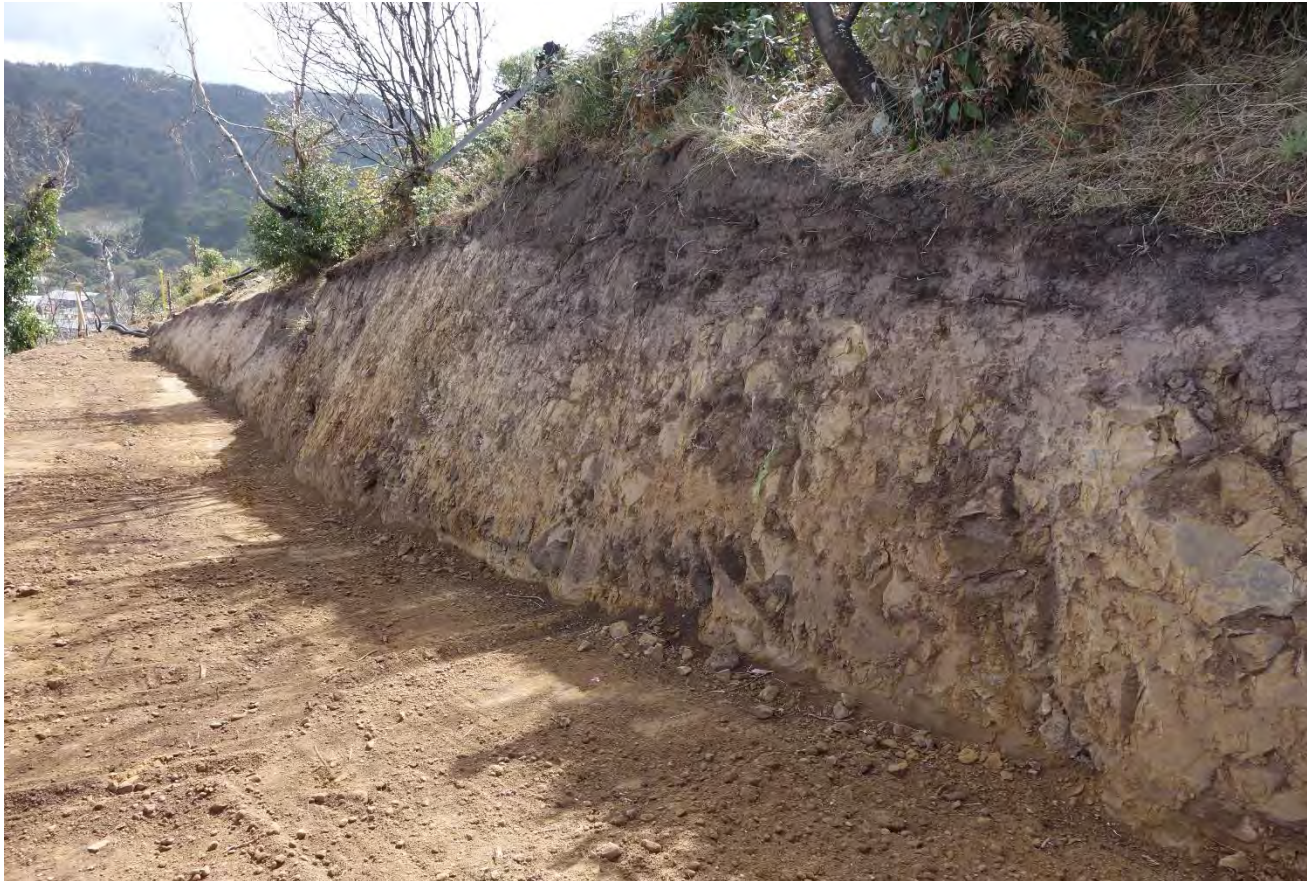
Photo 15 VicRoads retaining wall works – Slope 1 at 25 Iluka Avenue. Soil Profile of Colluvium overlying Highly Weathered SANDSTONE (at base of cut).
