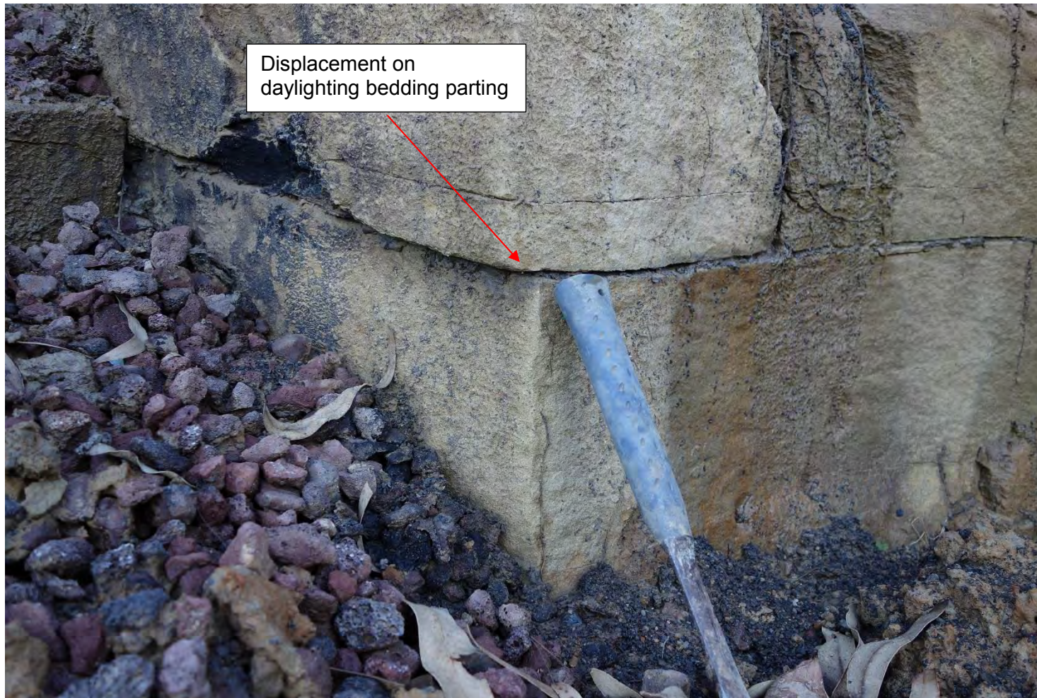
Photo 6 Burnt out retaining wall at 23 Iluka Ave - Displacement on bedding surfaces in Unit 3A.
