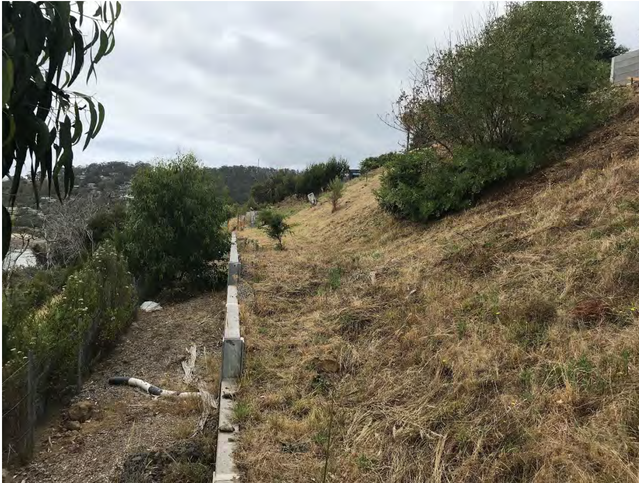
Photo 9 New Retaining walls below 17 Iluka Avenue looking south west with moderate back slope (for ~1.5 m width) immediately behind the wall.
