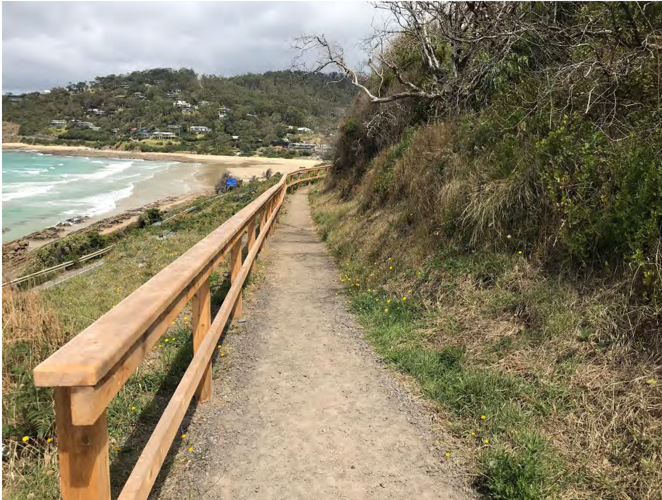
Photo 14 VicRoads remedial works at proposed outlet from 18 Iluka Avenue. Soil Nail and Mesh with drainage immediately downslope of hand rail.
