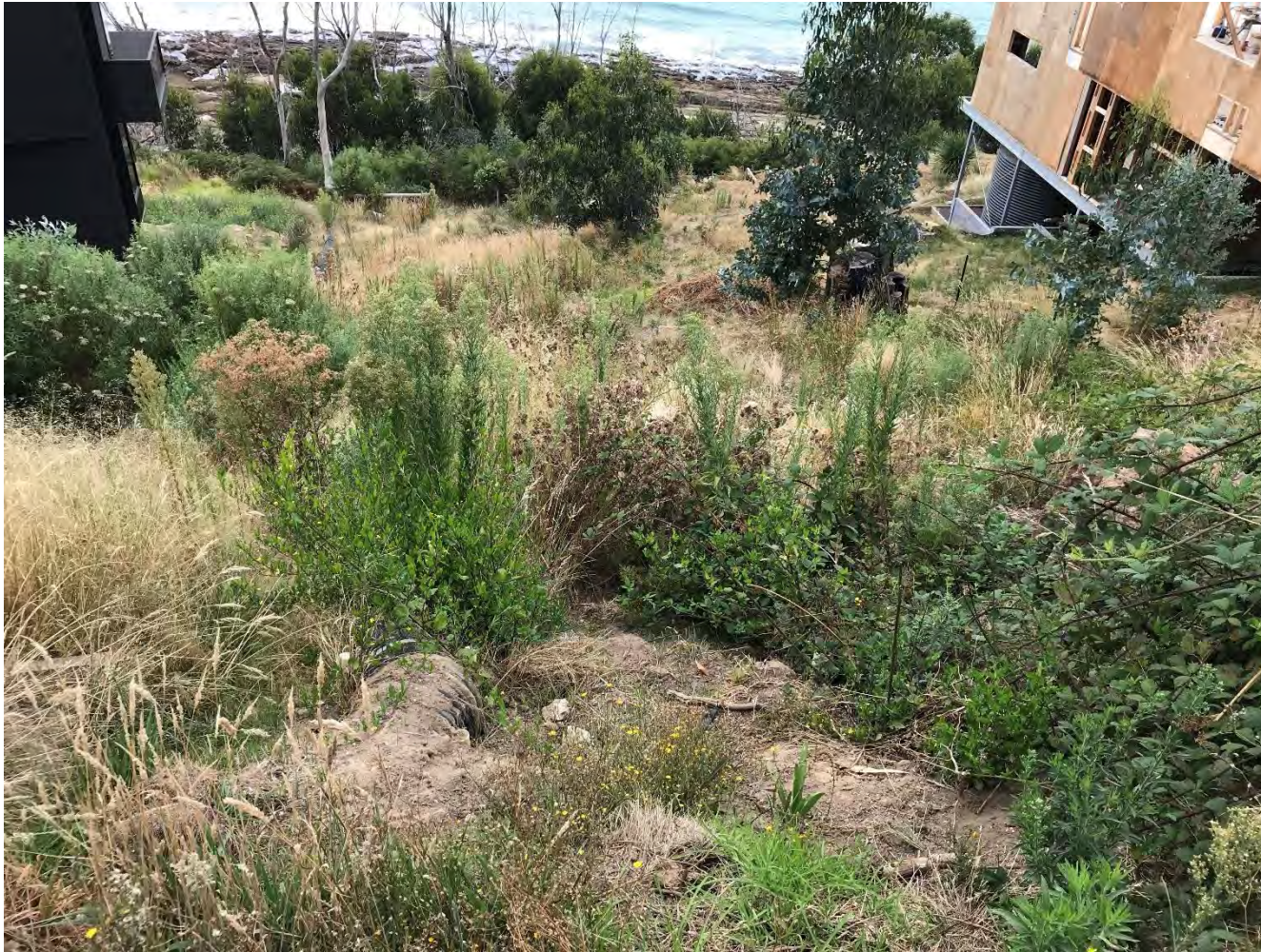
Photo 12 Typical Slopes in drainage easement between 13 and 14 Iluka Avenue.
