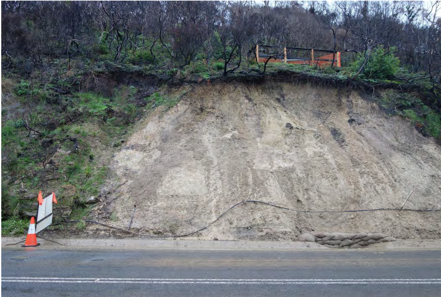
Photo 5 Small translational failure above the Great Ocean Road, looking north with highly weathered Sandstone bedding observed near the toe. Bedding does not appear to be undercut and sliding is occurring at the interface of colluvium/residual and the underlying more competent rock mass.
