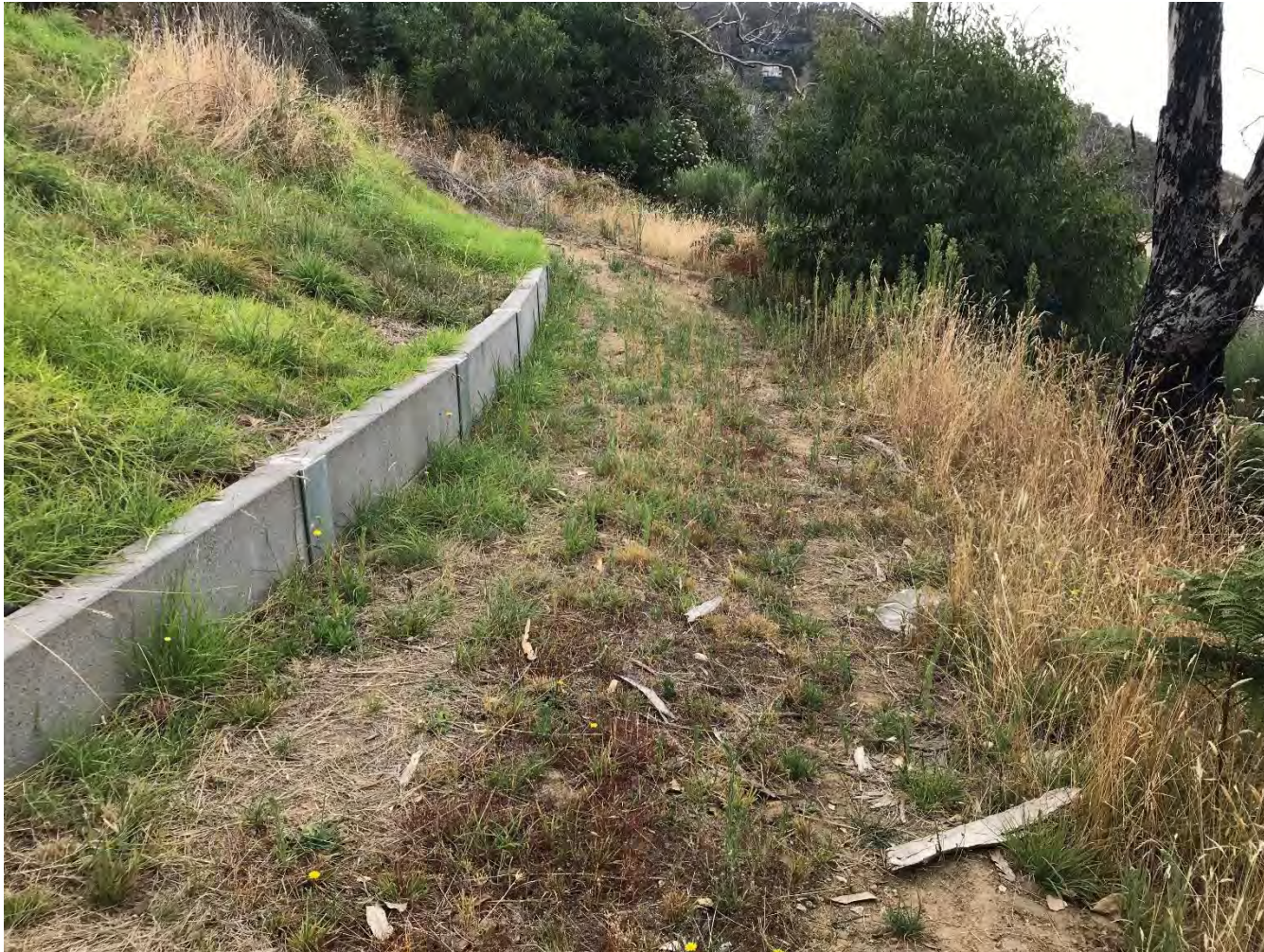
Photo 10 New Retaining walls below 10 Iluka Avenue with existing access track immediately below.
