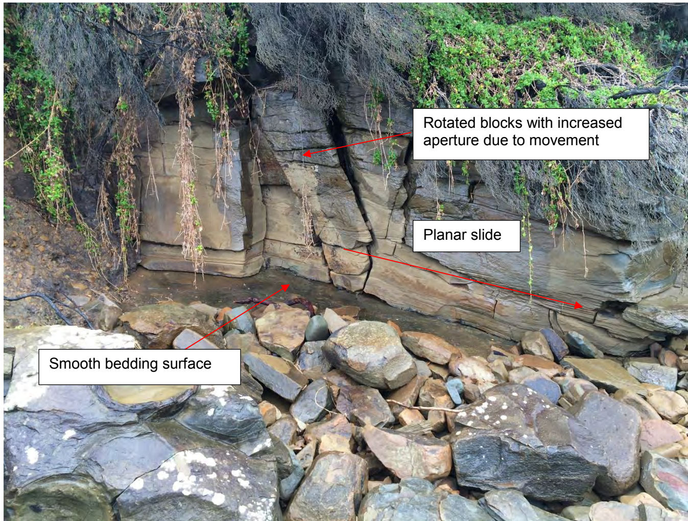
Photo 2 Planar slide of Moderately to Slightly Weathered SANDSTONE on smooth bedding plane
