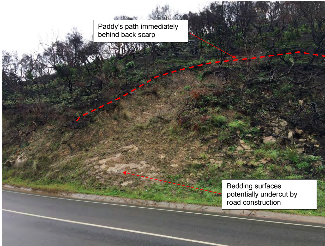
Photo 3 Small translational failure above the Great Ocean Road, looking north west.
