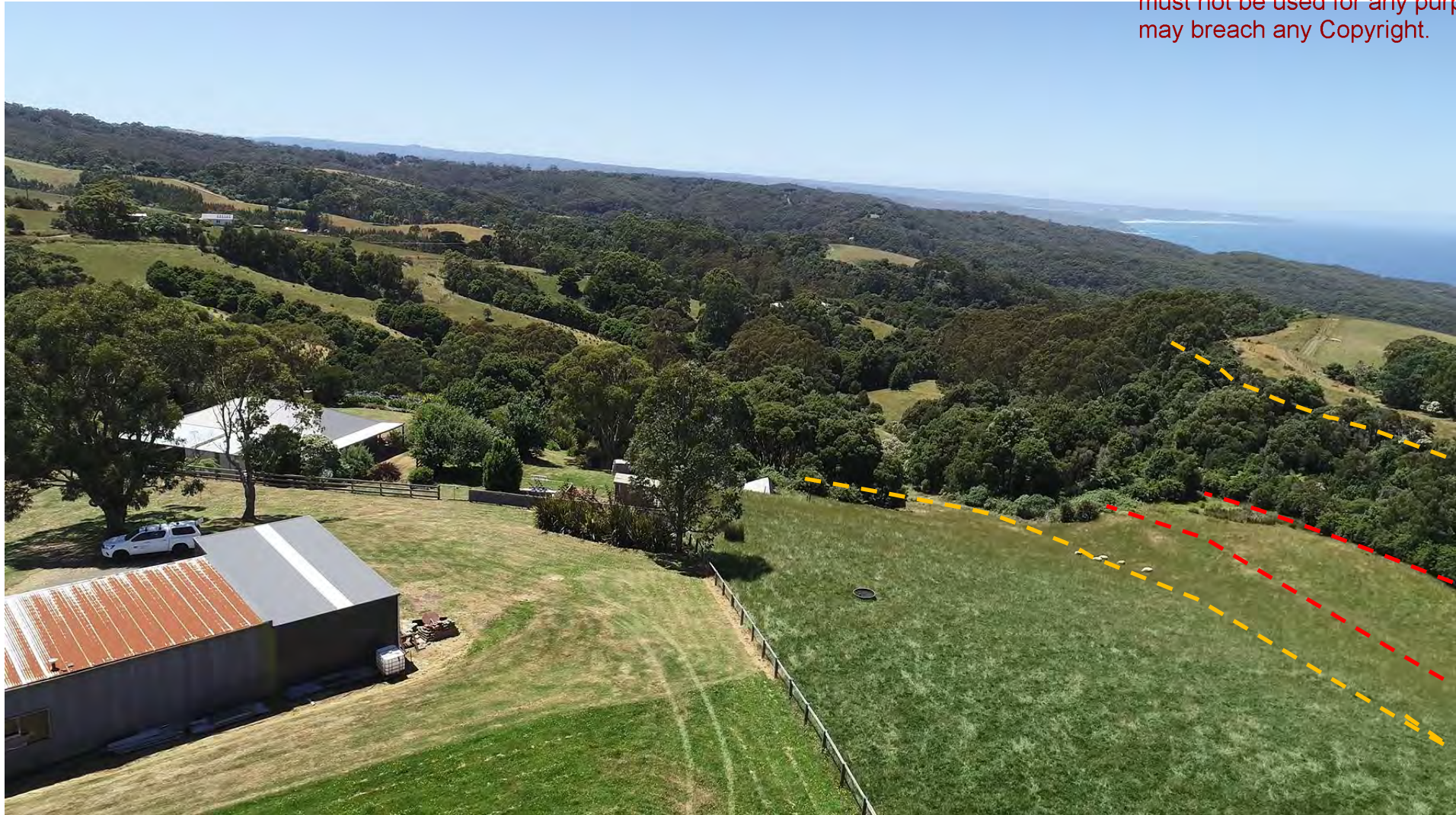
Aerial photograph of proposed staff accommodation development area and inferred landslide
