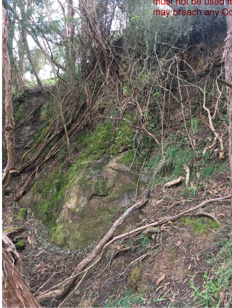
Hornes Road Landslide Feature (downslope from proposed Bushfire Shelter). Note highly to slightly weathered rock in profile.
