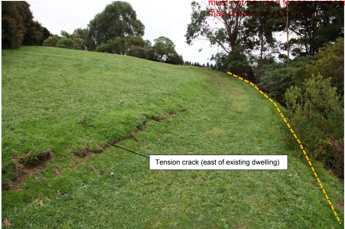
Tension crack and highlighted main scarp
