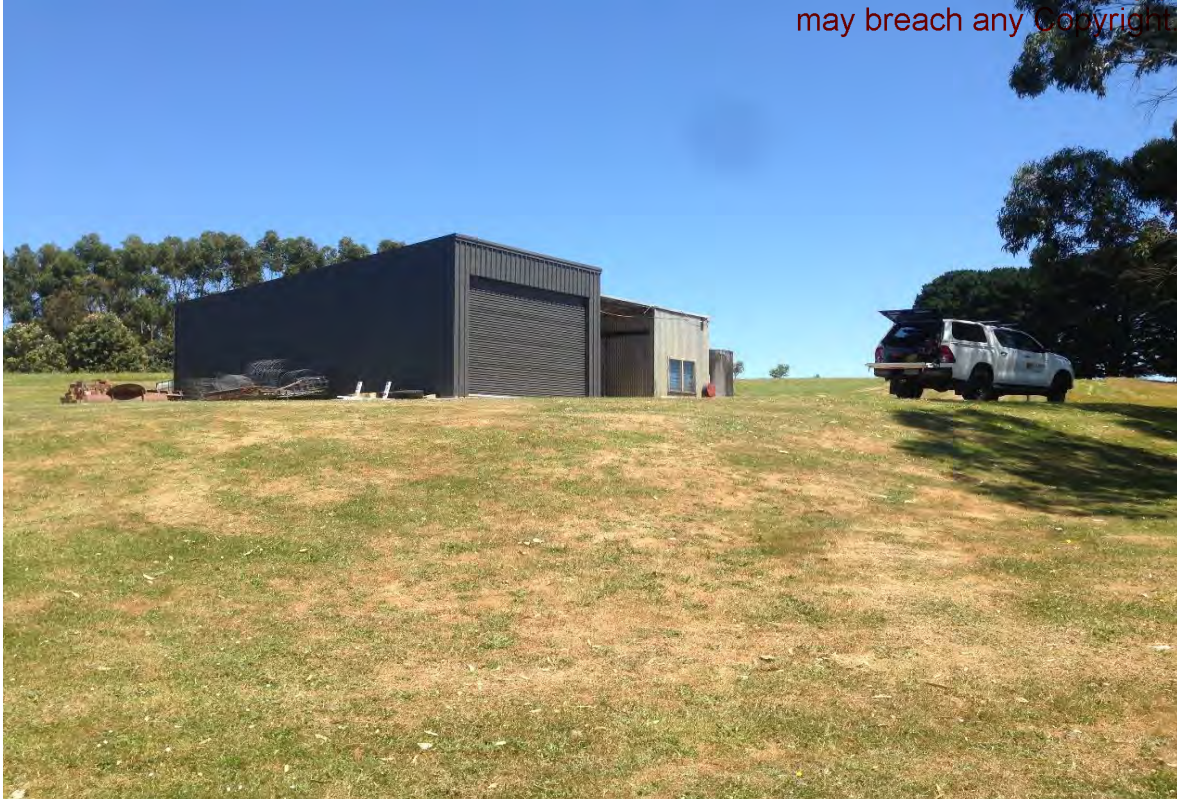
Photo 9: Existing site conditions, existing shed and proposed staff accommodation area.
