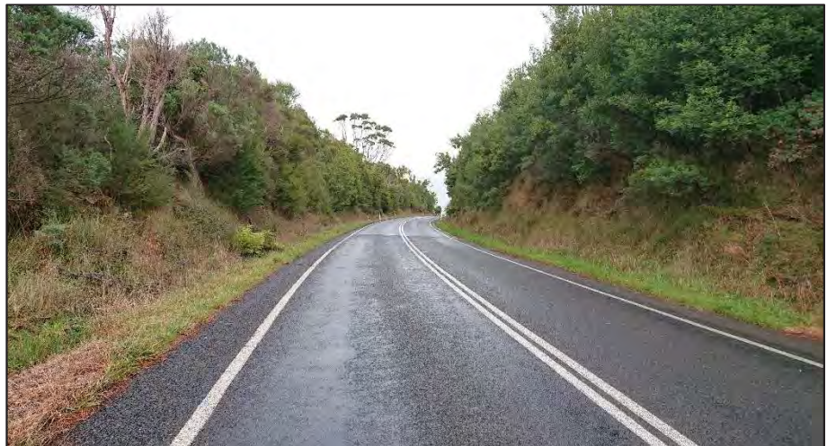
Figure 2.7: East approach to intersection on Great Ocean Road
