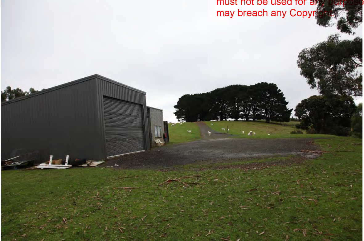
Existing sheds and proposed accommodation area
