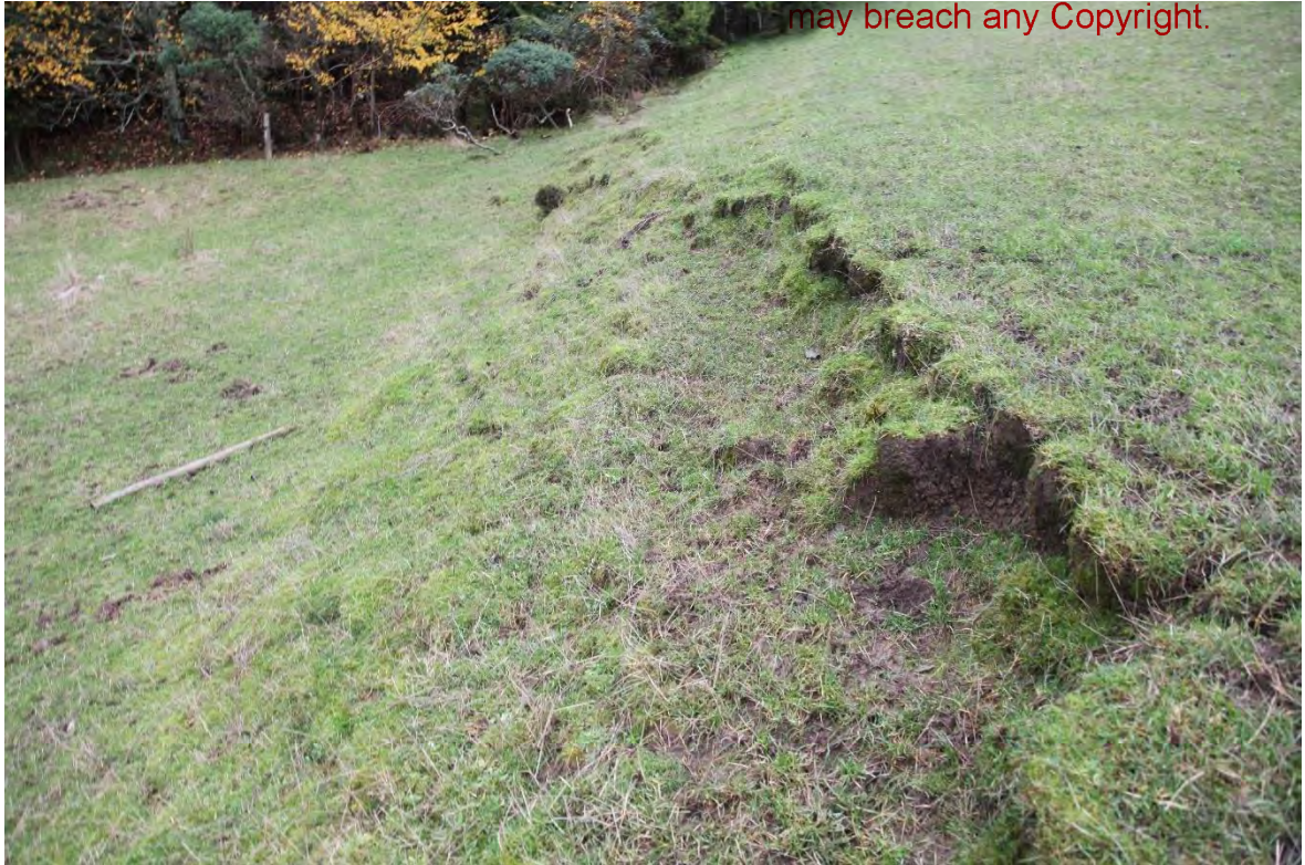
Evidence of recent fretting and slope movement in gully, edge of Hornes Road Landslide (south existing dwelling)
