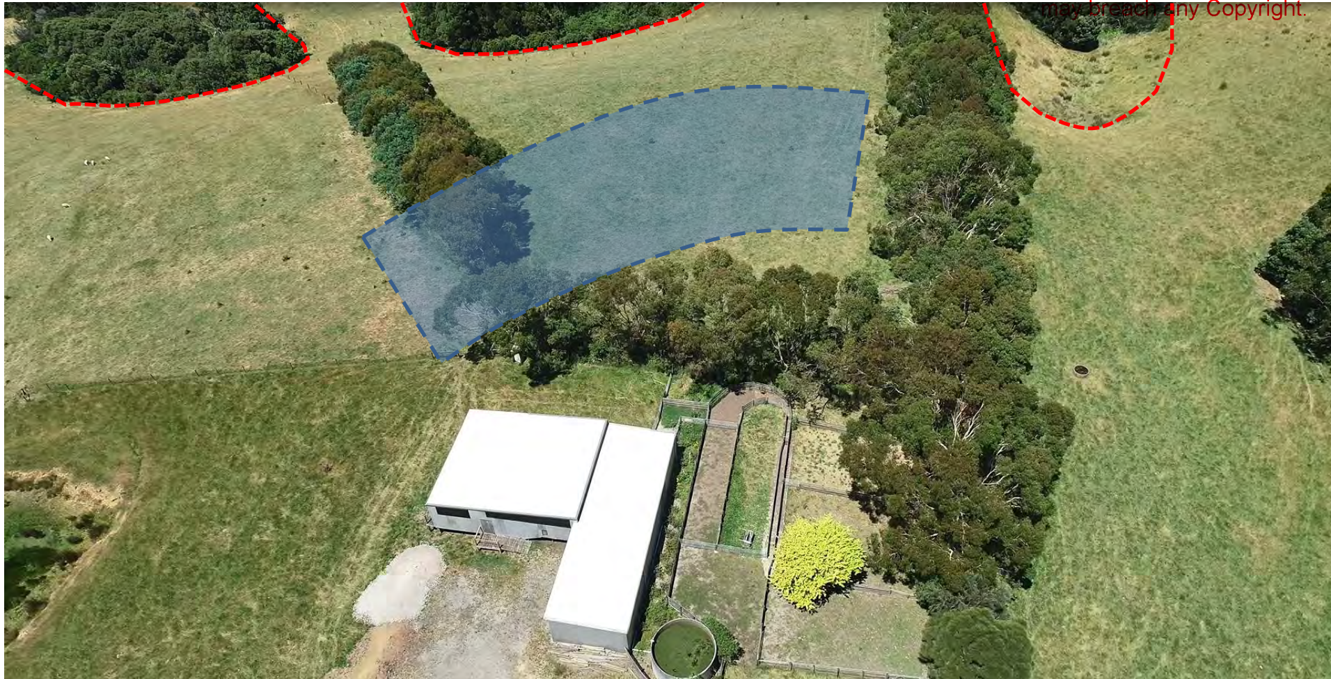
Aerial photograph of proposed dorm development area and inferred landslide features
