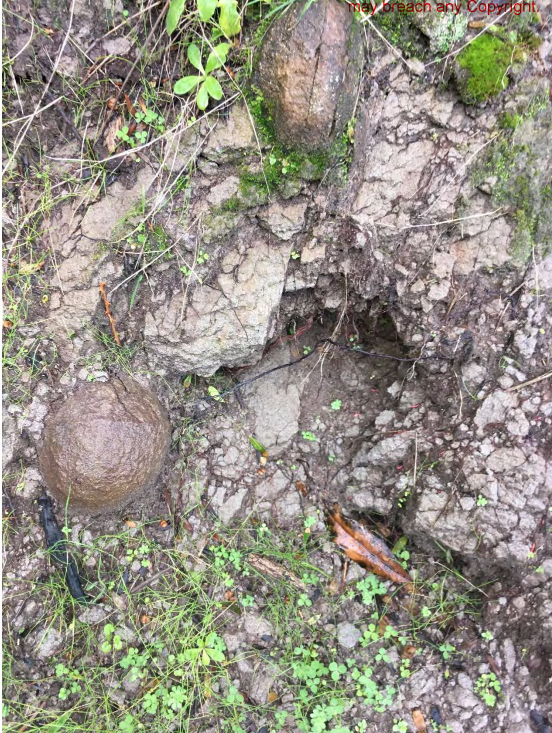
Irregular bedding angles and embedded concretions indicating slope movement (approximately 100m inland)
