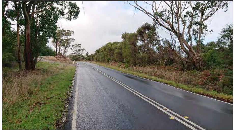
Figure 2.8: West approach to intersection on Great Ocean Road
