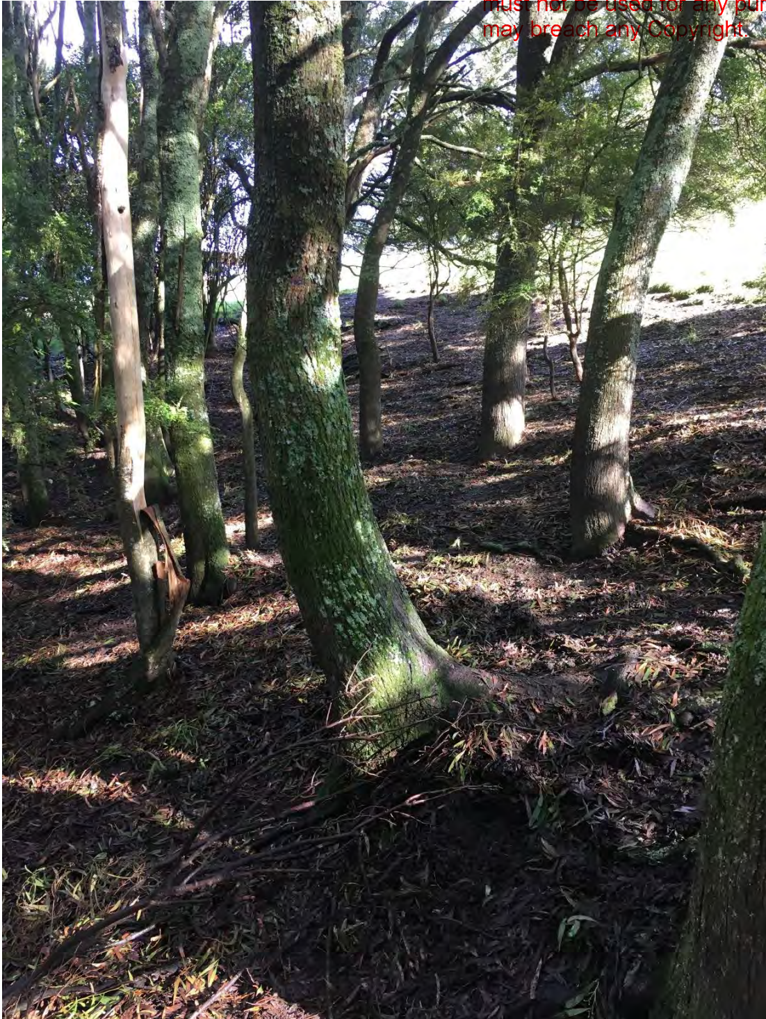
Existing native trees in gully (landslide feature) east of existing shearing shed. Note bent trunks indicating signs of soil creep
