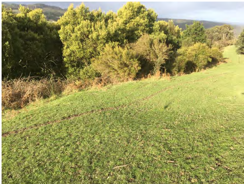
Hornes Road Landslide Feature (downslope from proposed Bushfire Shelter). Note surface depressions, indicating regression of landslide features
