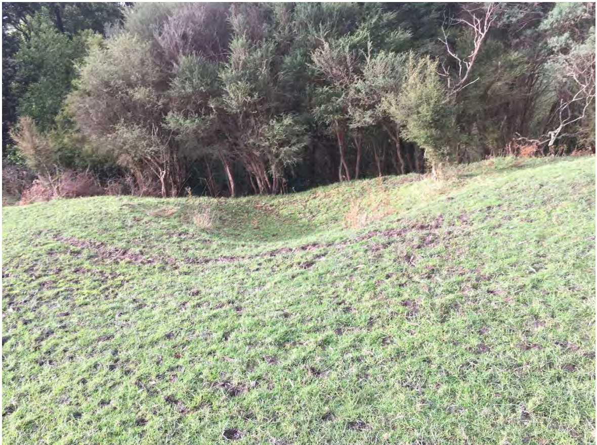
Small landslide feature, Hornes Road landslide edge, downslope from proposed Bushfire Shelter
