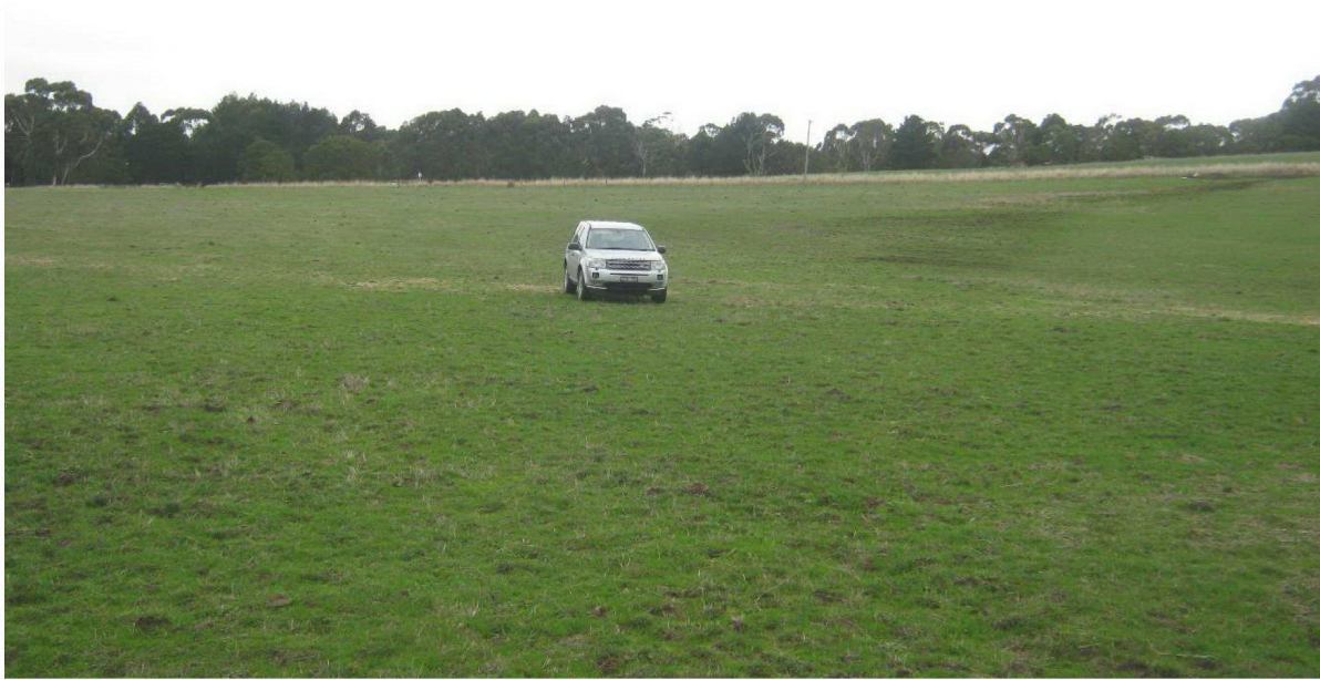
Dam looking east to Irrewillipe rd
