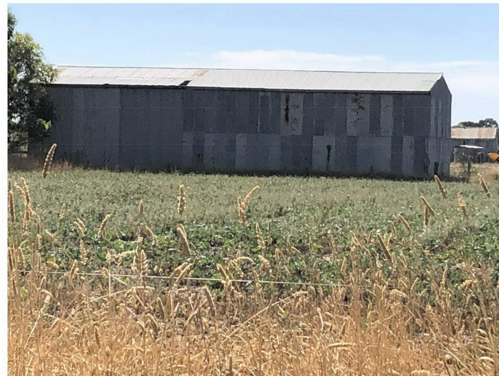
Existing Shed to be Converted to Processing Plant
