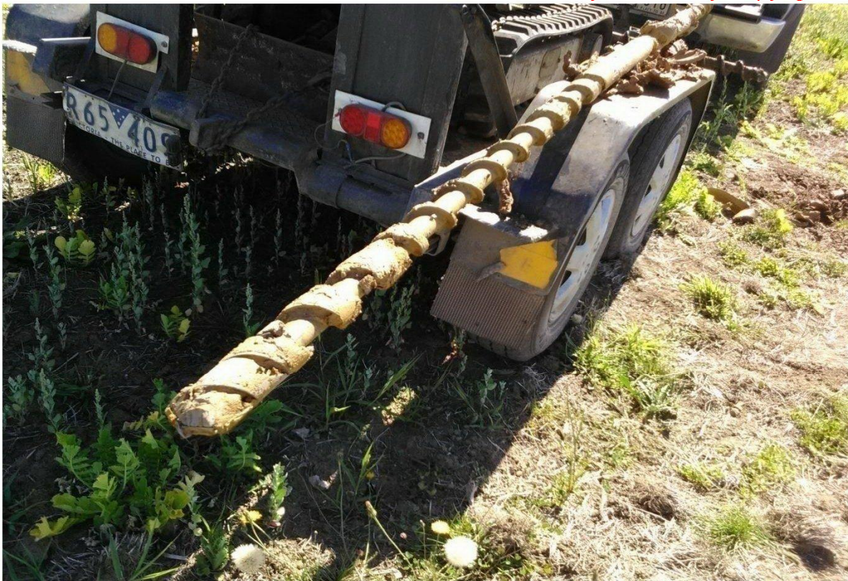
Fig 15. Soil profile investigation drilling proposed storage dam site. (Author).
