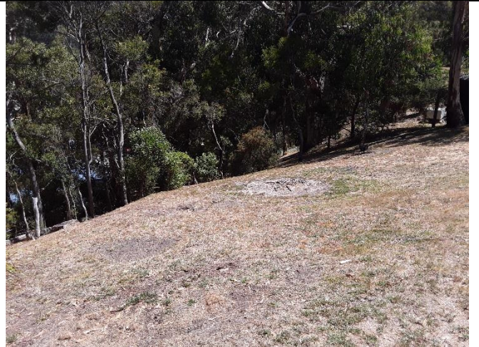
Photo 4: Landslide escarpment and steep break in slope.
