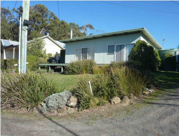
The above image shows the existing dwelling on the subject land with 31 McRae Road in the background.
