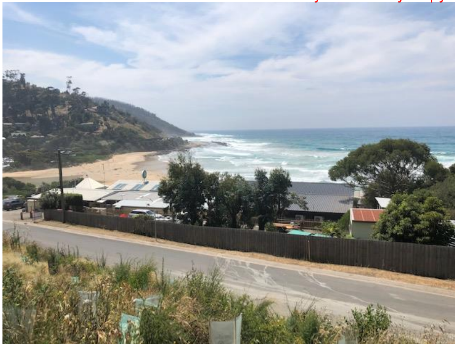
Figure 2 – Low threat vegetation around the Wye River Hotel to the south.
