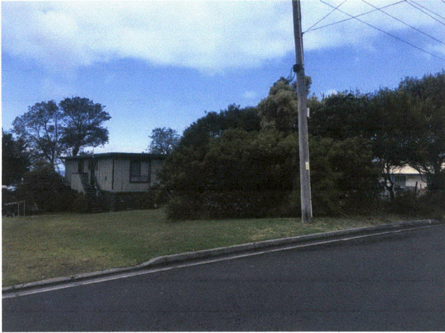
Photograph 3 View to northeast adjoining property from street
