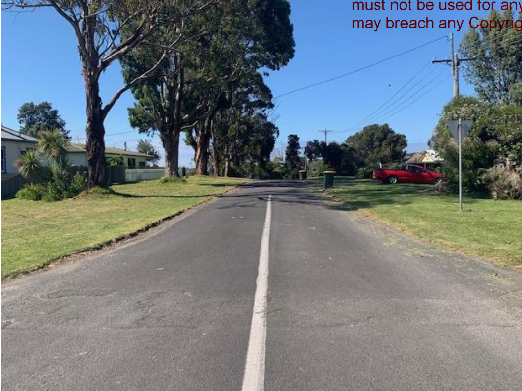
Photo 5 – Diana Street facing south.
