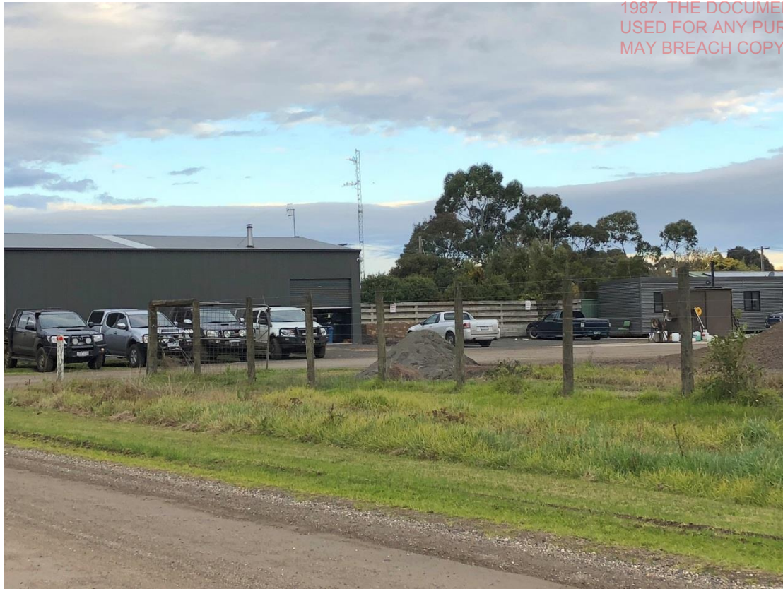
Figure 5: Existing sheds “store” accessed from Aireys Street.
