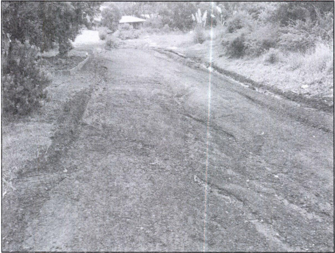
Ozone Street frontage, surface erosion following rain event (22.03.17)
