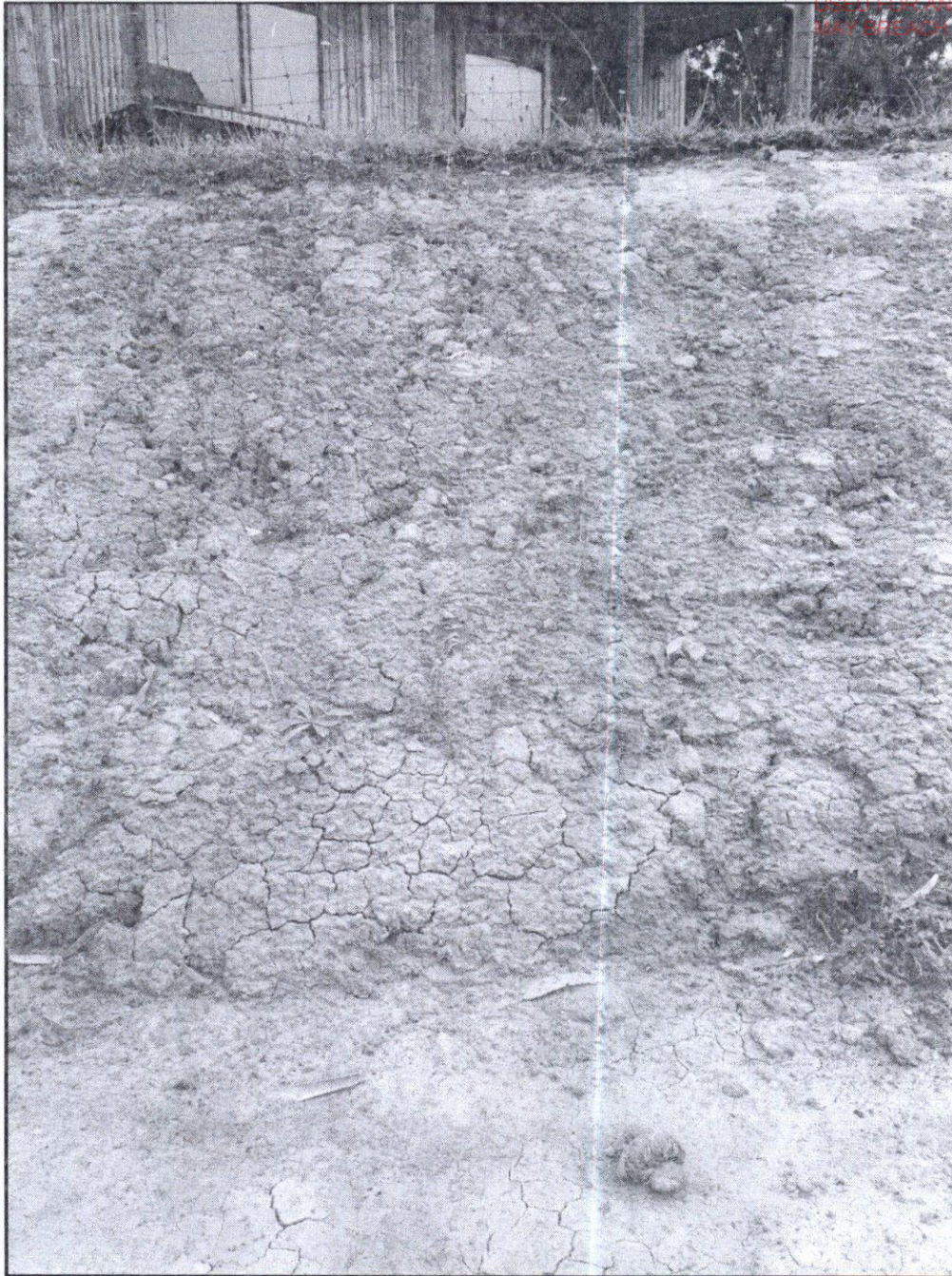
Existing site cut rear (north view)
