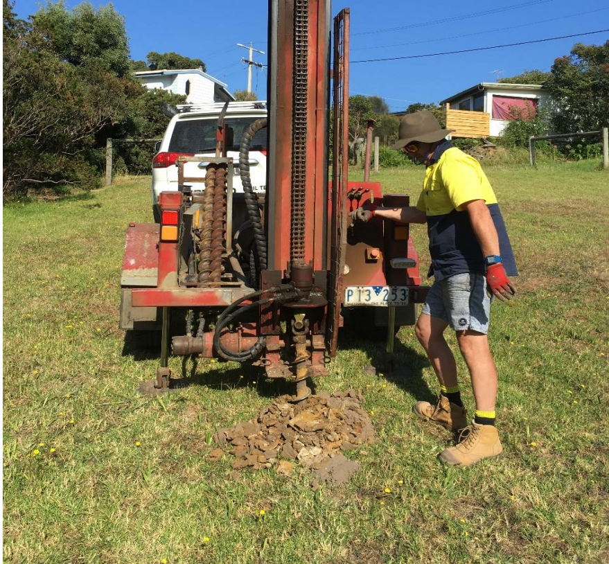
Photo 5: Borehole drilling being carried out.
