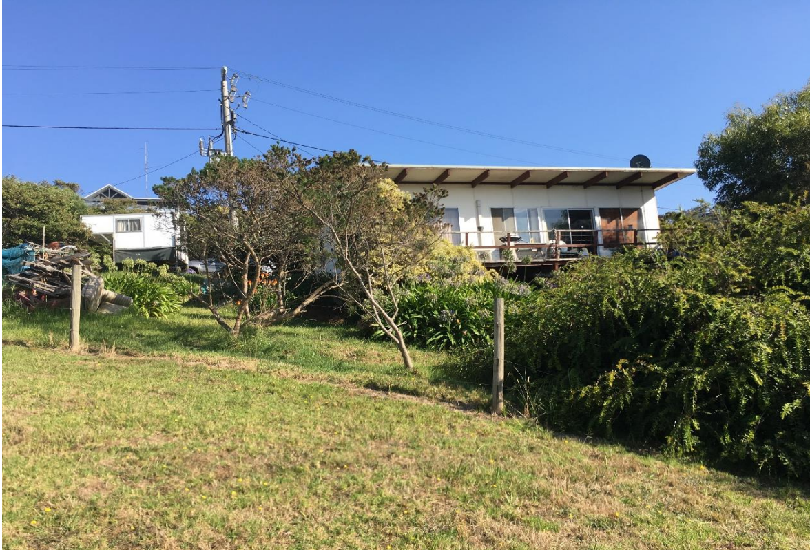
Photo 3: Existing site conditions, view north from borehole 2.
