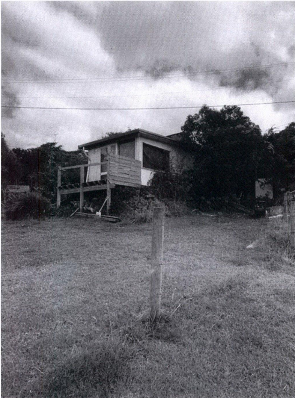
Photo 4: Existing fibro panelled shed adjoining the site to the rear at 30 Karlson Street.
