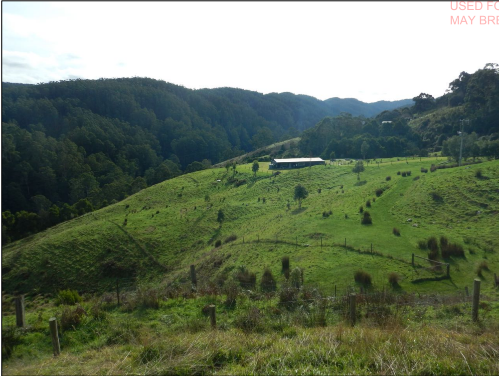
Figure 5 - Looking north at existing shed, showing orientation of proposed dwelling site in relation to the Forest to the west and north.
