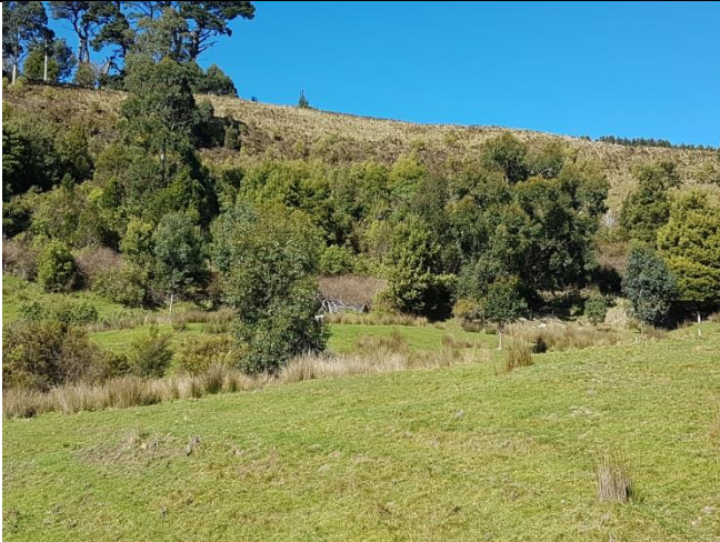
Photo 3: View of the slopes above the dam and the steep landslide scarp above Wild Dog Road
