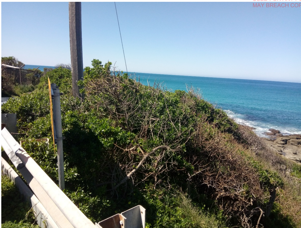
Figure 2. Adjacent slope to the south side of the compound.
