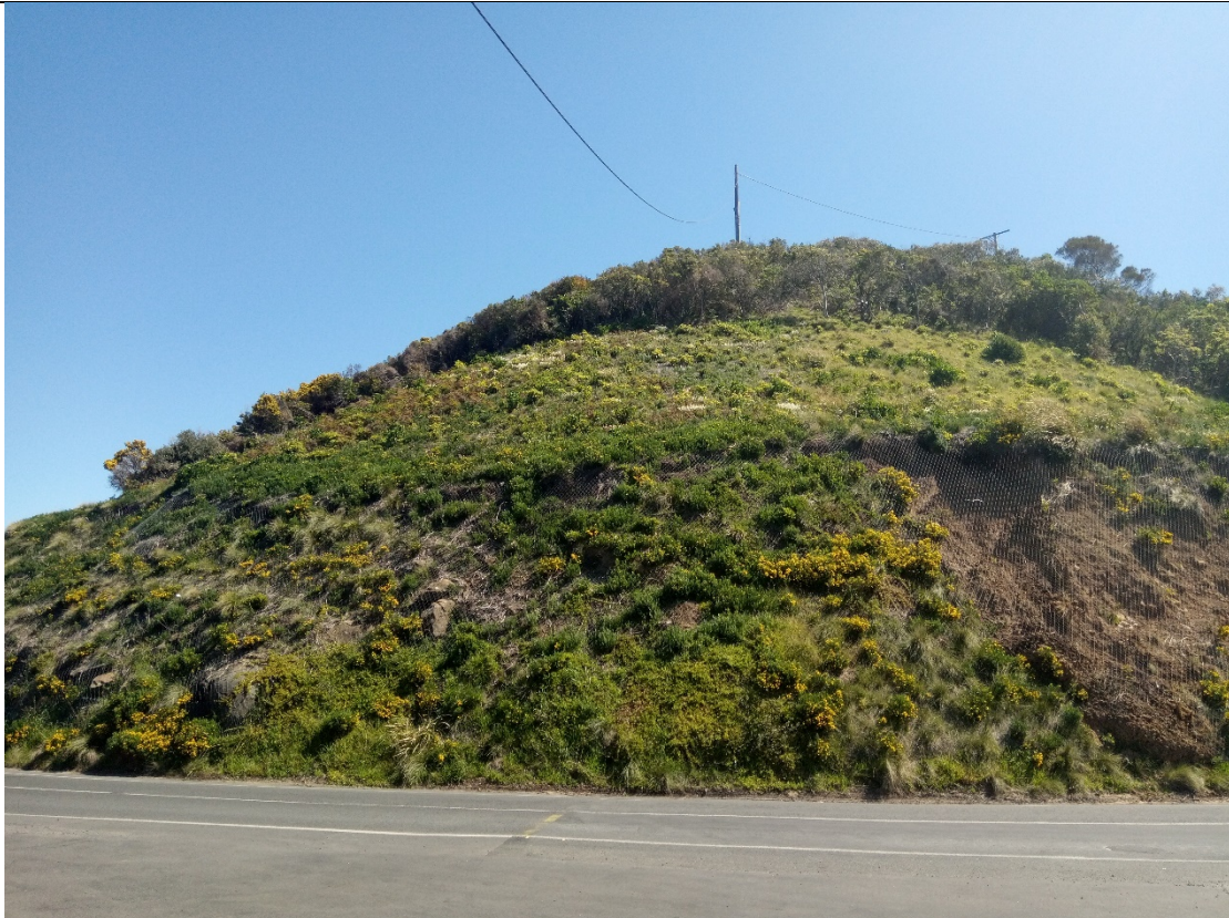
Photo 4: Slope to the west of the site, across the Great Ocean Road. Note geotechnical netting in place.
