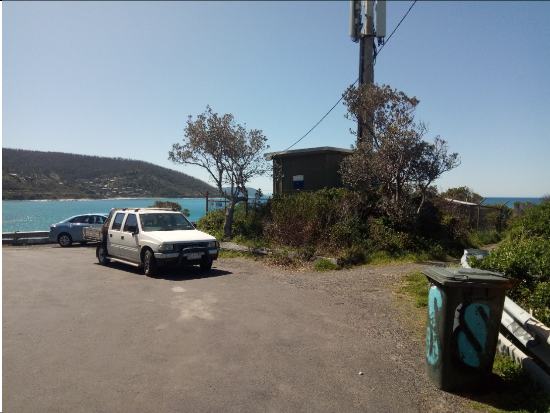
Photo 1: Looking north-east over the mobile network compound.
