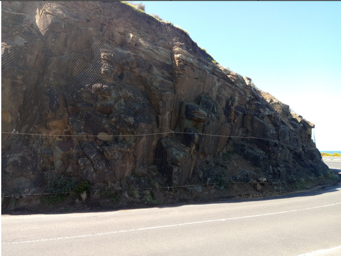
Photo 5: Extension of the geotechnical netting in Photo 4, south on the Great Ocean Road.
