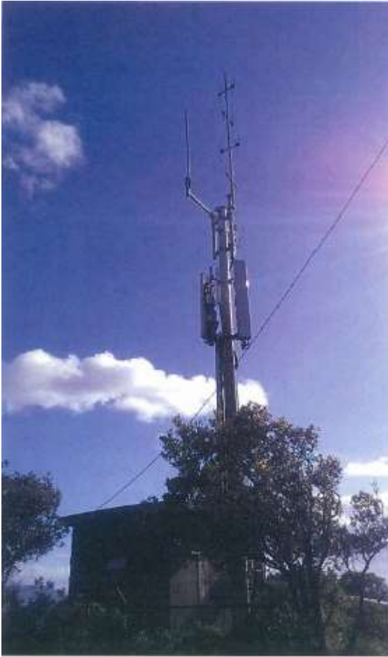
Figure 1 Existing telecommunications facility within the project area
