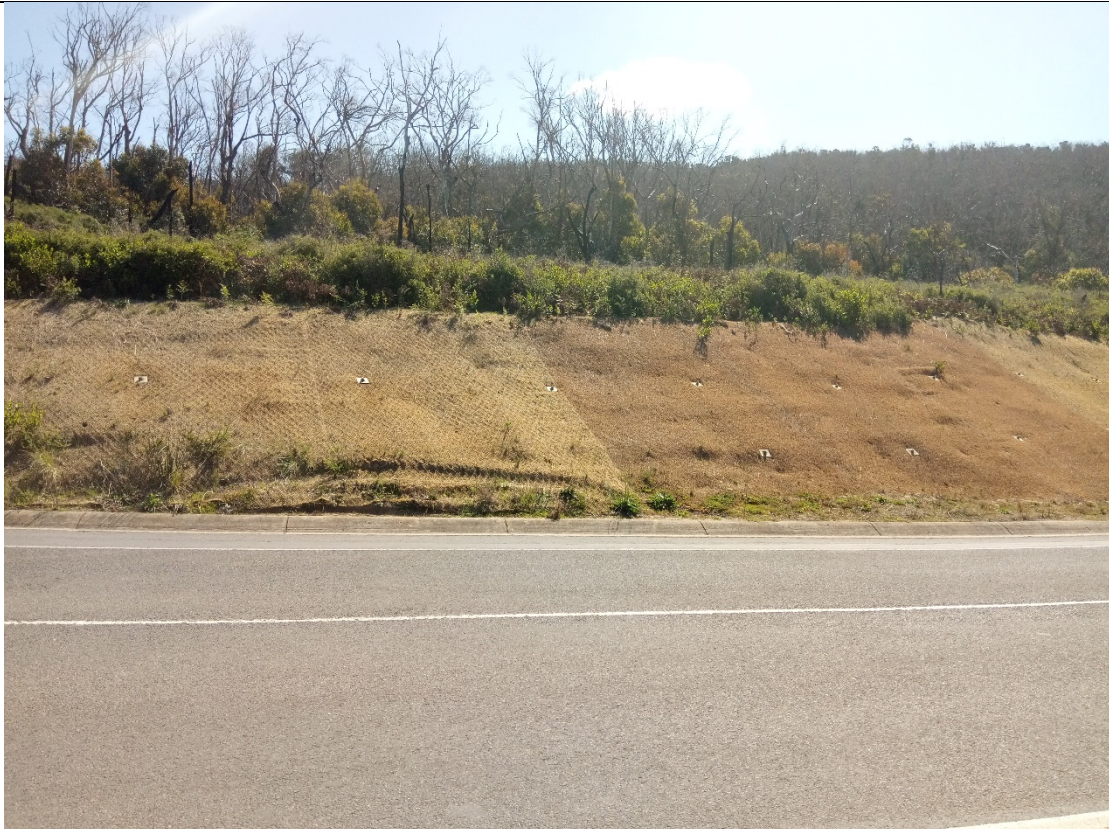
Photo 6: Geofabric placed on slopes around Wye River - north of the site.
