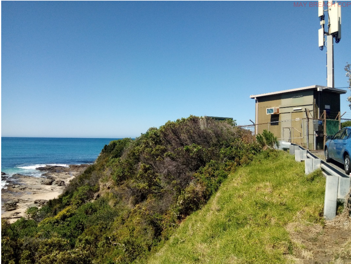
Figure 1. Adjacent slope to the north of the compound.
