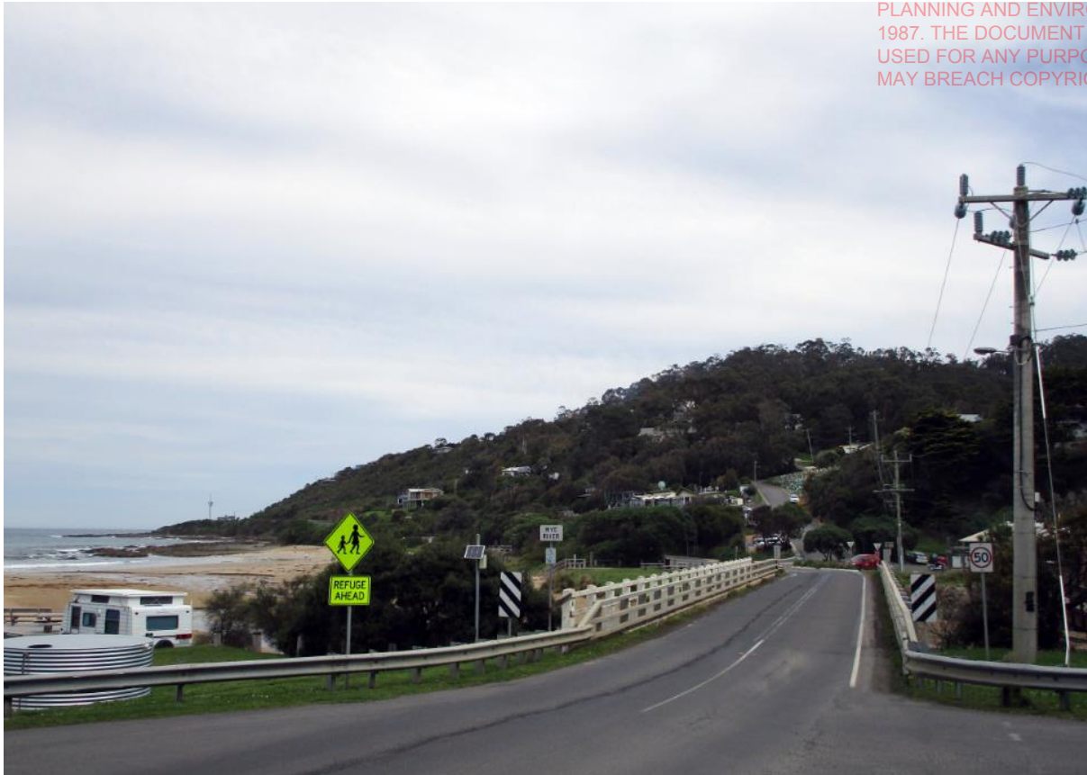
a) View from Wye River bridge looking south east towards the facility.
