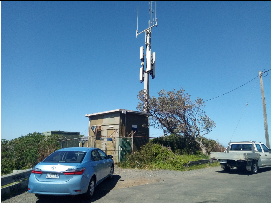
Photo 2: Looking south-east over the compound.
