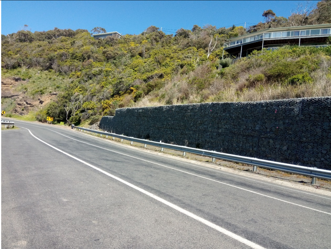
Photo 7: Gabion Walls placed in areas around Wye River – north of the site.
