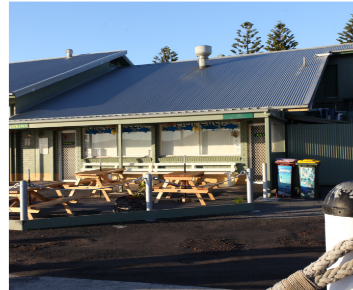
Image 18. Existing Fish Co-Op Building with Norfolk Island Pines in the background
