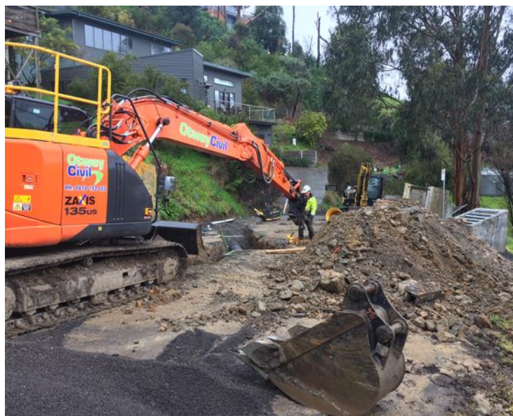
Laying of pits and pipes at Wallace Street
