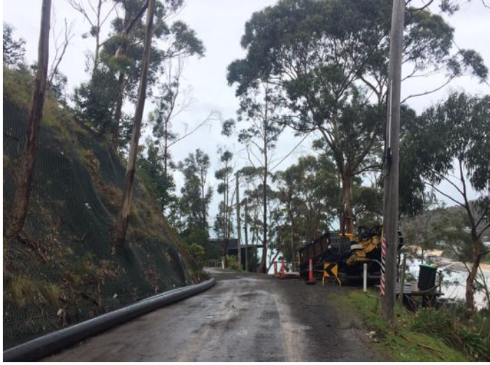
Durimbil Avenue - welded pipe and boring machine
