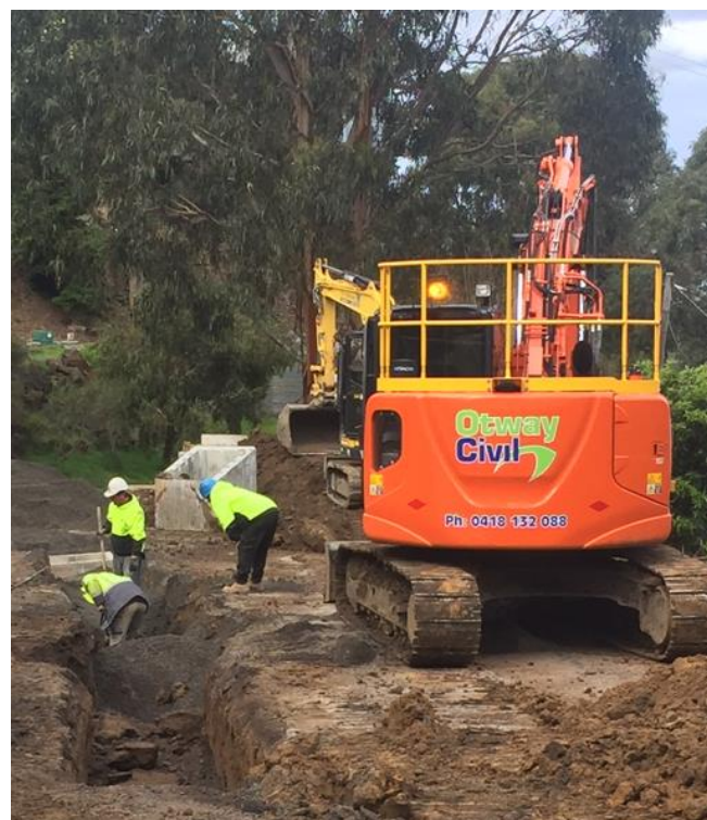
Laying of pits and pipes at Wallace Street
