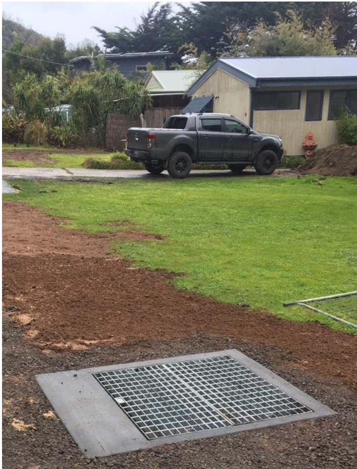
Completed pit arrangement in Sarsfield St
