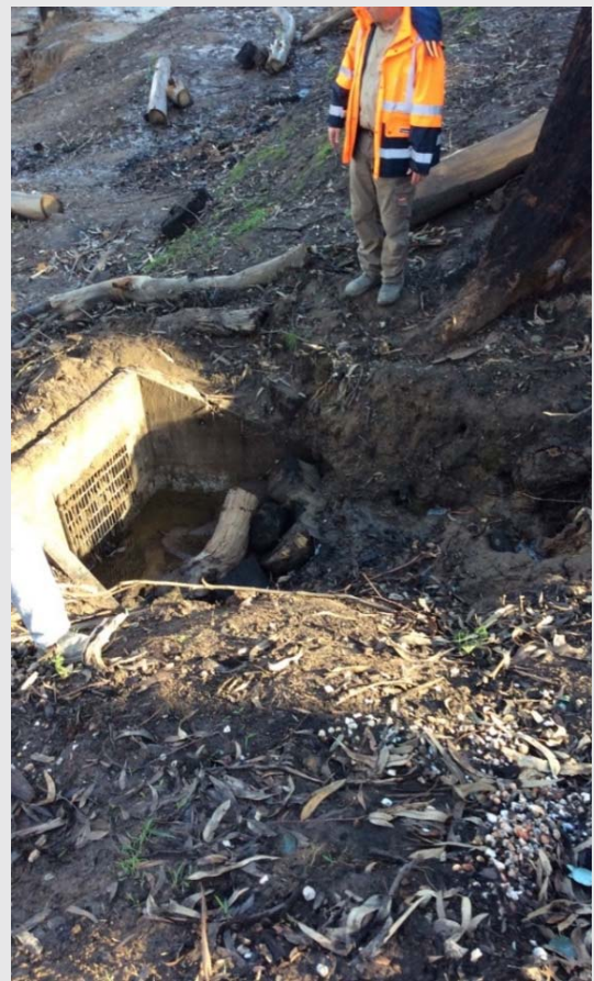
Figure 39 15 Koonya Ave Culvert Inlet
