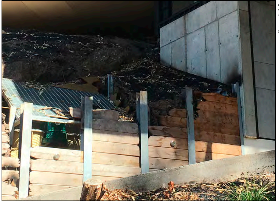
Plate 4 Damaged retaining wall at a Wye River property
