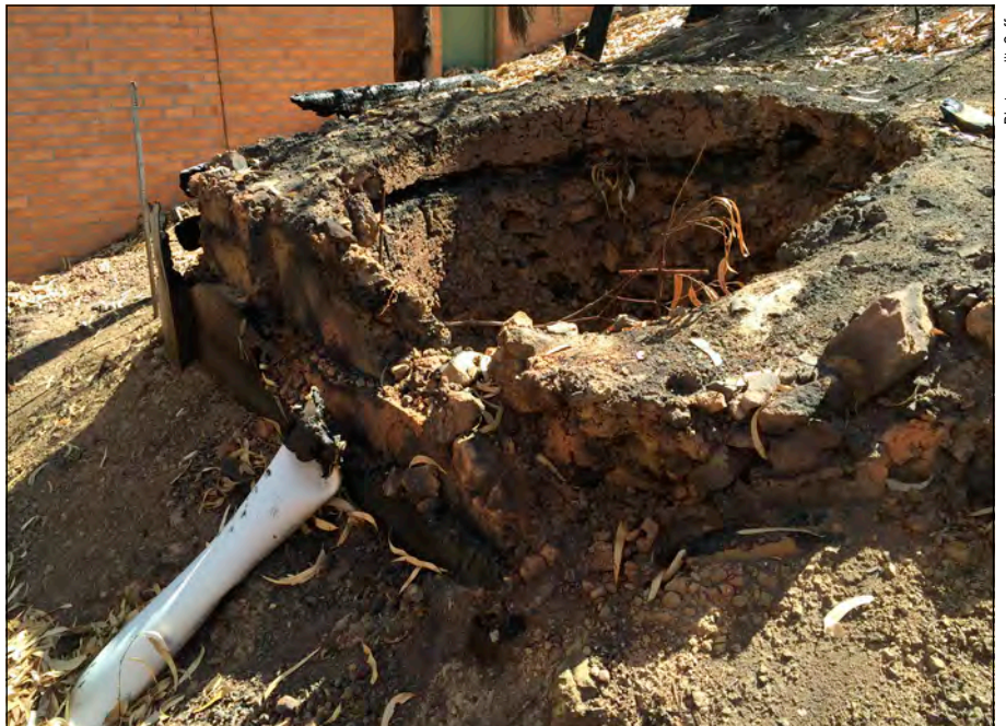
Plate 6 Remaining hole where a water tank was destroyed
