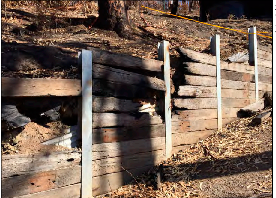
Plate 5 Burnt retaining wall at a Wye River property
