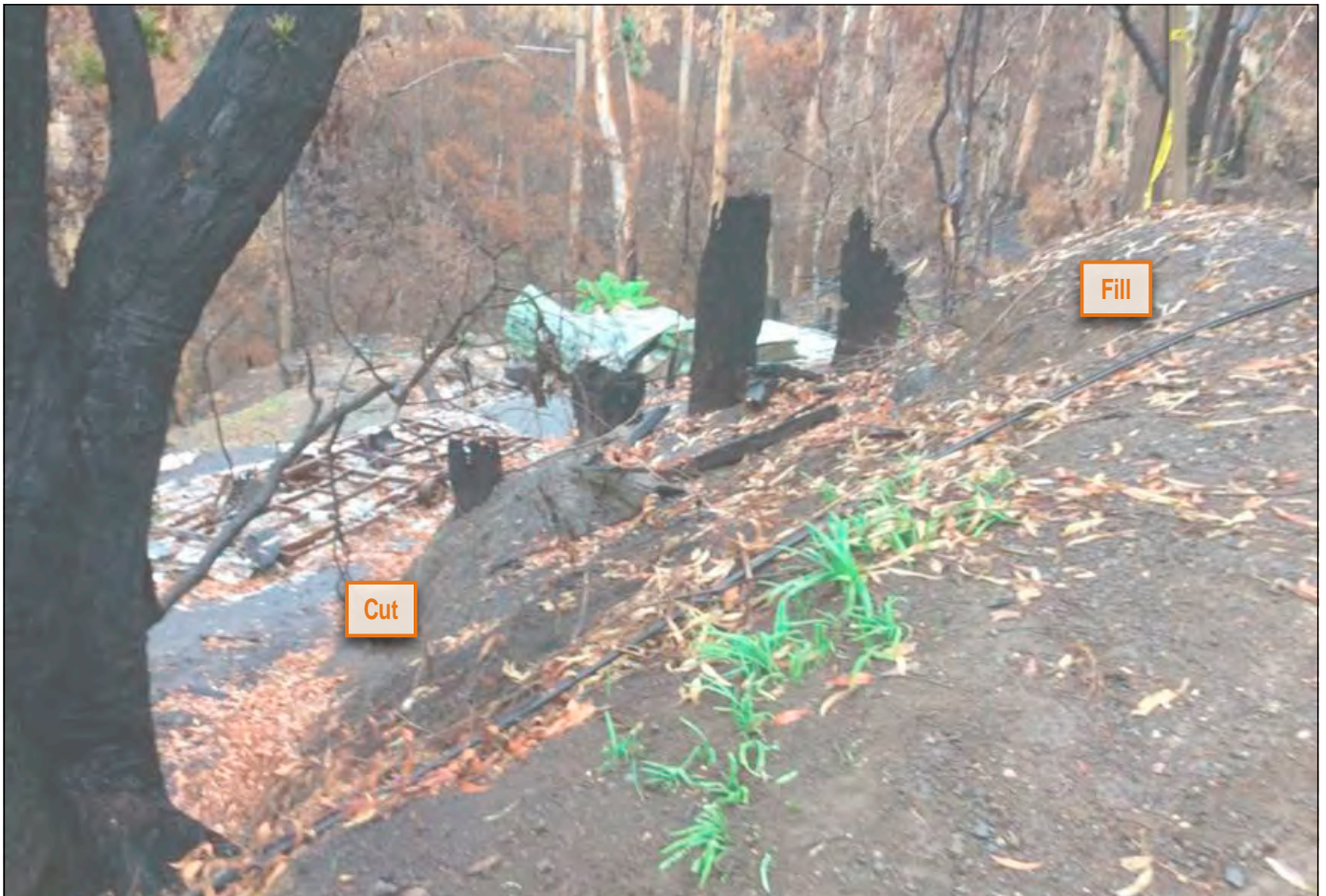
Photograph 4 "Downslope" property showing both cut and fill
