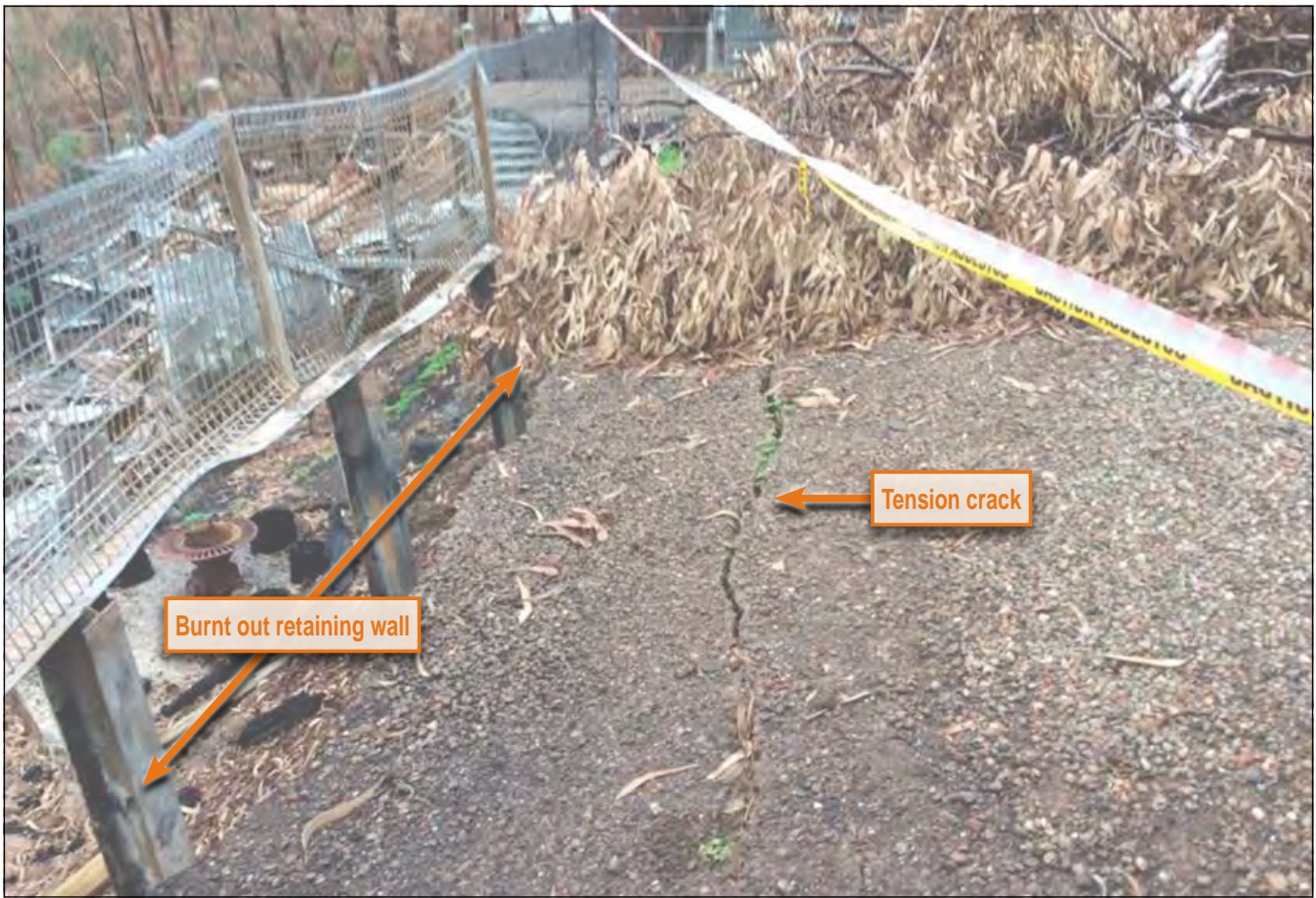
Photograph 1 Tension crack in carport adjacent to burnt out retaining wall
