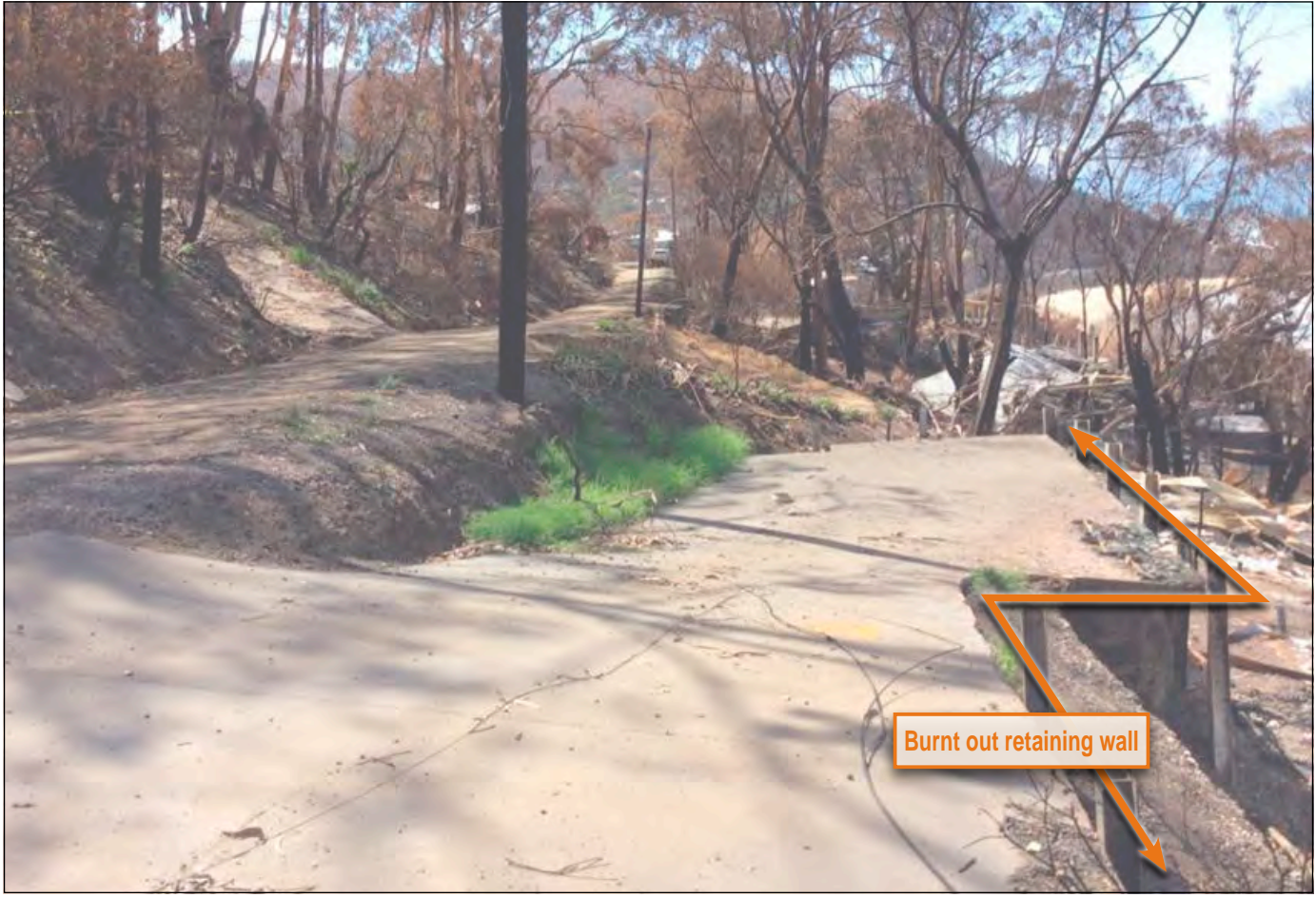
Photograph 2 Burnt out retaining wall
