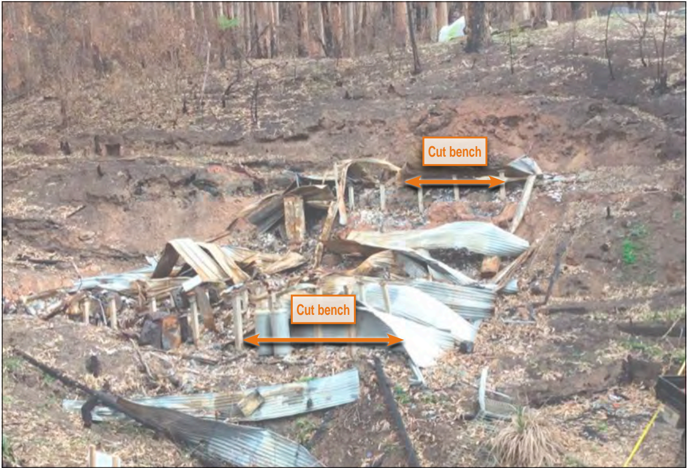
Photograph 3 "Upslope" property showing cut benches
