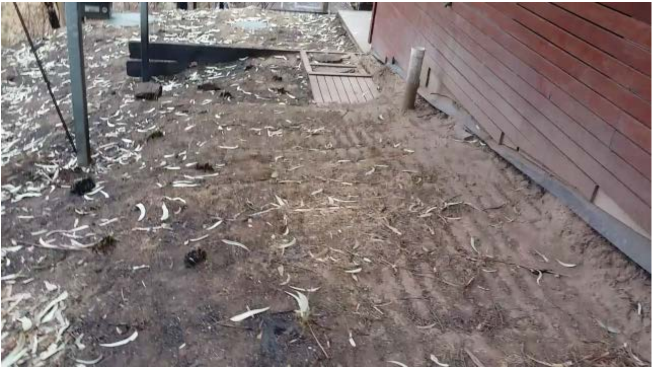
Figure 71: 33 Bare earth interface adjacent to sub-floor area. The dried earth on the sub-floor boards indicate water suppression in the area.
