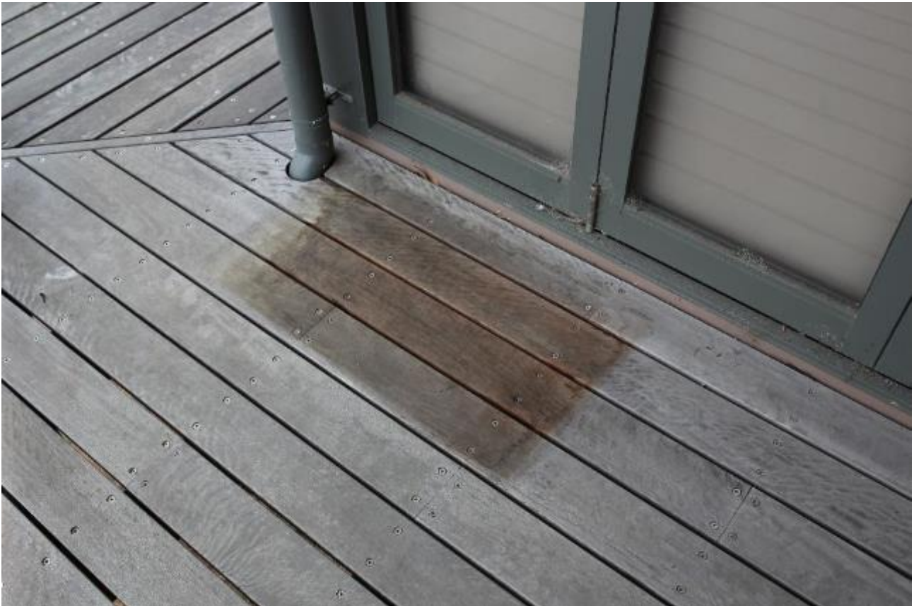
Figure 32: An example of the removal of a doormat from a deck.
