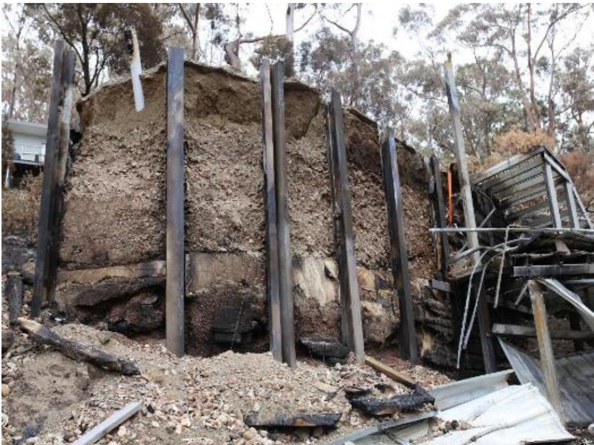
Figure 30: Driveway off Karingal Drive, Wye River. An example of burnt out timber retaining wall sleepers.
