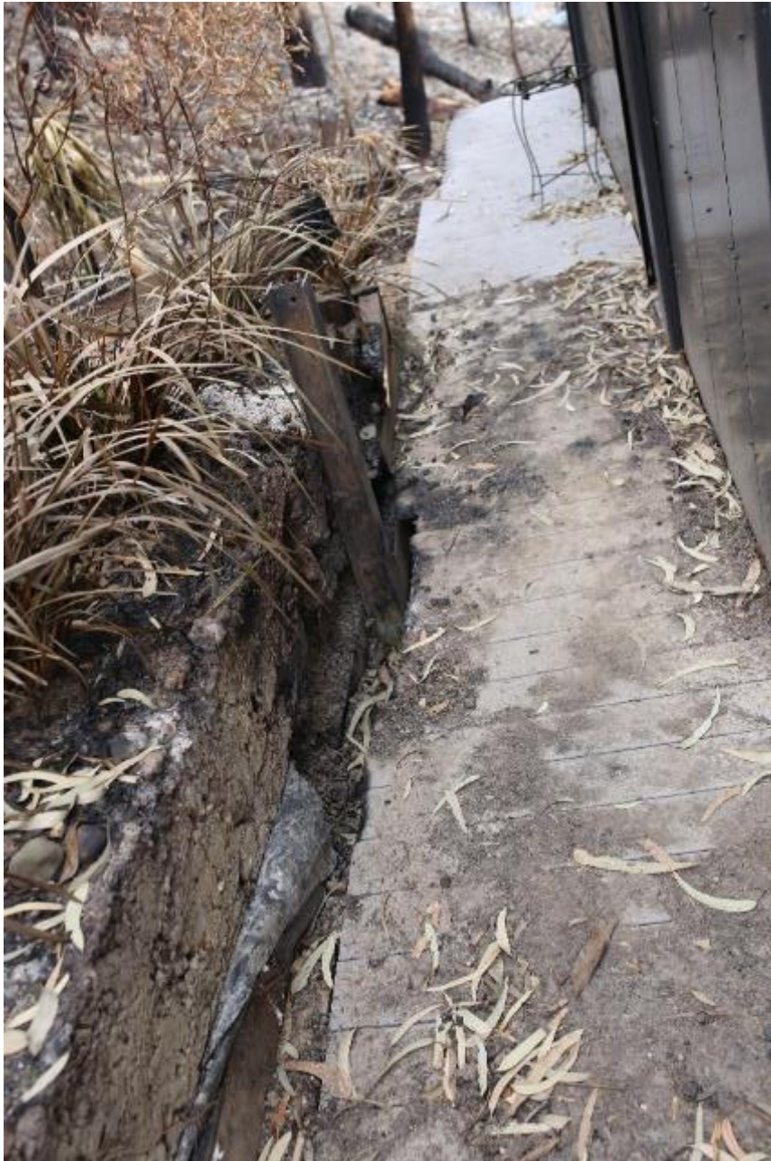
Figure 39: Deck-retaining wall interaction with evidence of water wash from aerial suppression.
