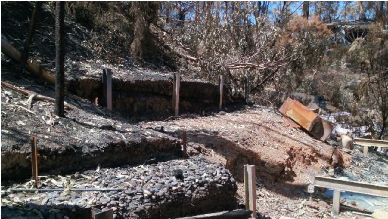
Figure 50: Burnt retaining walls adjacent to house.
