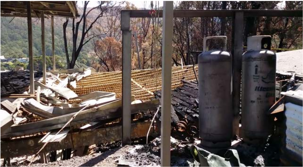
Figure 61: Rear deck combustion at driveway entrance
