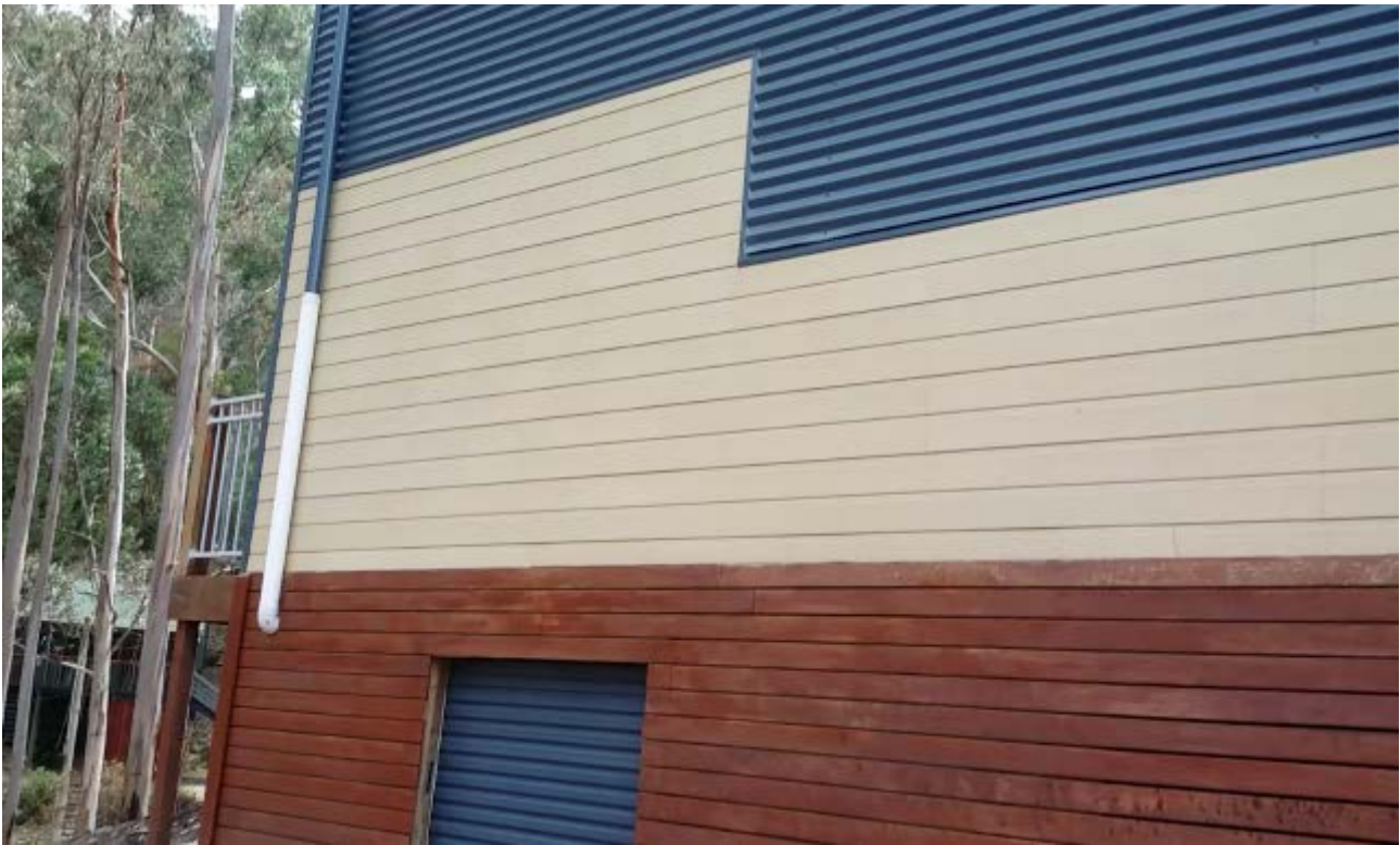
Figure 65: Cladding of walls and sub-floor
