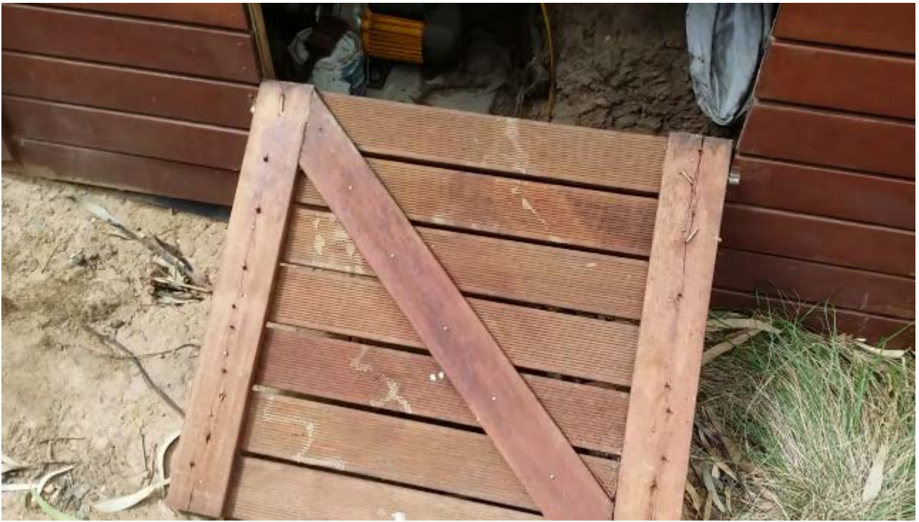
Figure 67: Subfloor area and material stored within.
