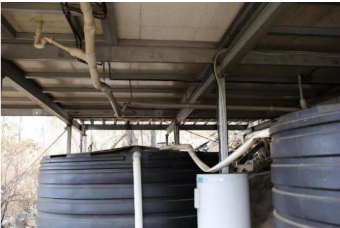
Figure 41: Water tanks and piping in subfloor area.
