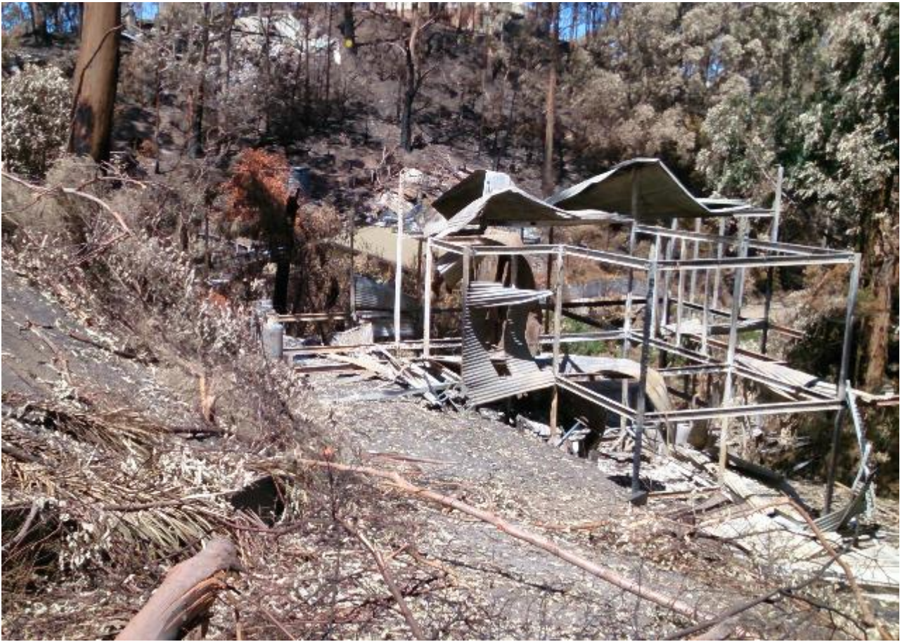
Figure 52: House on Durimbil Avenue showing house and location of pressure vessels.
