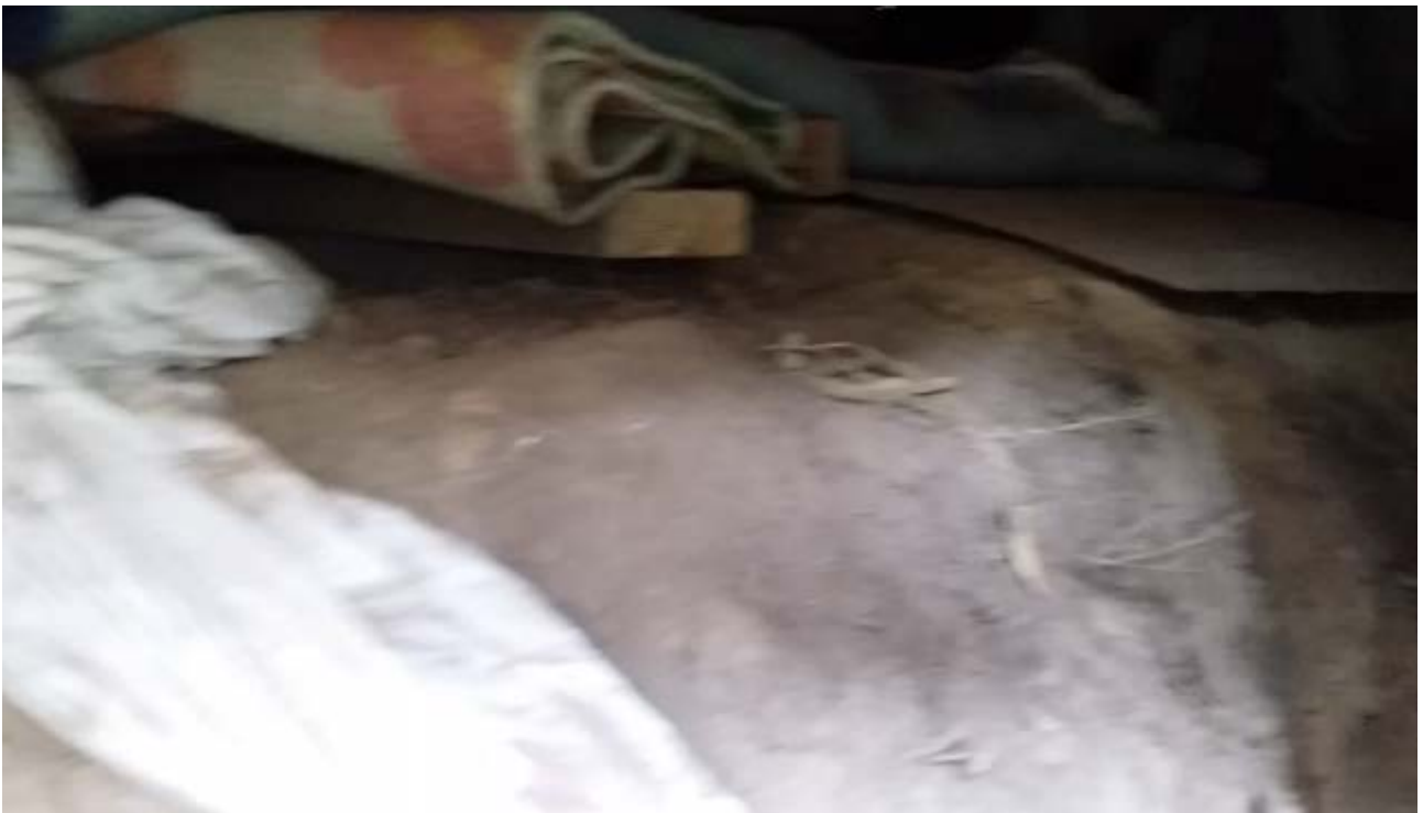
Figure 68: Extensive combustible objects in sub-floor area
