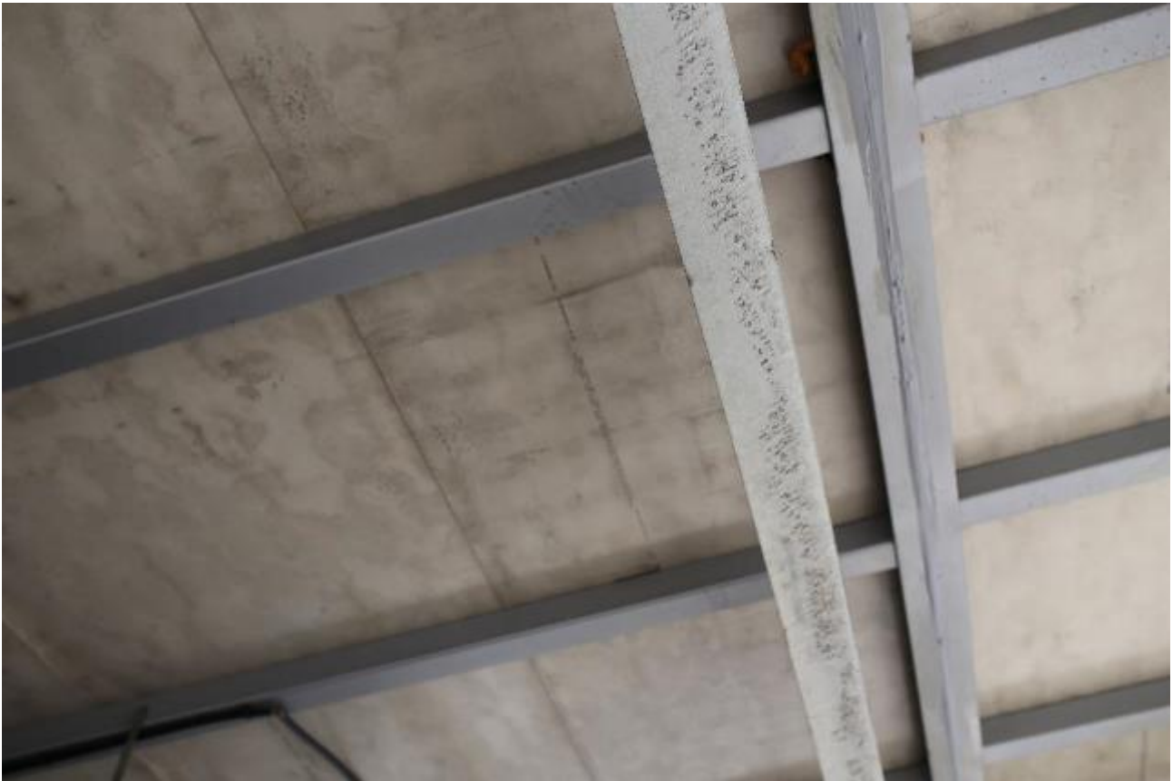
Figure 36: Under floor system, steel and James Hardie Scyon flooring.
