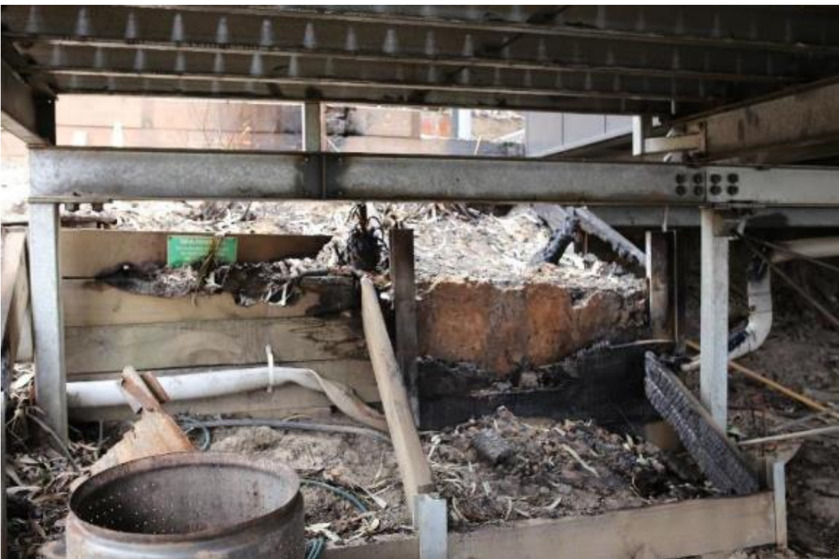
Figure 38: Retaining wall combustion below the deck.
