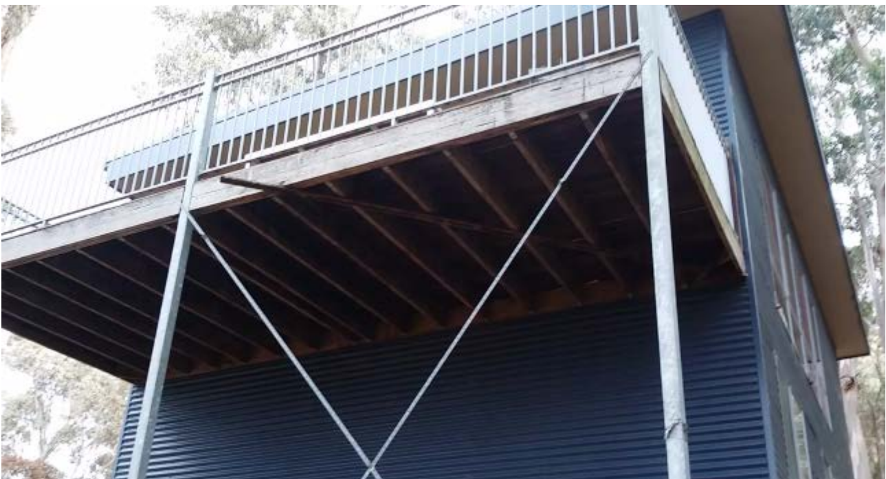
Figure 72: 33 Elevated deck with no clear signs of radiation or ember attack.
