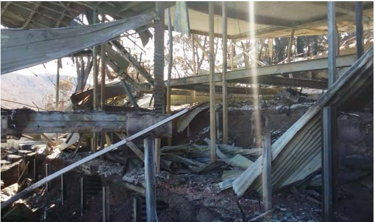
Figure 59: 23 Location of burnt out timber retaining walls below and beside structure
