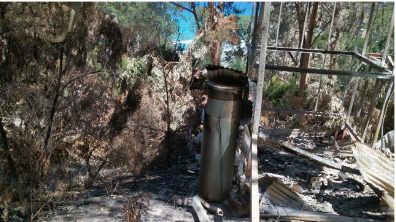
Figure 49: House on Durimbil Avenue showing adjacent vegetation scorch.
