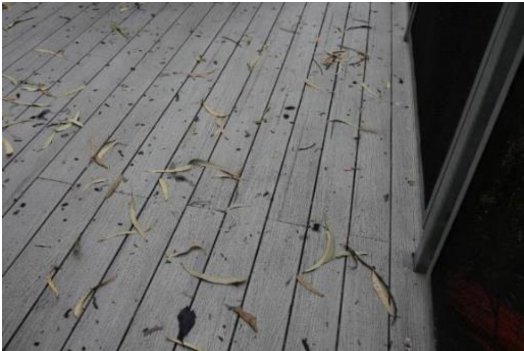
Figure 42: Ember scorch marks on plastic-wood composite decking.
