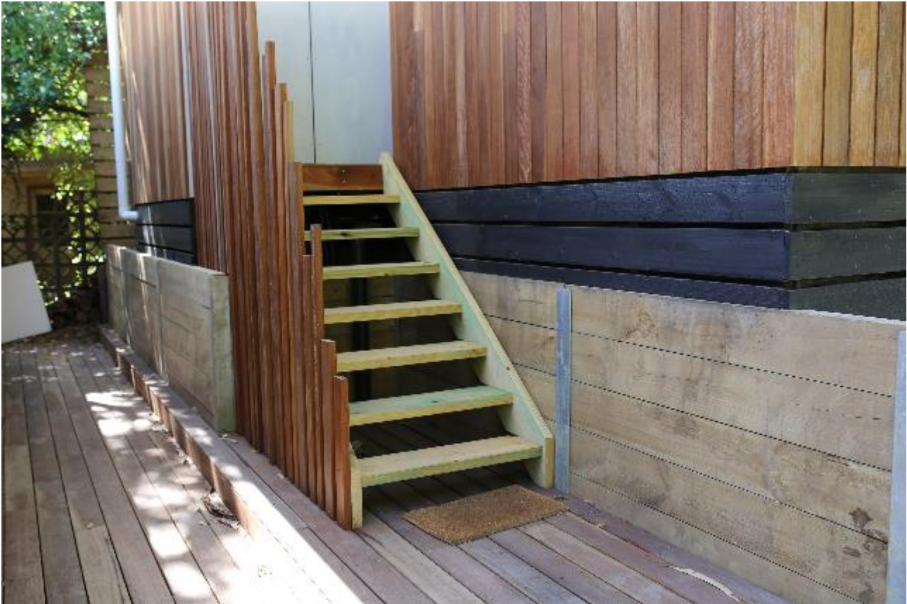
Figure 4: Example of land stabilisation using timber sleepers in proximity to other combustible features within Wye River.
