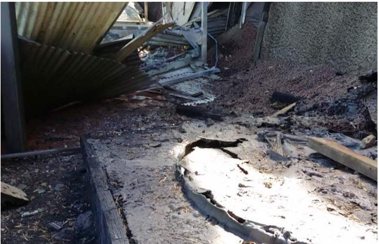
Figure 60: 23 Burnt out retaining walls and tank adjacent to house.
