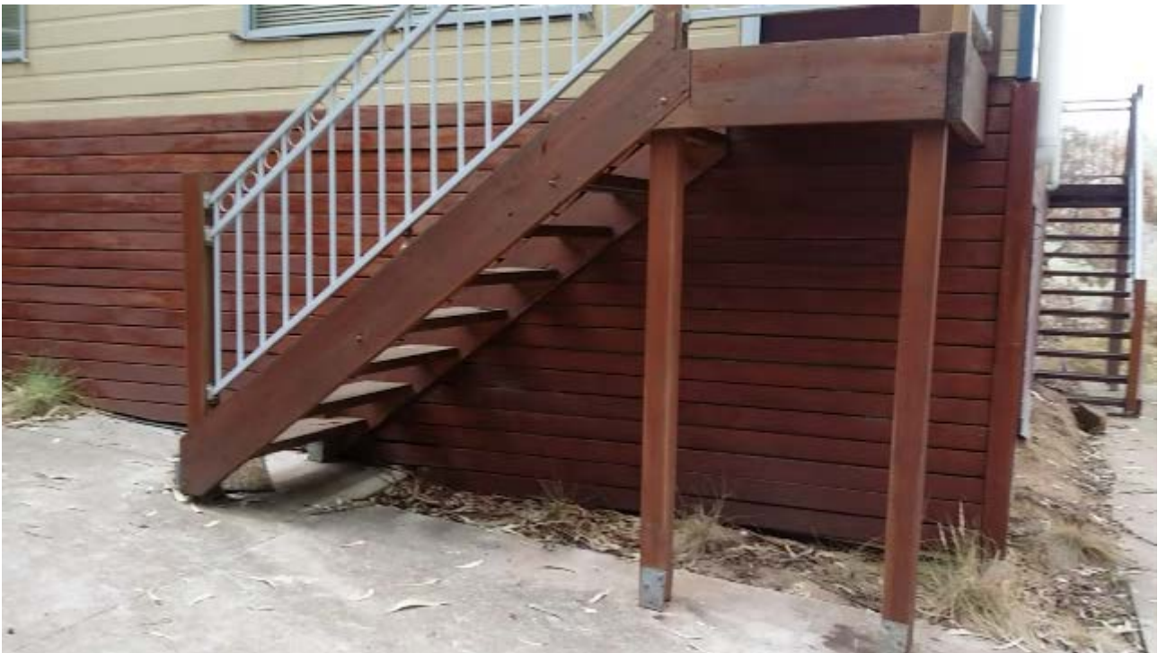
Figure 66: Concrete apron, house to surface fuel orientation, and surface fuels present after the fire.
