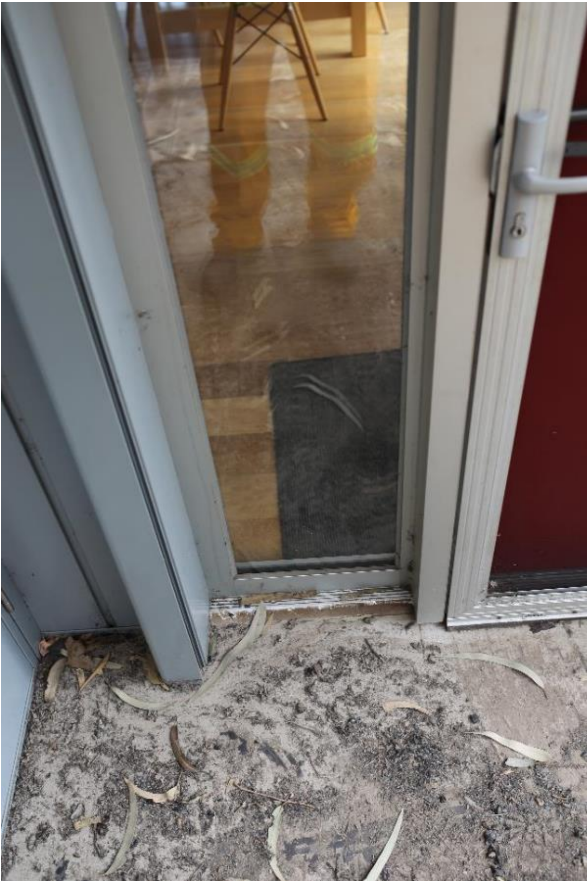
Figure 33: Silt washed onto decking from an adjacent water drop
