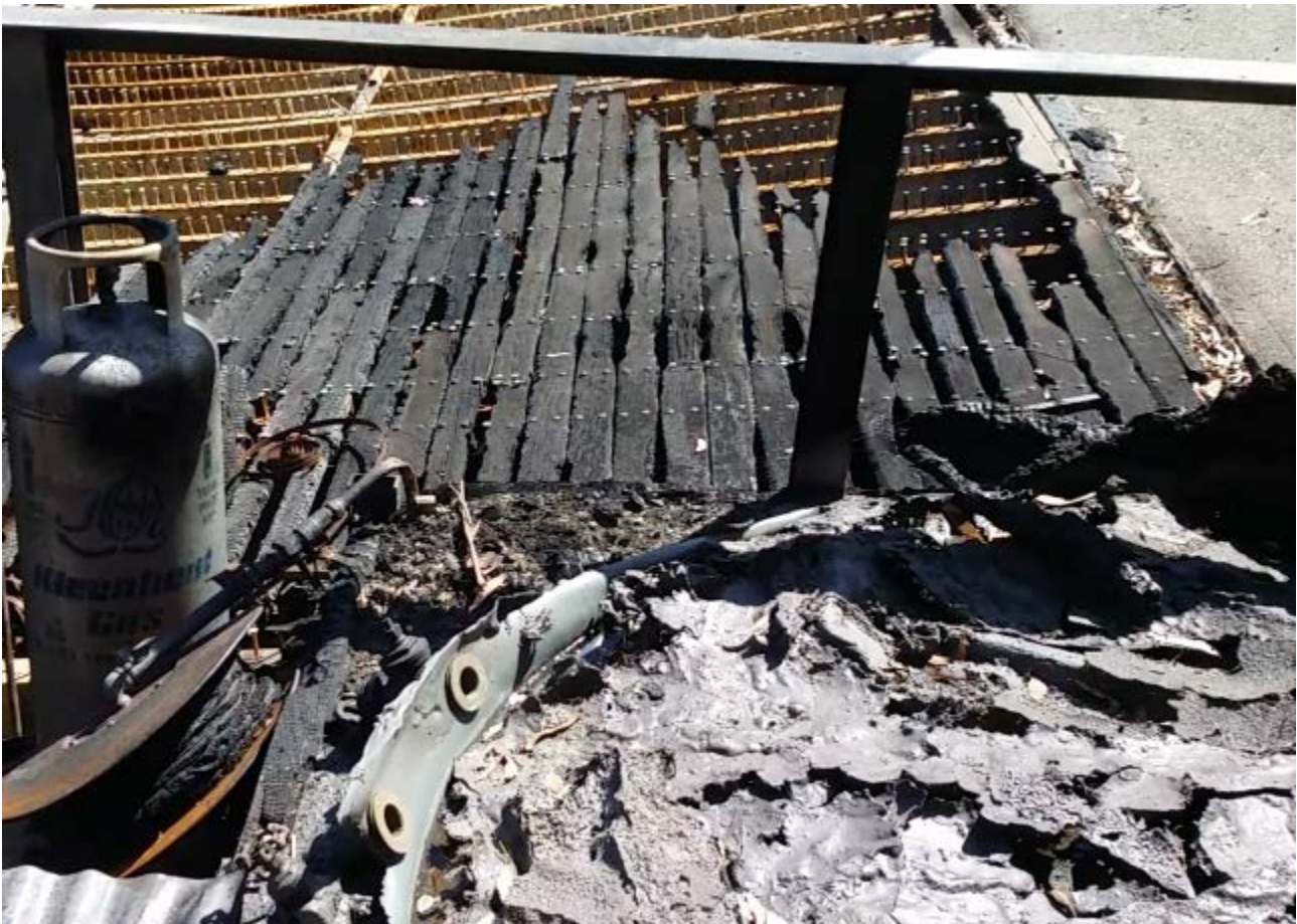
Figure 62: 23 Interaction between the timber driveway deck and a polyethylene water tank. It is possible that the ruptured water tank split out over the timber driveway and prevent the complete combustion of the deck.
