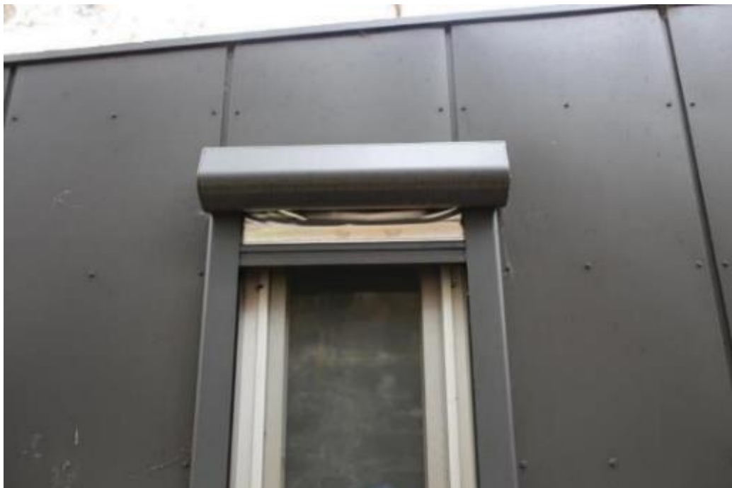
Figure 43: Window with pull down fire shutter.
