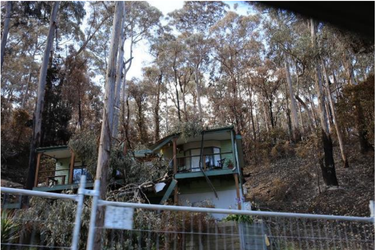
Figure 31: A house on Wallace St Wye River, subject to tree strike cause by fire interaction at the base of a tree.
