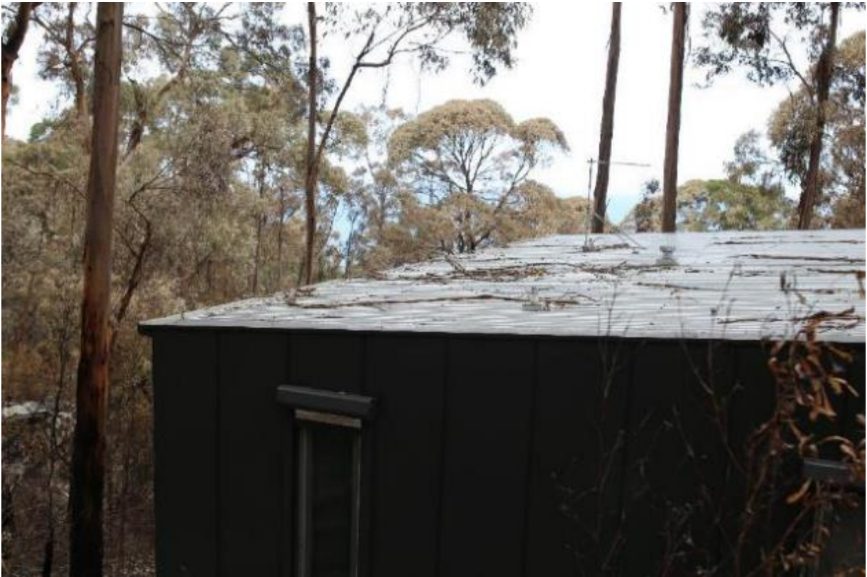
Figure 44: Simple roof profile with metal gutter guards.
