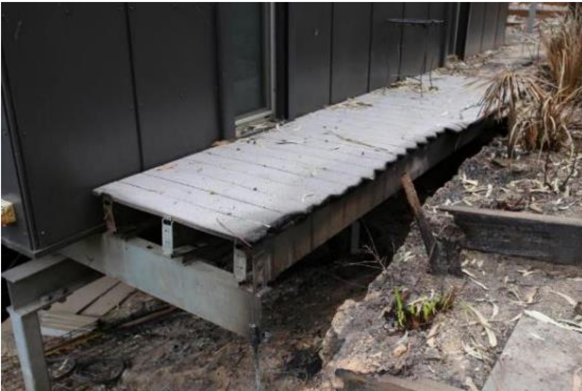
Figure 40: Impacted decking and support structure.
