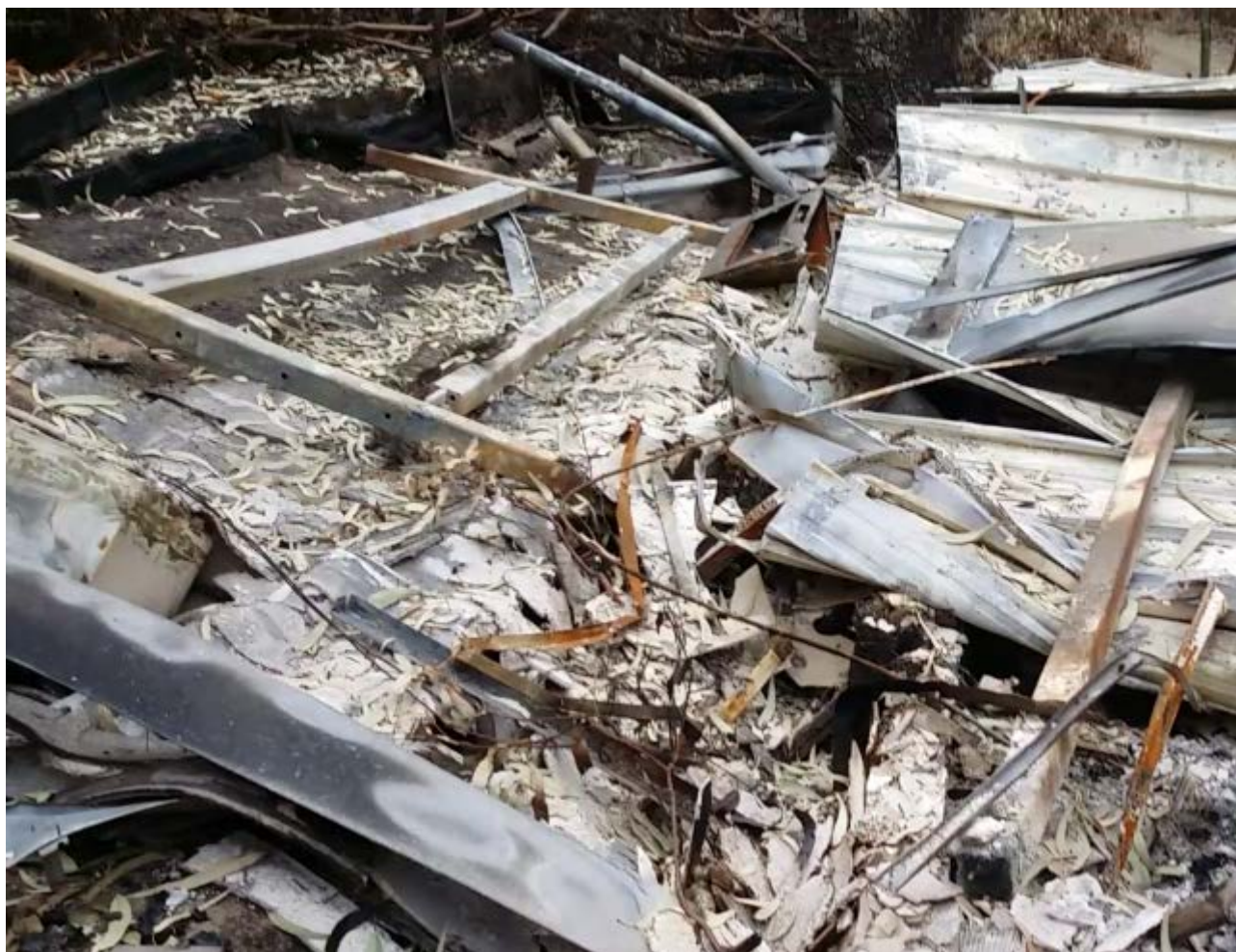
Figure 56: Ground to wall interface after the fire.
