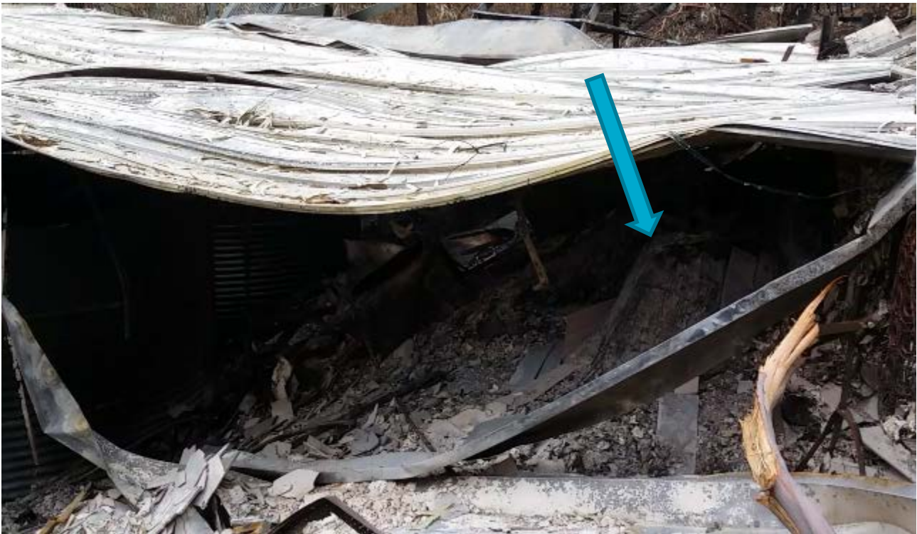
Figure 54: House on Koonya Avenue showing an old tree stump under the floor on the right of the picture.
