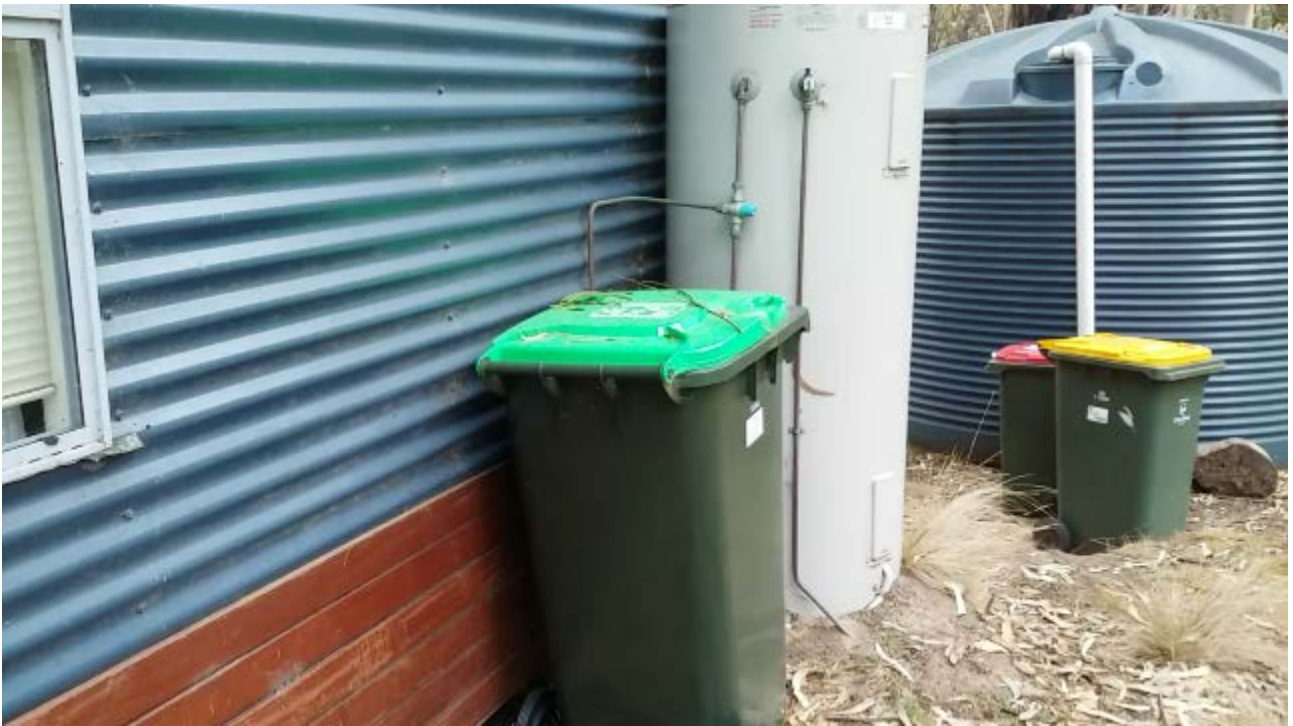
Figure 69: House to tank proximity and adjacent combustible elements including rubbish bins and firewood.
