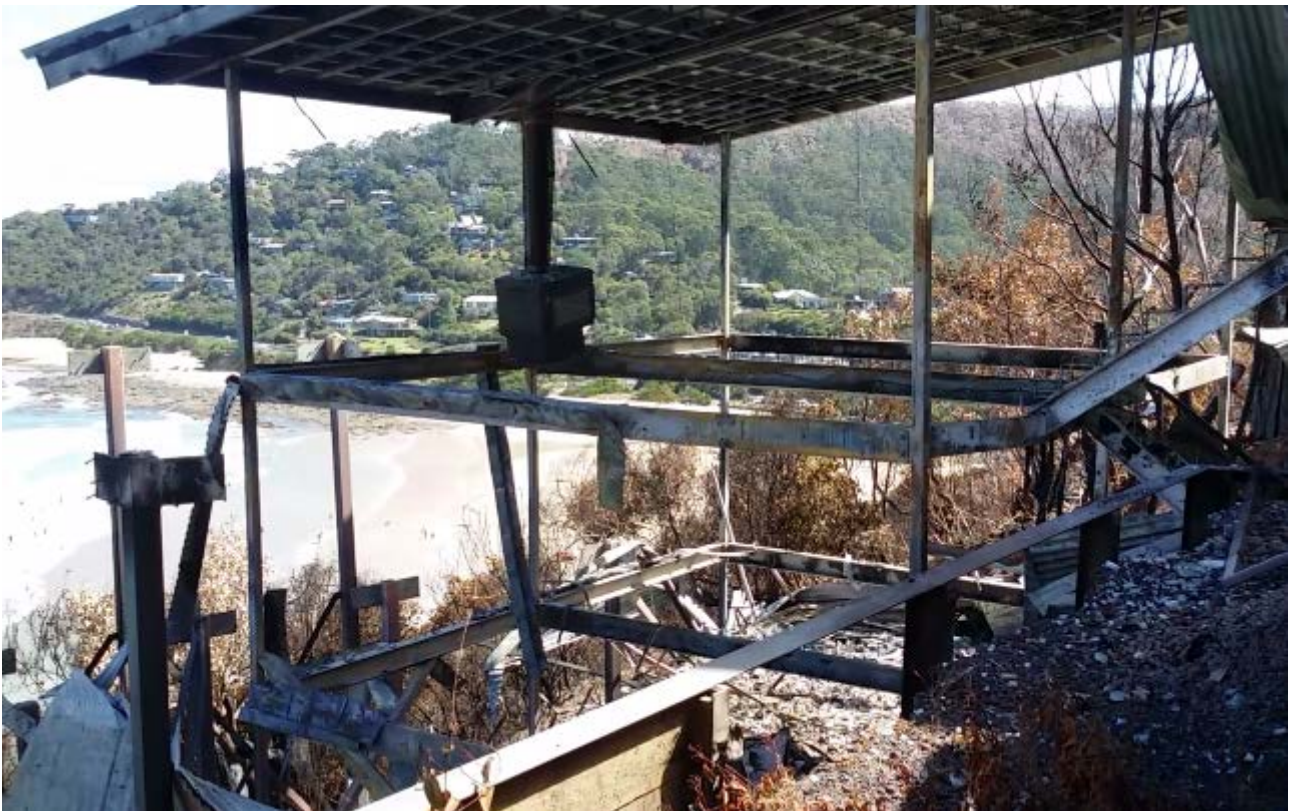
Figure 58: House on Iluka Avenue Wye River, showing vegetation condition below structure
