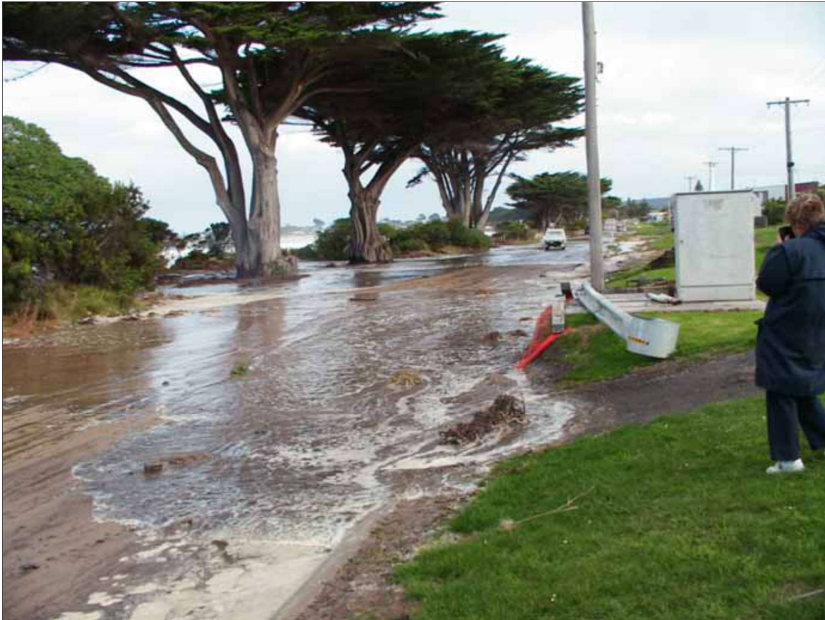
FIGURE 5-2 COASTAL INUNDATION IMPACTING THE GREAT OCEAN ROAD IN APOLLO BAY (G. MC PIKE 2005)
